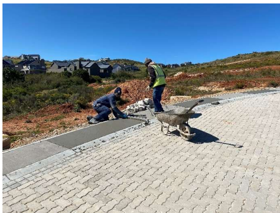
Road verges being constructed within Phase 9.
