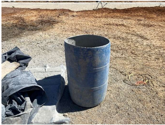
Dustbins present on site at each cement batching area for discarding the ready-mix bags.
