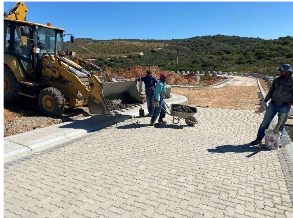
Cement being transported with TLB and loaded into a wheelbarrow for road verges within Phase 9.
