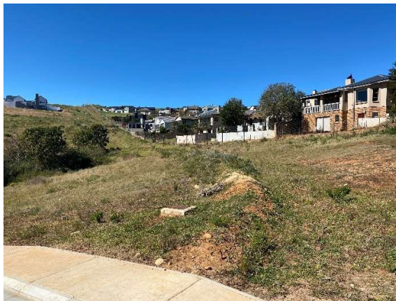
Detention Swale within Phase 10.
