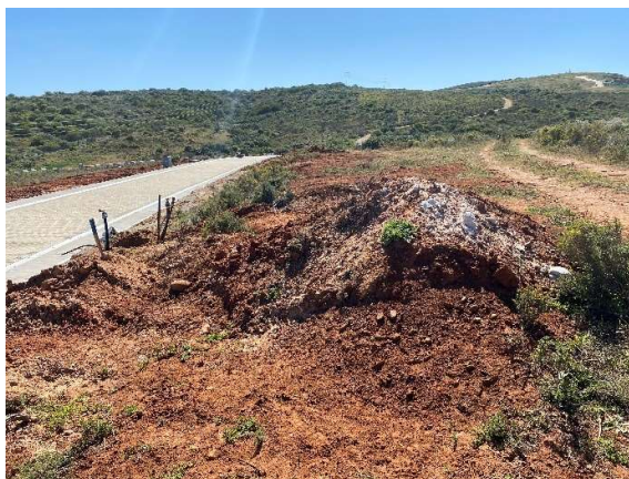
Topsoil windrowed and utilised along the road verges within Phase 9.
