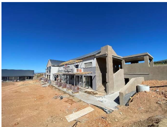
The school building under construction.
