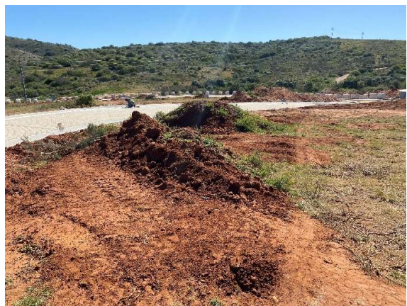
Topsoil windrowed and utilised along the road verges within Phase 9.
