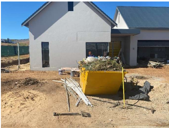
Skip present at a construction site within Phase 10.
