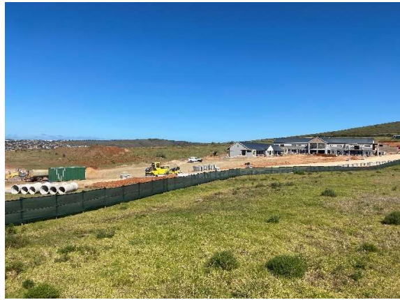
Condition of construction within Phase 19 appropriately screened/fenced off with shade netting.
