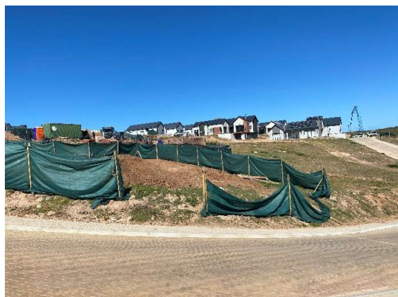
Each residential construction site has been screened with shade netting.
