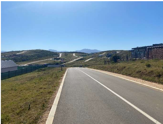
Condition of access road leading toward Phase 10.
