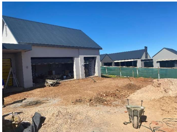
Condition of a residence being constructed in Phase 10.
