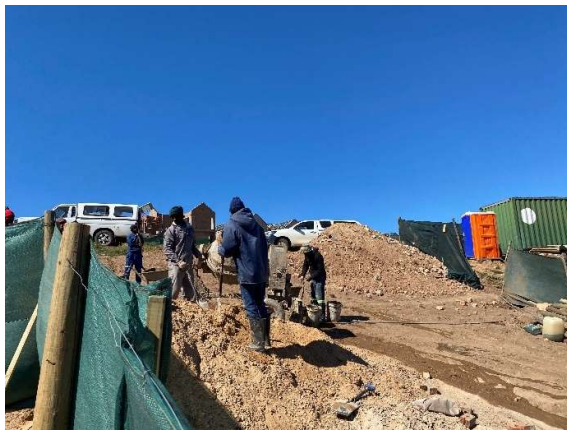
Active cement batching within a single residence in Phase 4.
