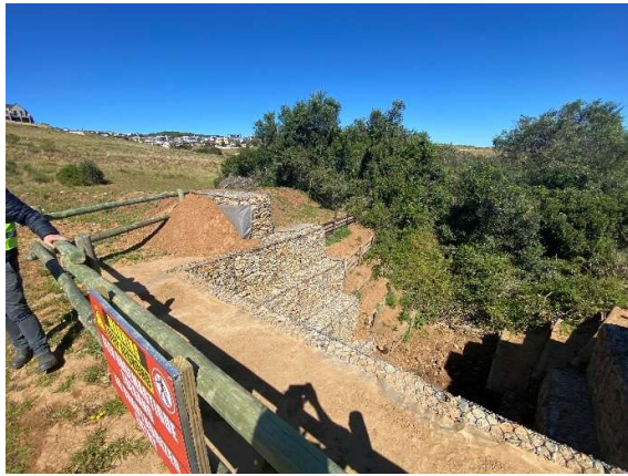
Large gabion stormwater culvert discharge infrastructure area for stormwater from Phases 11 - 14.
