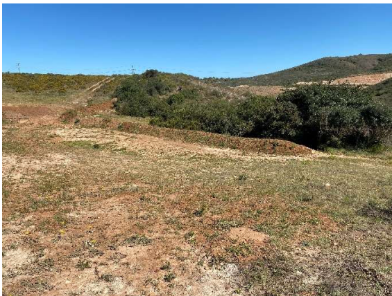
Detention Swales created underneath Phase 4 to collect stormwater and surface runoff from Phase 4 and 9
