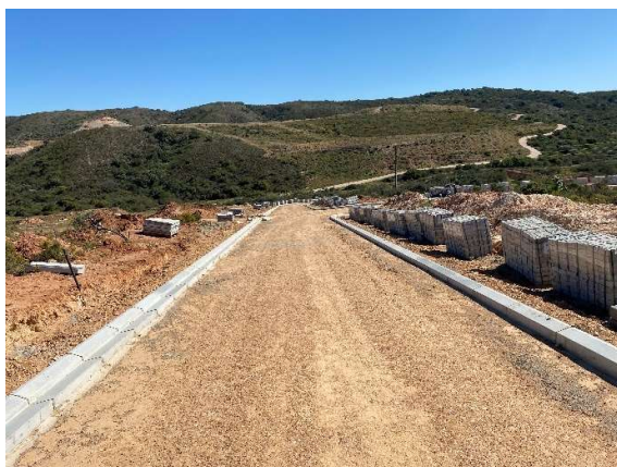
Internal road being constructed within Phase 9.
