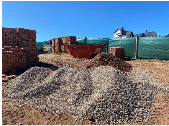
Material stockpiles within construction footprints.
