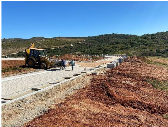
Internal road being constructed within Phase 9.
