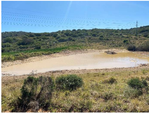
Detention pond beneath Phase 9.
