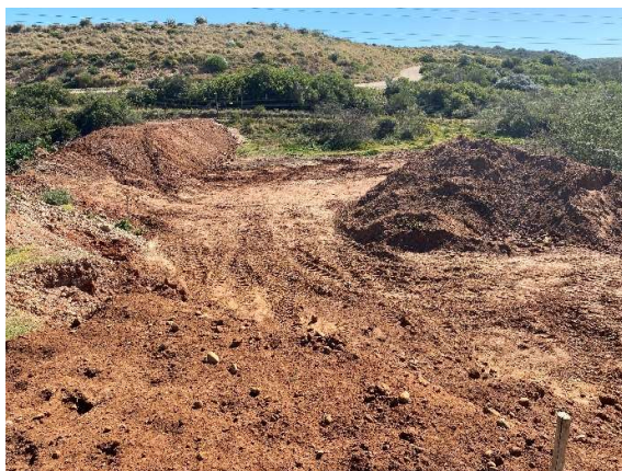
Detention pond being constructed beneath Phase 9 and 10.
