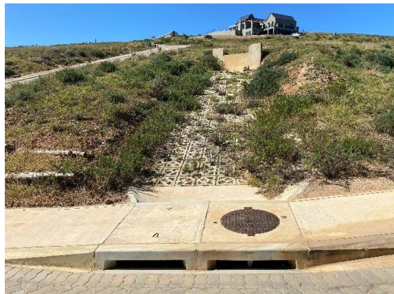
Grassblocks to act as energy dissipation along the west of Phase 11 along the access road.
