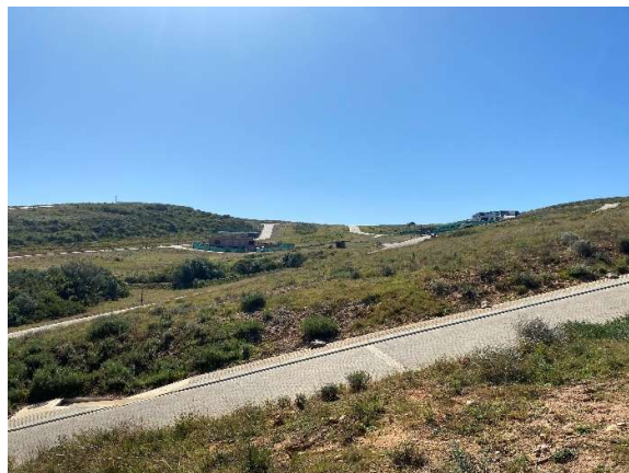
Condition of the site toward Phase 12 (middle left) and Phase 11 (top right).
