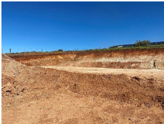
Excavation for the building of the School off Matunyane Street.
