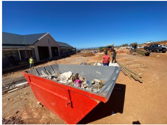
Waste skip present at the school construction site.
