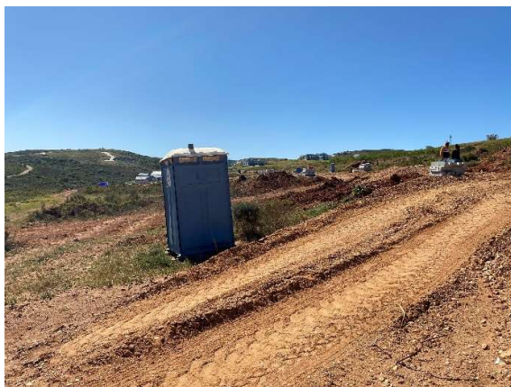
Chemical toilet within Phase 9.
