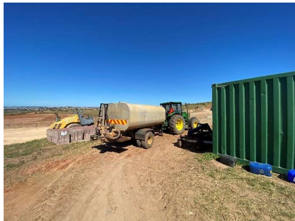
Watering truck available for dust suppression at the school construction site.
