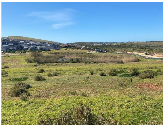
Detention Pond/Wetland between Phase 1 and 2, and Phase 19 under construction.
