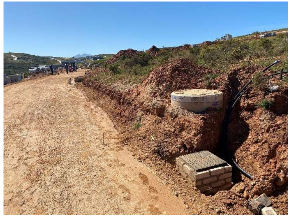
Stormwater and grey water systems being installed within Phase 9.
