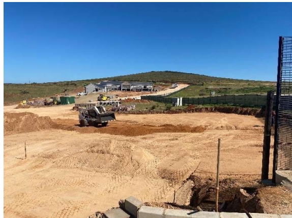
Construction of the Business zone and the school site underway as seen from the entrance to the estate.
