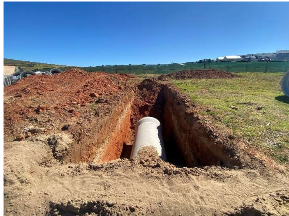
Civil services being installed within Phase 19.
