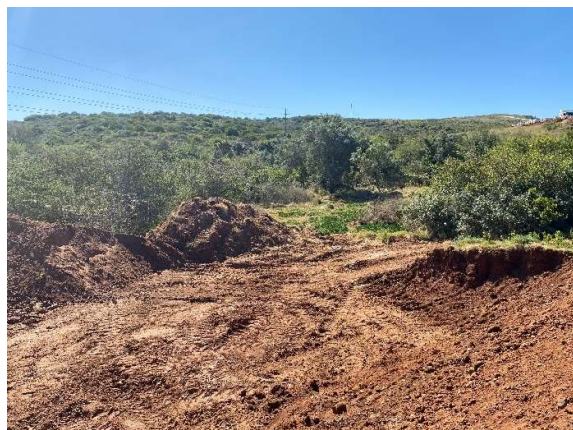
Detention pond being constructed beneath Phase 9 and 10.
