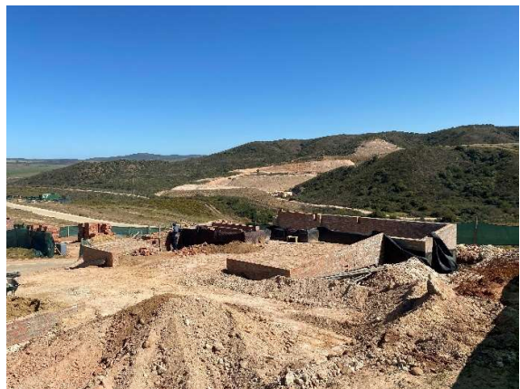
Construction of a single residence.
