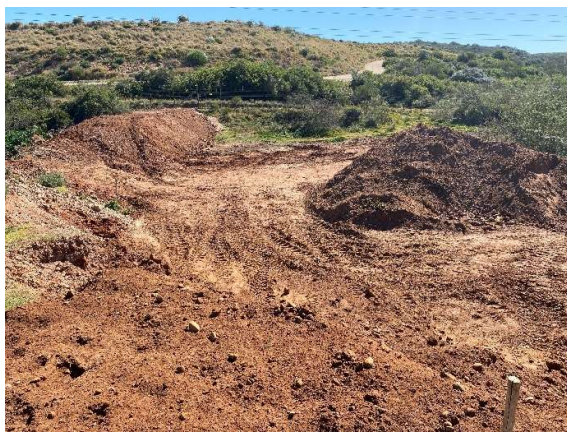
Detention pond being constructed beneath Phase 9 and 10.
