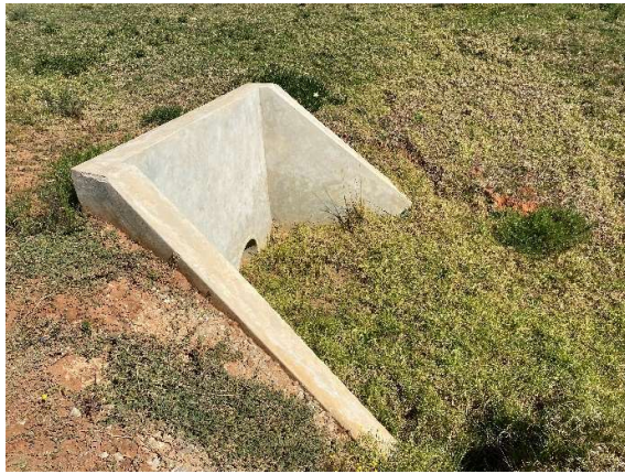
Stormwater culvert outlet along the access road north of Phase 10.
