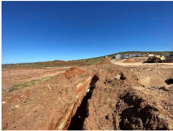
Civil services being installed within Phase 19.
