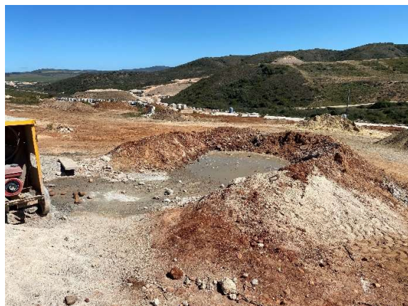
Cement batching pond within Phase 9 to contain runoff.
