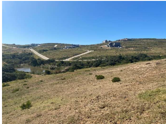
Detention pond Phase 10, 14, and 12.
