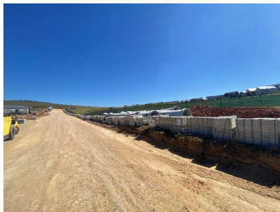
Internal access road within Phase 19. Material for the road verges layed down temporarily along the road.
