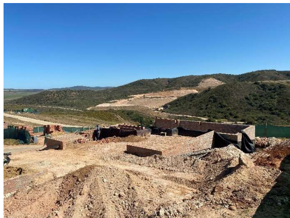
Construction of a single residence.
