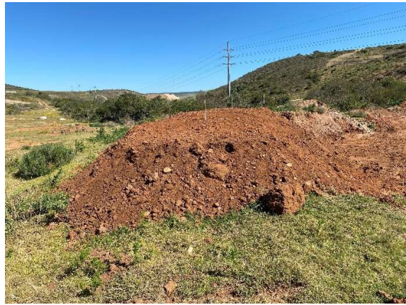
Detention pond being constructed beneath Phase 9.
