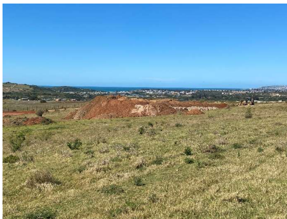
Stockpiles of excavated material and topsoil adjacent the school within the development footprint.
