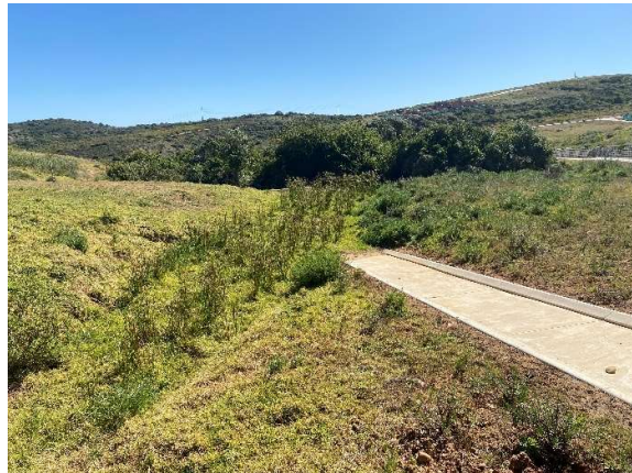
Stormwater infrastructure outlet along the access road north of Phase 10.
