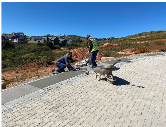
Road verges being constructed within Phase 9.
