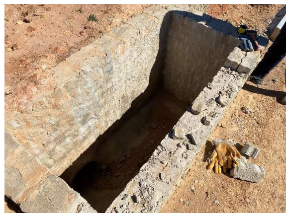
Stormwater infrastructure along the road.
