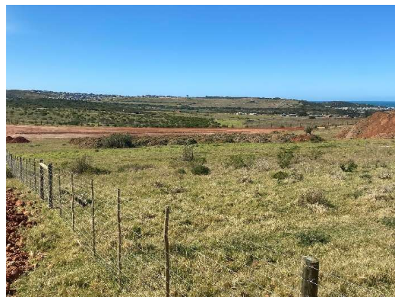
Topsoil stockpiles adjacent the school within the development footprint.
