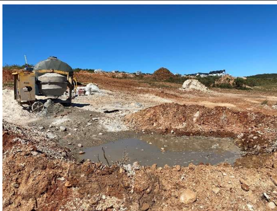
Cement batching pond within Phase 9 to contain runoff.
