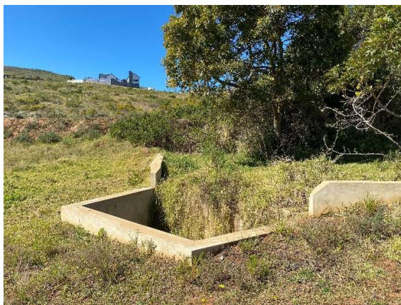
Stormwater culvert intake towards the west of Phase 11.
