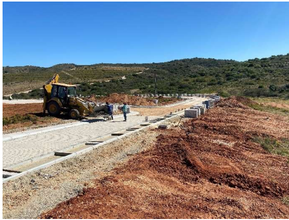
Internal road being constructed within Phase 9.
