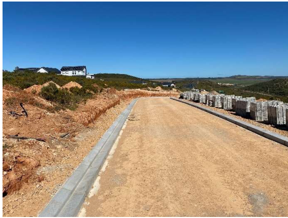
Internal road being constructed within Phase 9.
