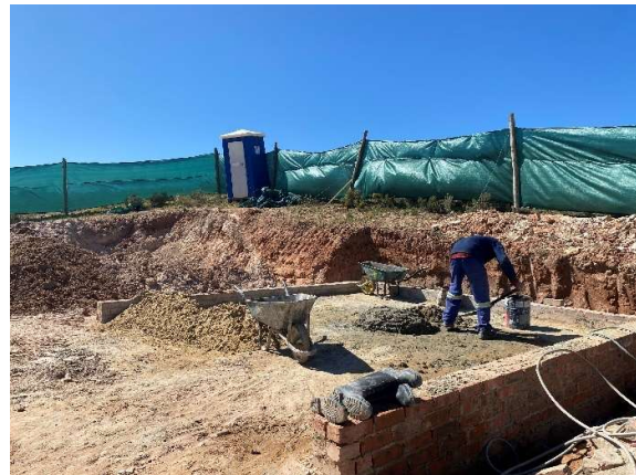
Cement mixing on the foundation of a residential platform.
