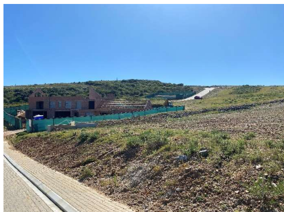
Construction of a large residence within Phase 12.
