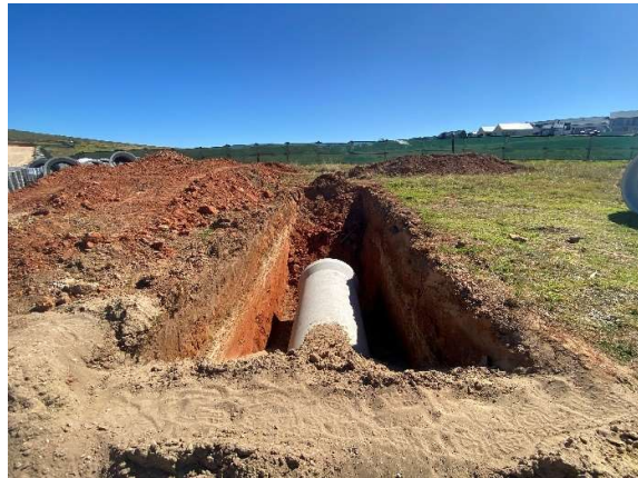
Civil services being installed within Phase 19.
