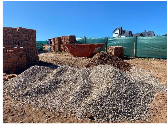
Material stockpiles within construction footprints.
