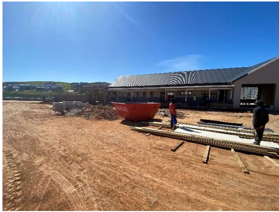
Temporary material laydown area within the construction footprint of the school.
