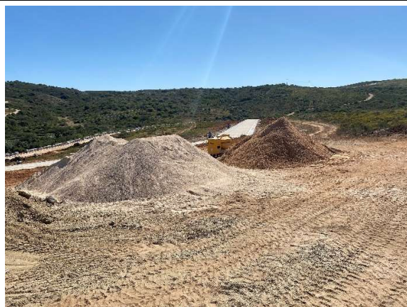
Material stockpiles along the road sections within Phase 9 on the proposed erven locations.
