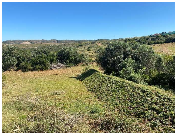
Detention Swale within Phase 10.
