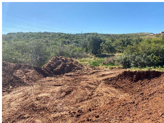
Detention pond being constructed beneath Phase 9 and 10.
