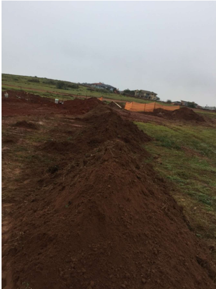
No-Go netting in place as approved by ECO.
