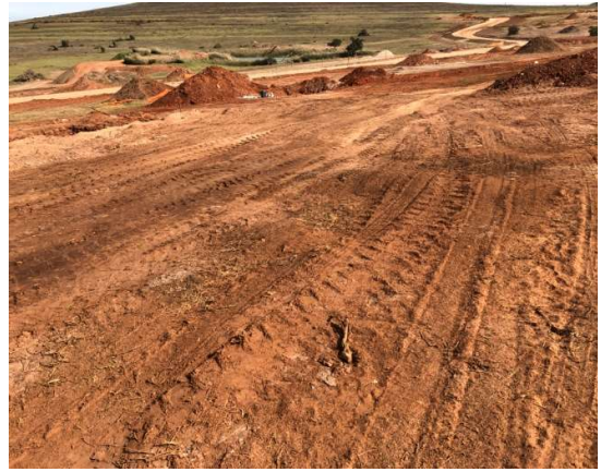
Topsoil is being replaced as top layer.
