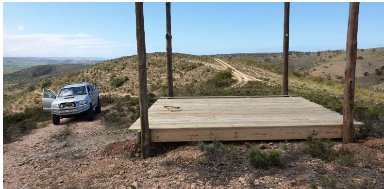
Decking at first resort unit
