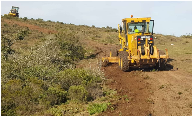
Construction of the main road to the resort area.
