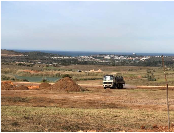
Water truck spraying water on haul roads.
