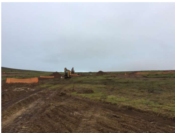
Construction area is pegged out to illustrate work area.
