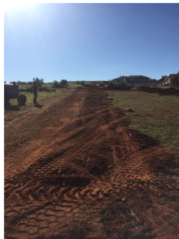
Topsoil has been placed on top of the subsoil.
