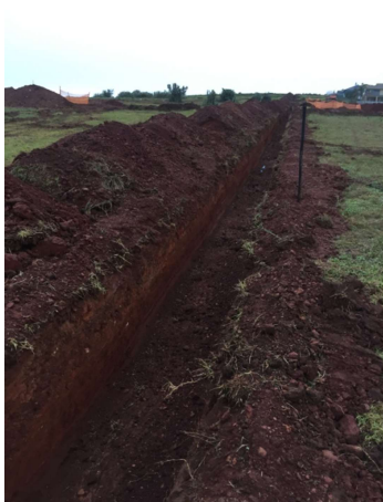
Topsoil is kept separate from subsoil.
