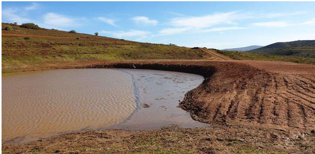
Storm water detention dam filled with storm and slowly released the peak of the flood.
