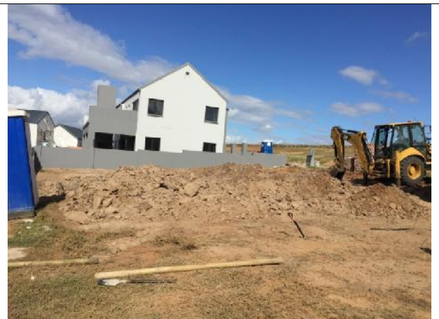
Erf 6620 – No-Go demarcation being installed.
