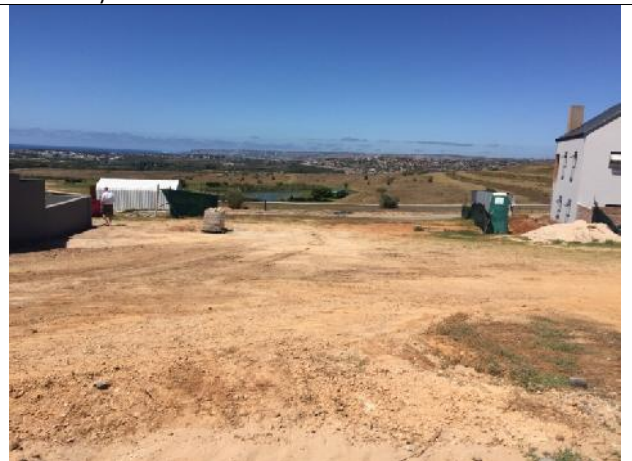
The construction material on Erf 6619 have been removed (10.02.2021).
