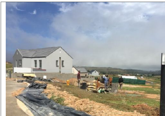
Concrete mixing should be done on a protective sheet with a small bunding wall to prevent contamination and possible run-off
