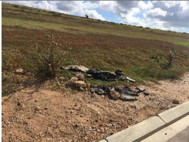
Excess tar must be removed (phase 3) and disposed of at an authorised disposal facility.
