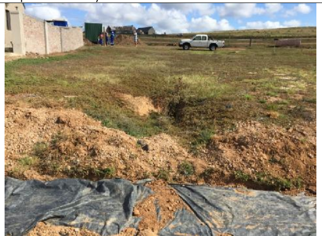
The sidewalk contractor must rehabilitate any disturbed areas as they progress (reshape the areas and seed with indigenous grass seed mixture).
