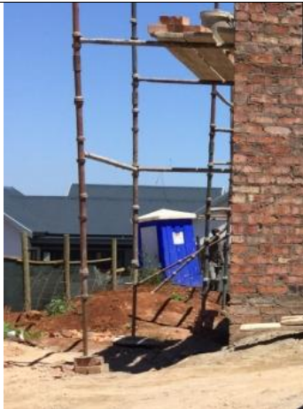
Individual home builder provide portable chemical toilets for staff during construction phase (Erf 6631)
