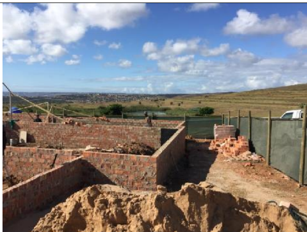
Erf 6549 - No-Go demarcation indicating the work zone.
