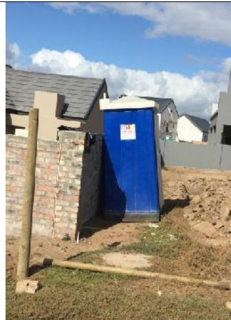
Individual home builder provide portable chemical toilets for staff during construction phase (Erf 6620)
