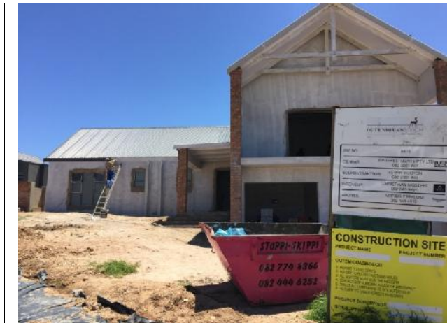
Individual home builders proved suitable skip or bins on site (Erf 6644).
