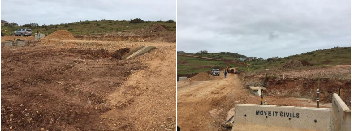
2021.09.30 – Ongoing construction of the civil services in phase 10 – topsoil replaced back (on top).
