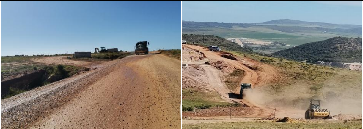
2021.09.08 – Water is sprayed on the road leading to phase 10 to minimize the dust.
