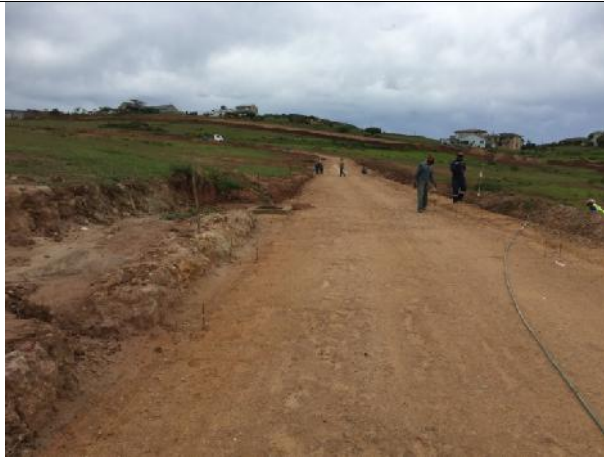
2021.10.28 – Ongoing construction of the roads in phase 10.
