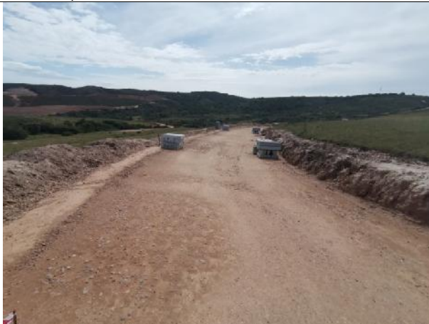
2021.10.22 – The installation of the curbs in phase 10.
