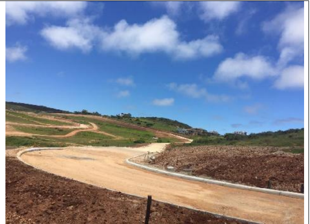
2021.12.09 – Ongoing construction of the roads in phase 10.
