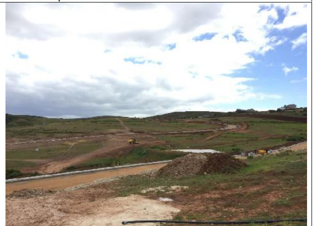
2021.11.18 – The ongoing construction in phase 10 (civil services).
