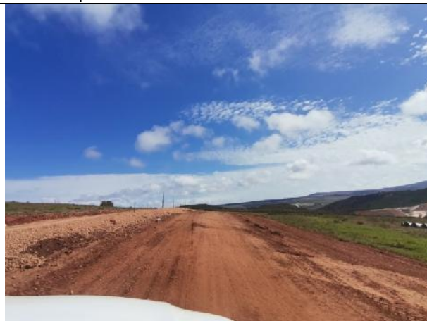
2021.11.11 – The temporary haul road to phase 10.
