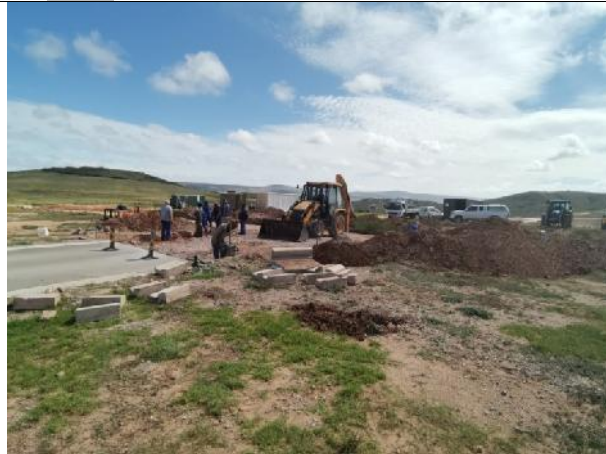
2021.11.11 – Ongoing construction of the roads in phase 10.
