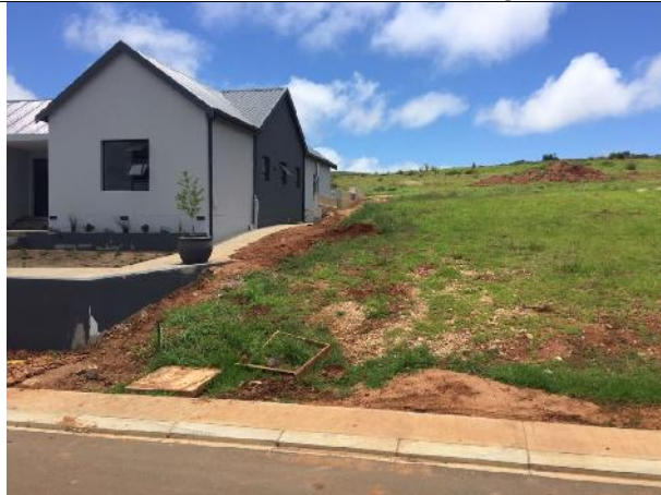
Completed house – rehabilitation recommendations were given to the contractor
