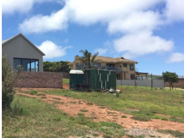
2021.12.09 – Ablution facilities for home construction staff – each site has its own toilet.
