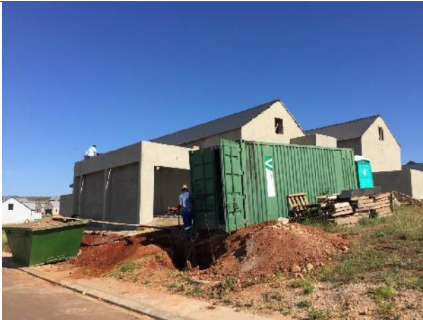
2022.01.27 – Ablution facilities and storage container for house construction staff – each site has its own toilet.
