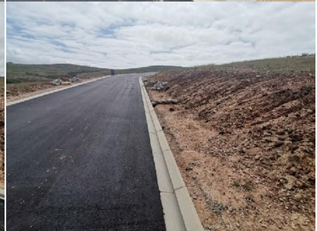
2022.01.27 – Sandbags are used for stormwater management in phase 10. Final shaping and rehabilitation will be done once the sidewalks are completed.
