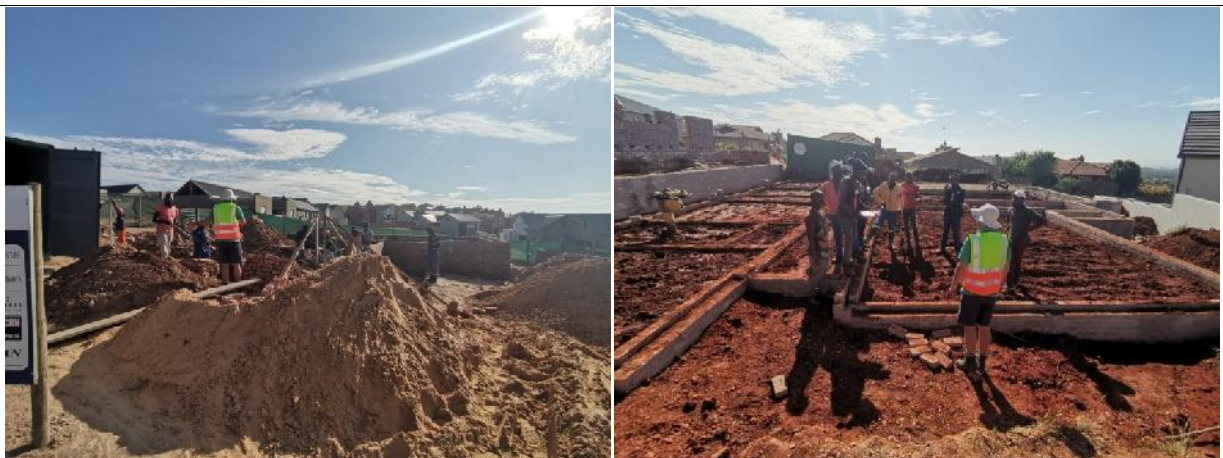
2022.02.02 – Environmental Induction done with construction teams.
