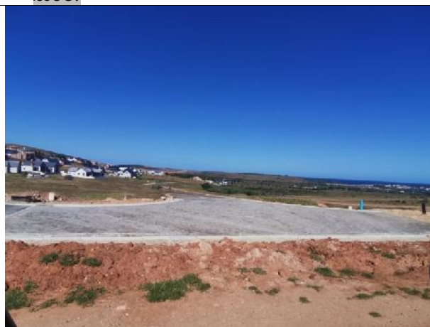
2022.02.17 – Ongoing construction of Mafunyane Street.
