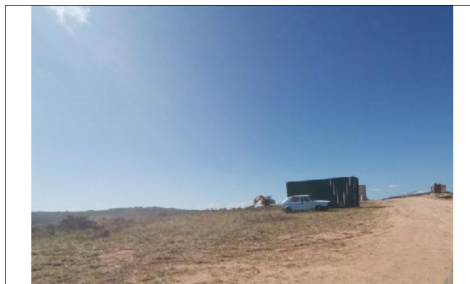
2022.02.17 – Construction site camp of phase 10
