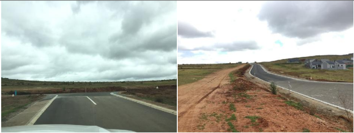
2022.02.25 – Construction of Mafunyane Street is near completion.
