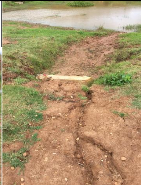
2022.02.25 – Stormwater outlet (phase 10) additional rehabilitation recommended (see Section 7) - the estate management is continuing with rehabilitation
