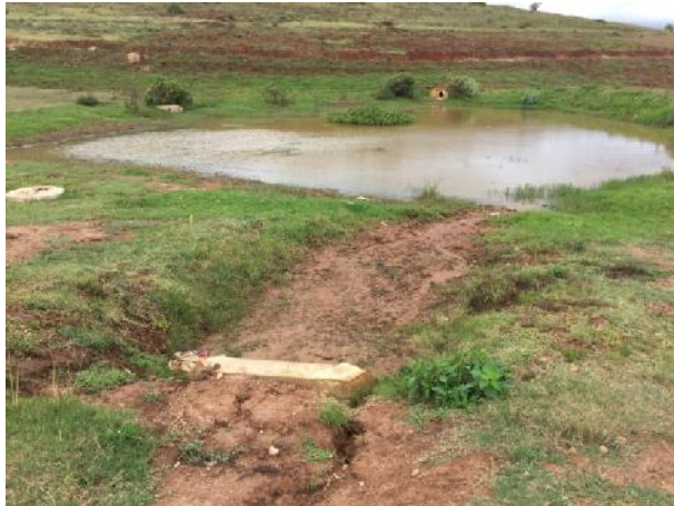
2022.02.25 – Stormwater outlet (phase 10) additional rehabilitation recommended (see Section 7) - the estate management is continuing with rehabilitation
