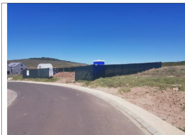
2022.03.18 – The demarcation around Erf 6560 in phase 2.
