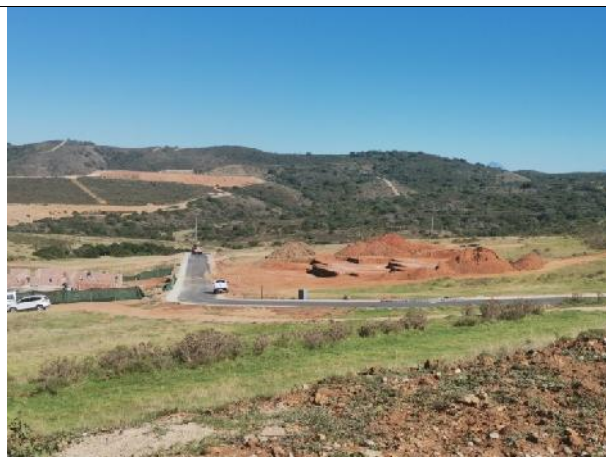
2022.03.18 – Construction of Erven in Phase 10.
