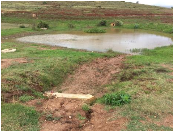
2022.03.23 – Stormwater outlet (phase 10) additional rehabilitation recommended (see Section 7) - the estate management is continuing with rehabilitation
