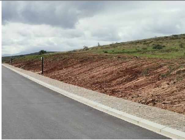
2022.04.08 - The steep road verges are to be shaped with horizontal grader lines to prevent vertical erosion and then seeded with the indigenous grass seed mixture.
