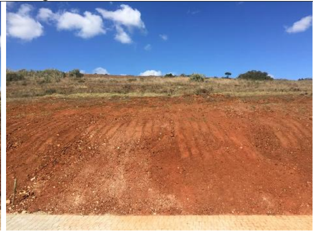
2022.04.29 – Vertical shaping was done as opposed to horizontal. HOA must now monitor the slopes for signs of soil erosion until the grass is established.
