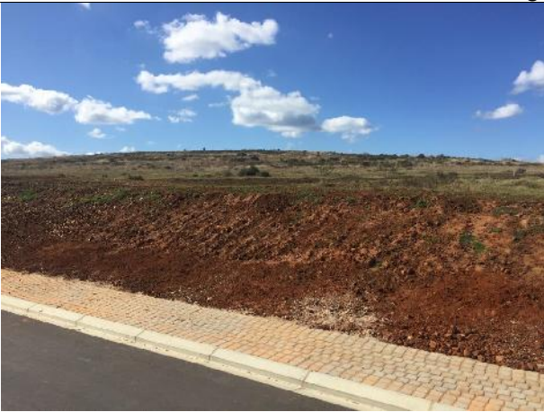
2022.04.29 – Vertical shaping was done as opposed to horizontal. HOA must now monitor the slopes for signs of soil erosion until the grass is established.
