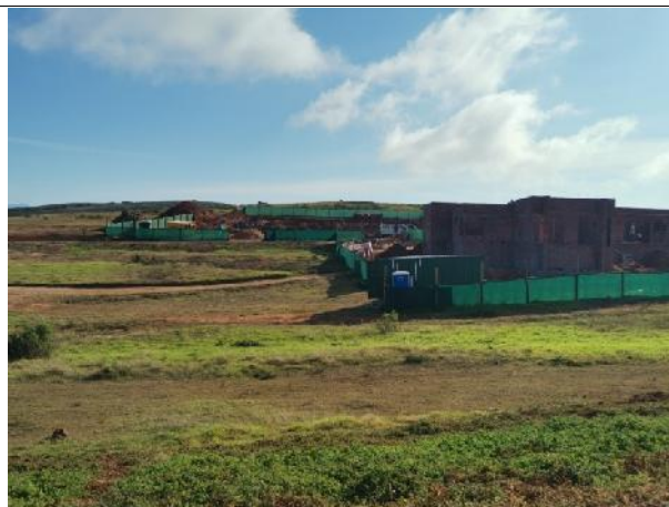
2022.04.13 – Construction of Erven in Phase 10.
