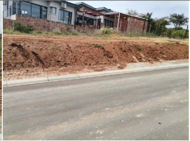
2022.04.08 - The steep road verges are to be shaped with horizontal grader lines to prevent vertical erosion and then seeded with the indigenous grass seed mixture.
