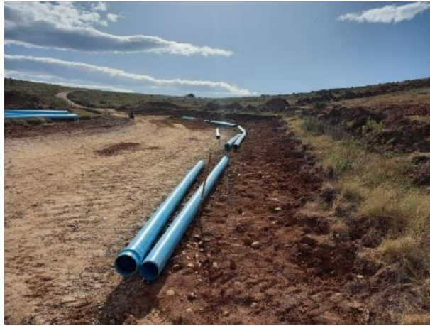
2022.07.01 – Civil services installation and construction of internal roads for phases 11 & 13.
