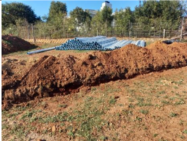
2022.07.13 – Storage of construction material for civil services installation.
