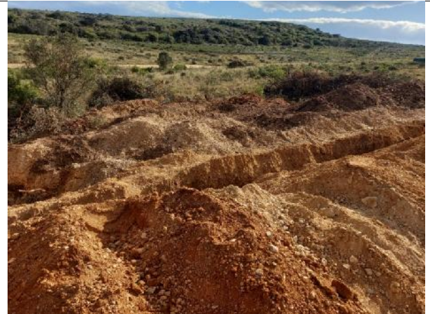
2022.07.01 – Topsoil and subsoil is kept on separate sides of the trench.
