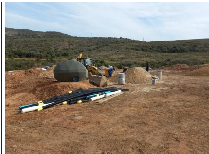
2022.08.11 – dedicated cement mixing and storage area.
