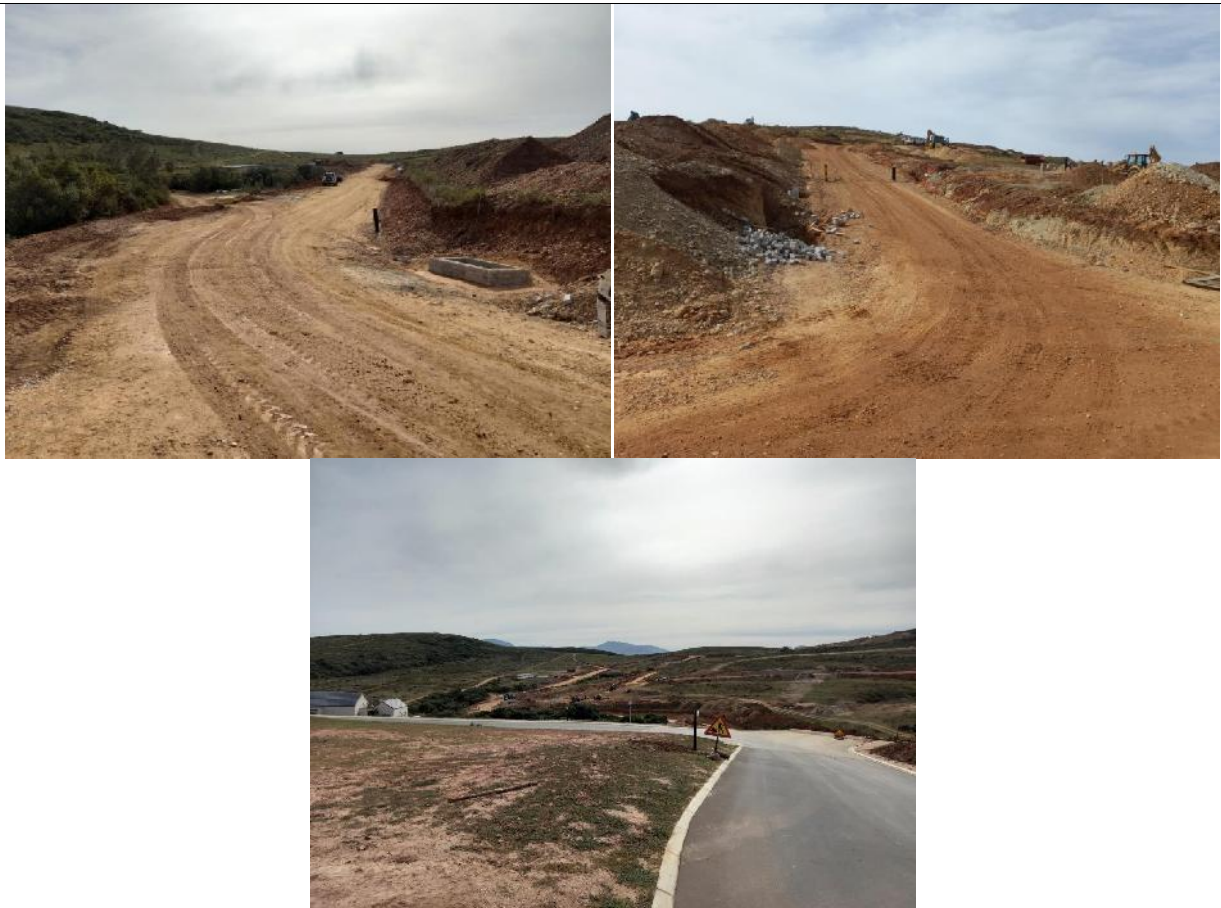
2022.08.11 – internal access roads of phases 11 & 13 in progress.
