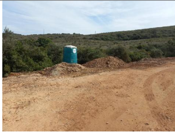
2022.08.11 – Ablution facilities are available on site for staff.
