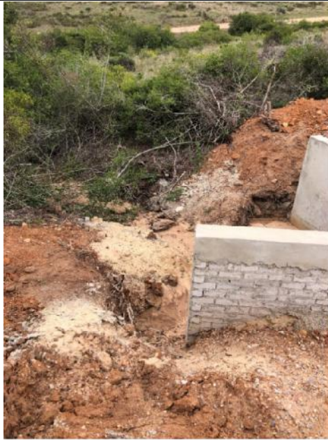
Silt fence and shaping of the stormwater outlet required on top
