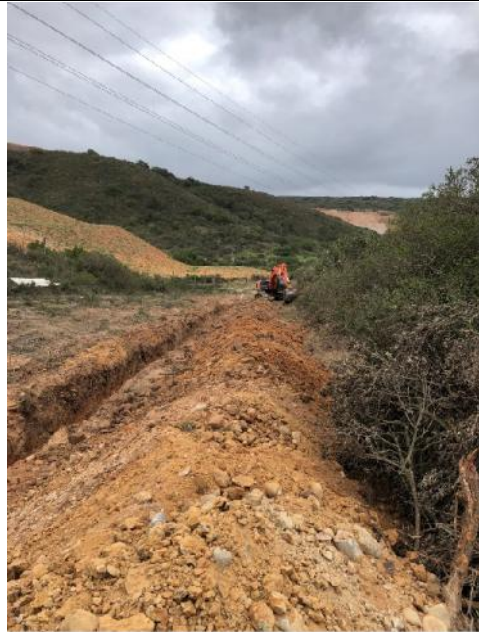
Trench – when closing, topsoil must be
