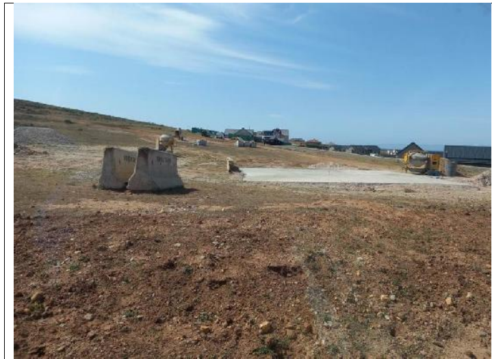
Construction site camp must be demarcated – cement slab processing area
