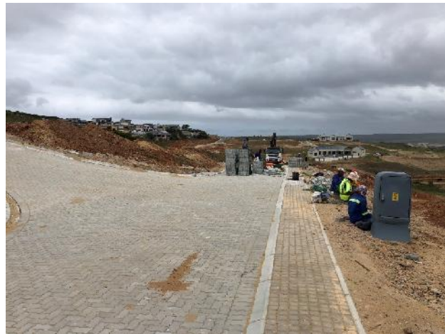
Construction site – phases 11 & 13
