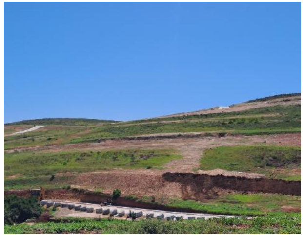
Stormwater swales are constructed as construction progresses
