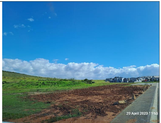
Temporary parking area at the entrance gate was closed and ripped.
