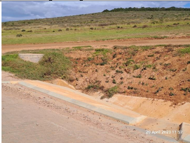
Stormwater channel sides rehabilitation in progress.
