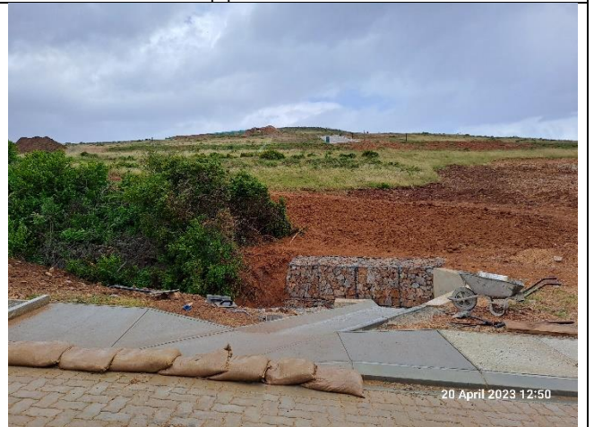
Stormwater channel in phase 11
