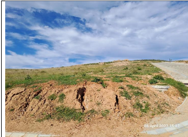
Erosion protection and rehabilitation required on steep slopes – phase 11 (contractor is busy with rehabilitation).
