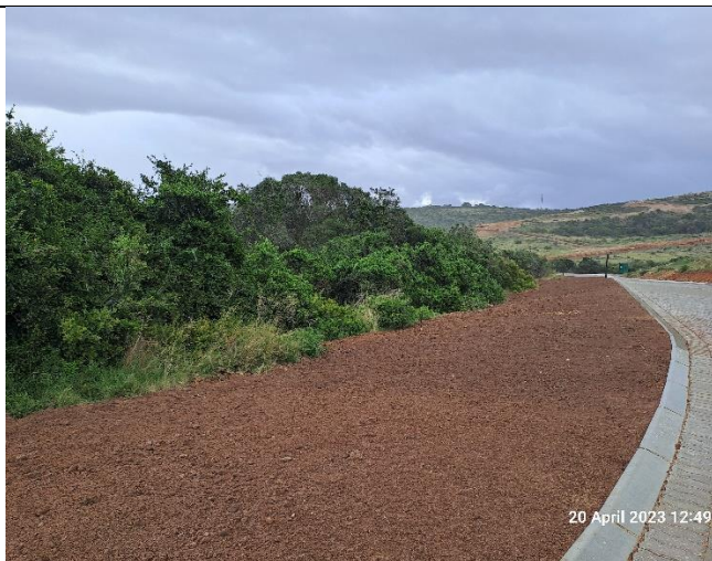
Topsoil was replaced and can now be seeded with the indigenous grass seed mixture.
