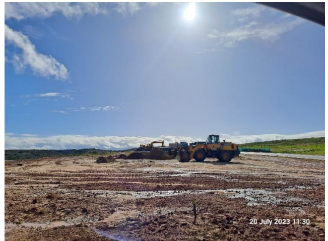
Site camp – rehab the disturbed areas that will not be used during construction of future phase.
