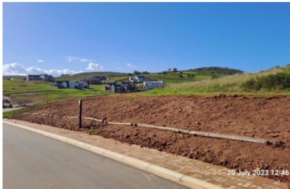
(2023.07.20) – The landscape committee has started to rehabilitate the road verge along Mafunyane street.
