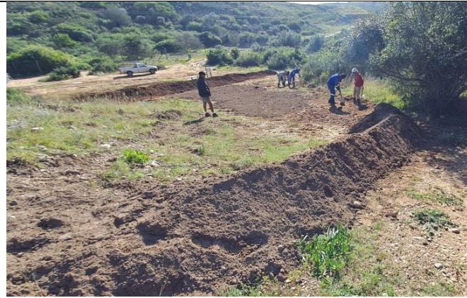
(2023.07.13) – Berms were created on the western side to direct and manage stormwater.
