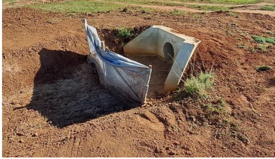
(2023.07.13) – Stormwater outlets in phase 4 has been shaped and silt fences have been cleared.
