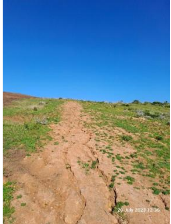
Sewer line – rehab required
