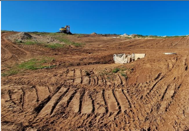
(2023.07.13) – Large areas of compacted bare soil have been shaped and covered with topsoil – grass seeds and vegetation are now required.
