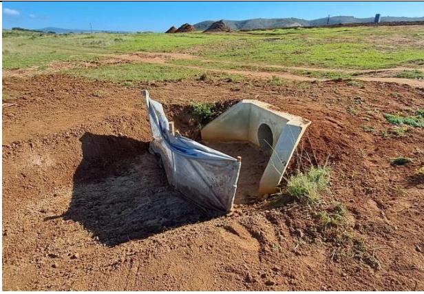
(2023.07.13) – stormwater outlets have been shaped and topsoil is replaced.
