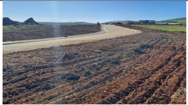
(2023.07.13) – road verges were shaped and covered with topsoil.
