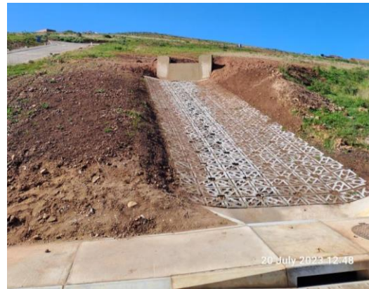
(2023.07.20) – stormwater management – phase 11 to mitigate slope erosion.
