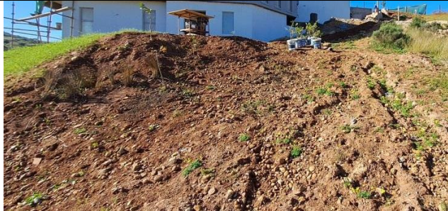
(2023.07.13) – phase 10 – rehabilitation in progress.
