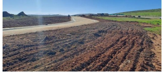
(2023.07.13) – Road verges have been reshaped in phase 4. Continuous monitoring is required.
