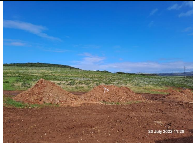
Few stockpiles still to be removed once soil is dried out a bit more.
