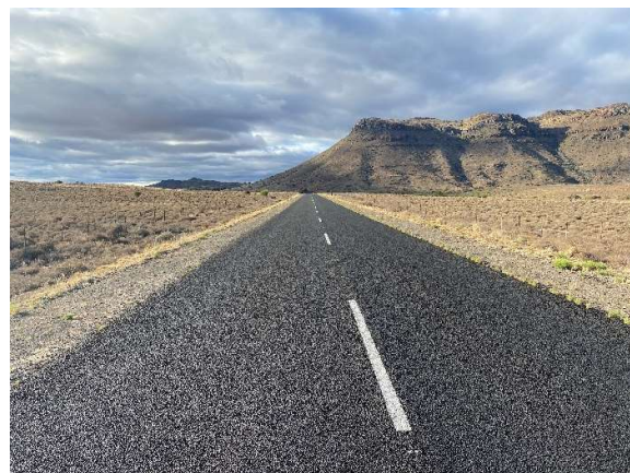
Condition of the new road surface and cleared road reserve at km 28.20 along the TR16/9.
