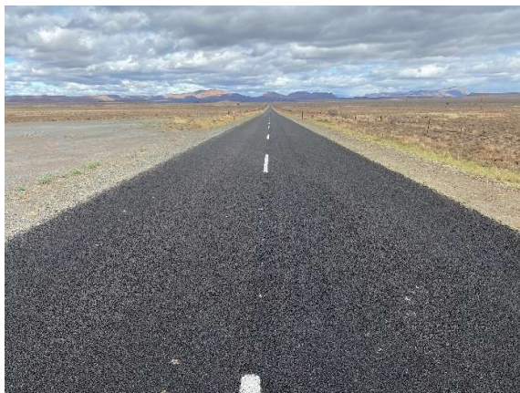
Condition of the new road surface and the cleared road reserve adjacent to stockpile area 2.
