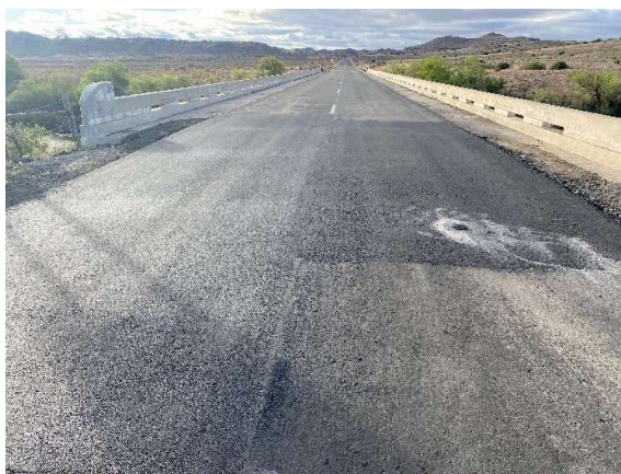
Current condition of the Buffalo River bridge at Km 26.94 along the TR16/9.
