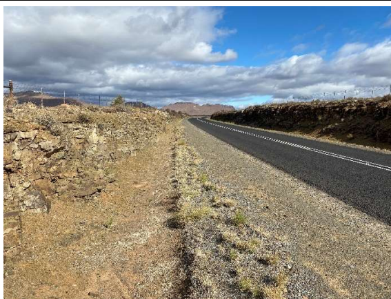
Cleared road reserve with stormwater drainage channels created at the road reserve shoulder along the TR 16/9.
