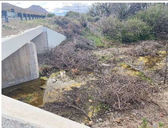
Upgraded culvert at km38 on TR 16/9 where some cleared vegetation debris still noticable.
