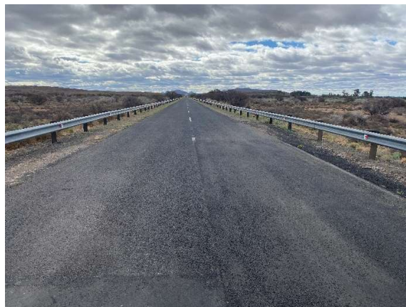
Condition of the new road surface and newly installed guardrails at Km17.36 along the TR 16/9.
