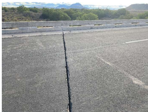
Buffalo River bridge deck where seals between the joints have been removed in preparation for bridge upgrades.
