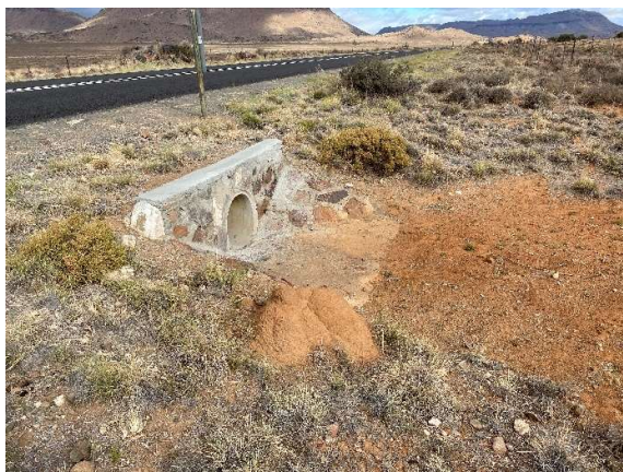
Culverts upgraded with new concrete repairs, daylighting, stone-pitching and clearing of vegetation.
