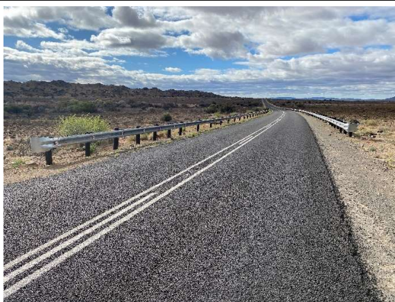
Condition of the new road surface and guardrails along the TR 16/9 at Km 25.2.
