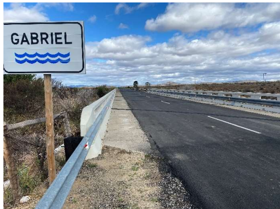
Newly installed guardrails at B4611 on TR16/8 at Km 46.11 (Gabriel Stream).
