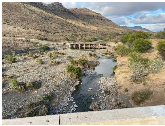
The old bridge upstream of the Buffalo River bridge as seen from the deck of the bridge towards the northeast.
