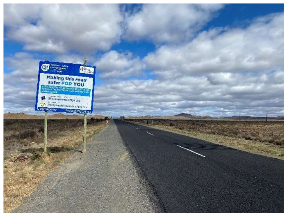
Construction information notice board placed at approximately Km 0.25 on TR 16/9.
