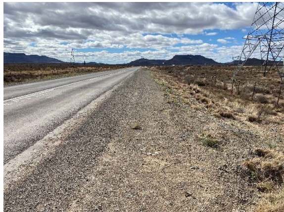
Cleared road reserve at Km 44 on TR 16/8 where vegetation within the road reserve was removed.
