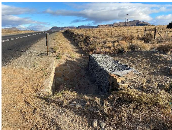
Box culvert to dissipate stormwater energy and channel towards existing culvert at km 27.29 along the TR16/9.
