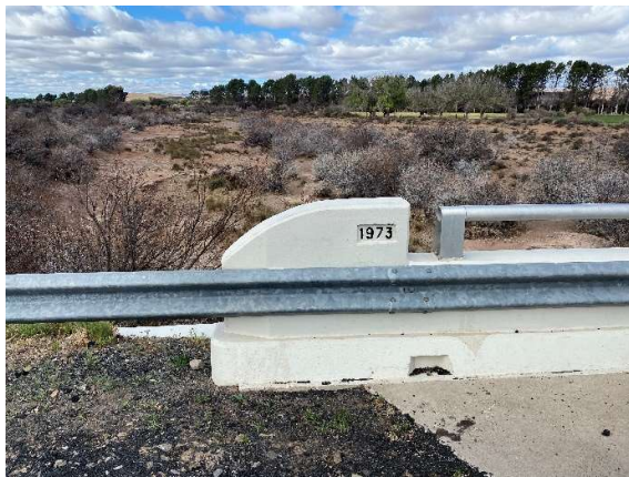
Numbering of the Brakvallei River bridge displays along the new precast concrete handrails.
