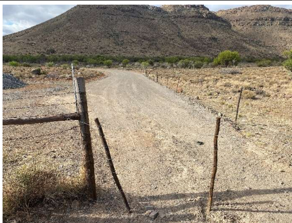
The southern offramp and entrance to the gravel bypass road which is to lead across Buffalo River.
