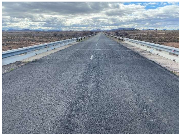
Condition of the completed Brakvallei River bridge road surface as seen towards the northwest.
