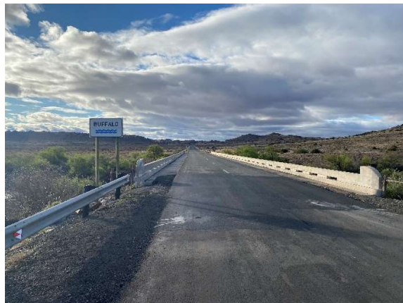
Current condition of the Buffalo River bridge at Km 26.94 along the TR16/9.
