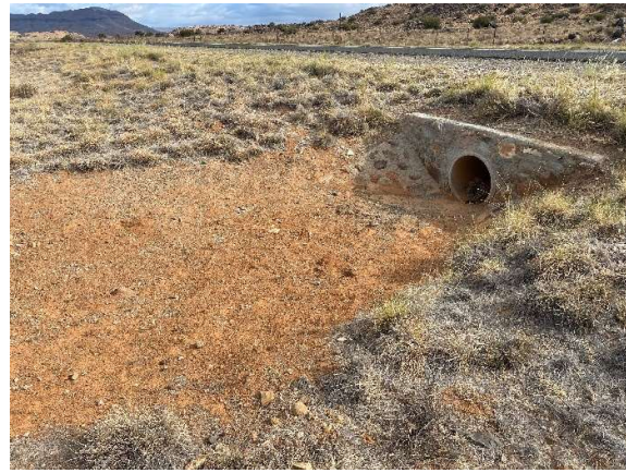
Culverts upgraded with new concrete repairs, daylighting, and clearing of vegetation.
