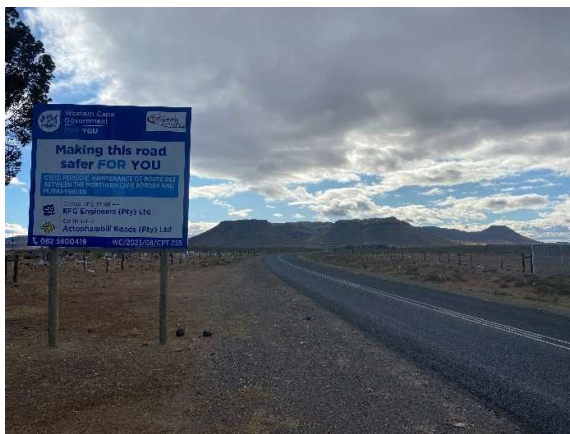
Construction information notice board placed at approximately Km 41.3 on TR 16/9.
