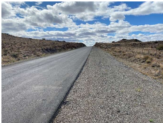
Condition of the road reserve along the TR 16/9 as seen towards the northwest.
