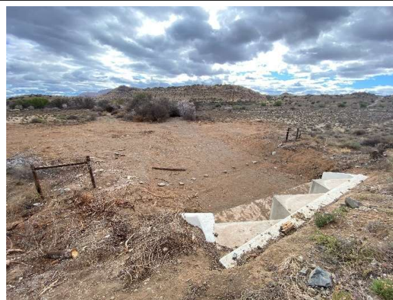
Downstream of box culvert shows daylighting required given the topography to prevent damming of water.
