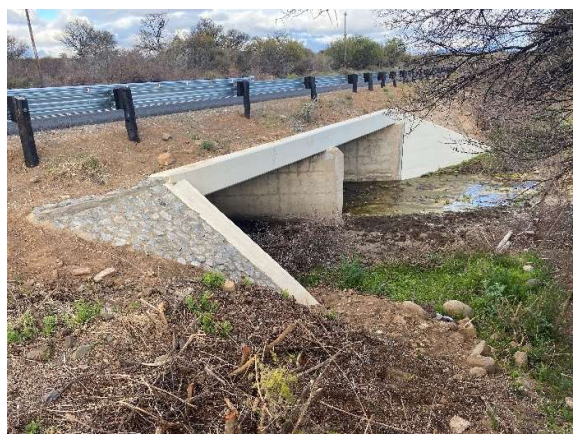
Upgraded culvert at Km38 on TR 16/9 with new concrete structures, erosion control, and clearing of vegetation.
