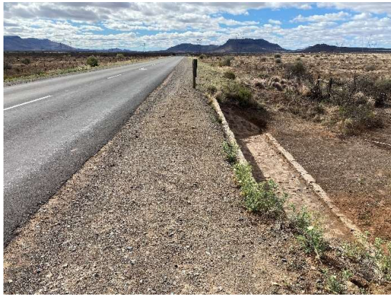
Upgraded culvert at Km 44.69 on TR 16/8 with repaired concrete and stone-pitching, daylighting and vegetation clearance.
