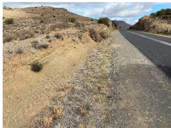
Stormwater drainage channel along the TR 16/9 at Km 24.9 of the road reserve along the route.
