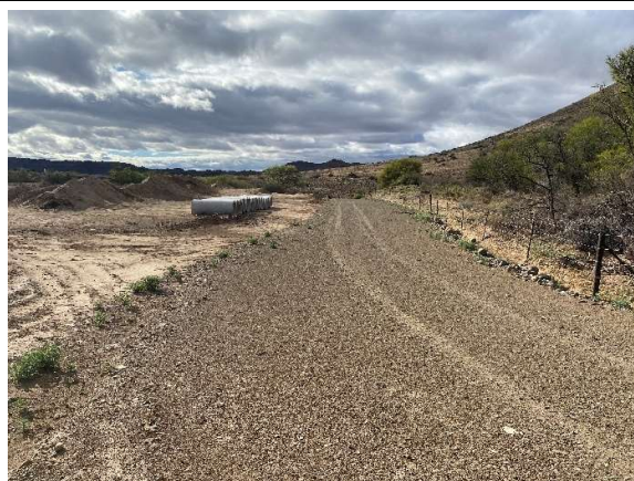
The southern gravel bypass road which is to lead across Buffalo River.
