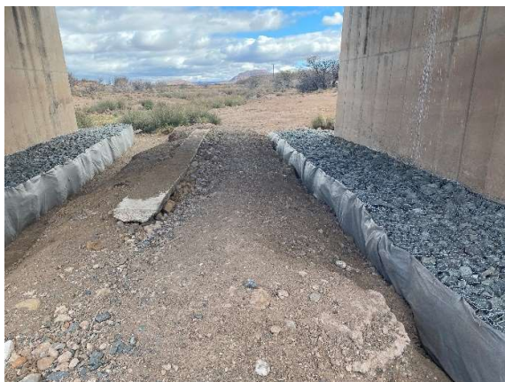
Below the Brakvallei River Bridge as seen towards the south.
