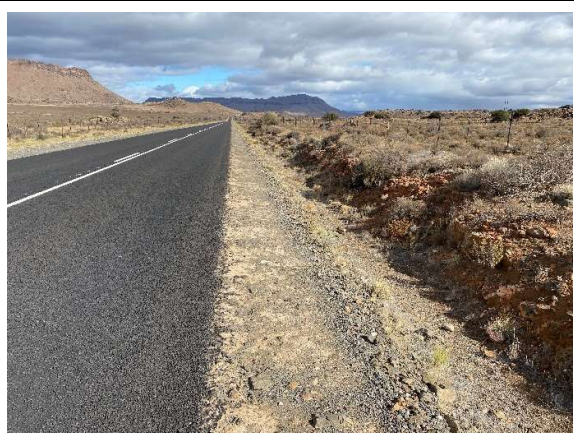
Cleared road reserve with stormwater drainage channels created at the road reserve shoulder along the TR 16/9.
