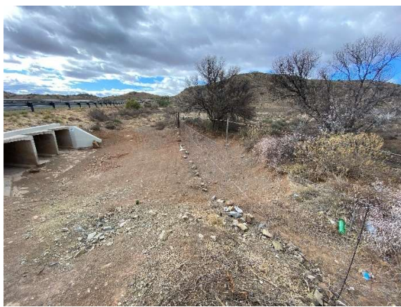
Upgraded box culvert 11425 at km24.45 along the TR16/9.
