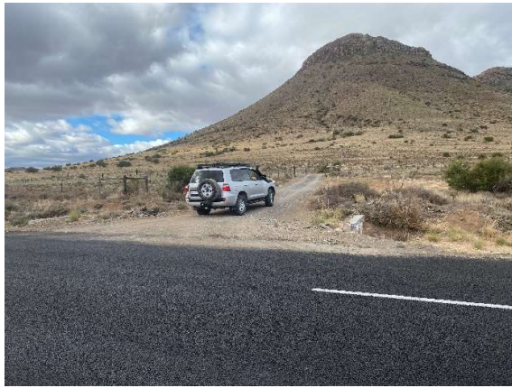
The entrance to the northern section of the gravel bypass road at km 26.56 along the TR16/9.
