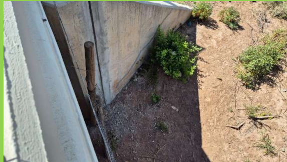
The ECO provided this photographic proof on the 26 th of November that the concrete spills in the Gabriel River has been removed.
