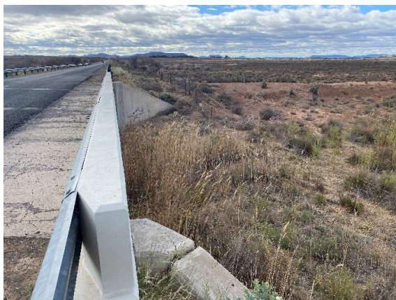
Upstream condition of the Brakvallei River bridge.
