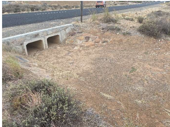
Culvert upgraded adjacent to the northern bypass road with repaired concrete structures and daylighting.
