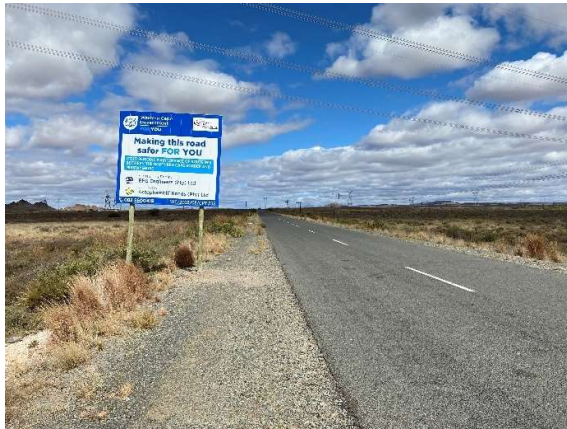
Construction information notice board placed at approximately Km 43.5 on TR 16/8.
