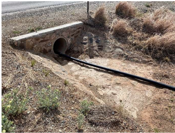
Culvert upgrading includes repaired concrete structures, stone-pitching, and vegetation clearing.
