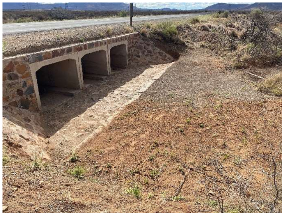
Culvert upgrading includes repaired concrete structures, stone-pitching, erosion control, and vegetation clearing.
