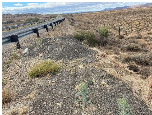
Small stockpile of stones to be removed at the new guardrail installation along the TR 16/9.
