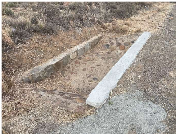
Culvert upgraded adjacent to the northern bypass road with repaired concrete and stone-pitching maintained.
