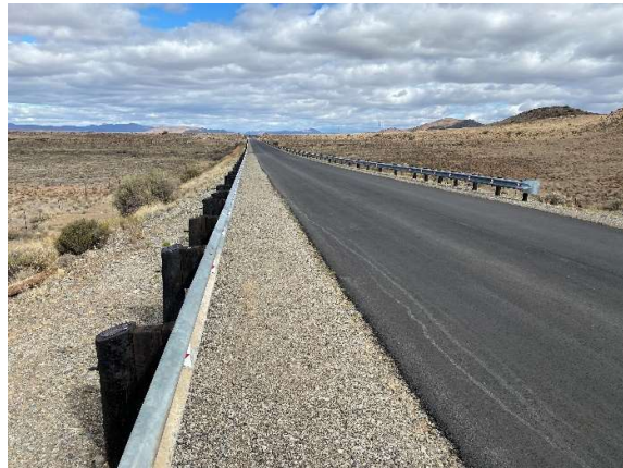
Newly installed guardrails along the TR 16/9 as seen towards the southeast.
