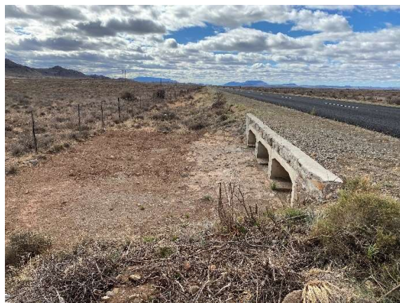
Culvert upgraded with repaired concrete and new stone-pitching, daylighting and vegetation clearance.
