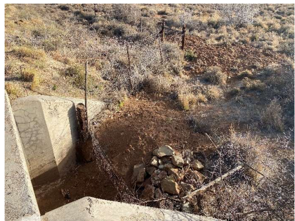
Culverts upgraded with concrete repairs, erosion control, and clearing of vegetation.
