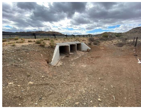
Upgraded box culvert with new concrete structures, erosion control, daylighting and clearing of vegetation.
