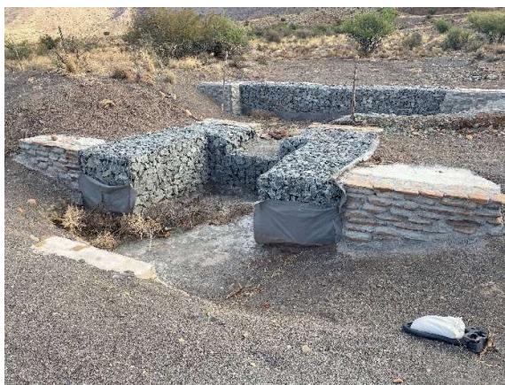
Newly installed gabion baskets for sediment within the road reserve at approximately Km 34.6 on TR 16/9.
