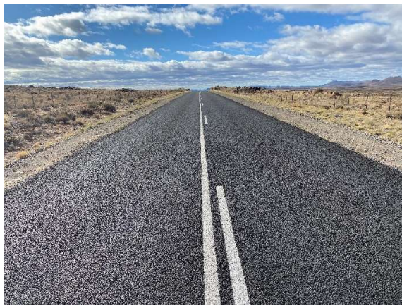
Condition of the new road surface and cleared road reserve along the TR 16/9.
