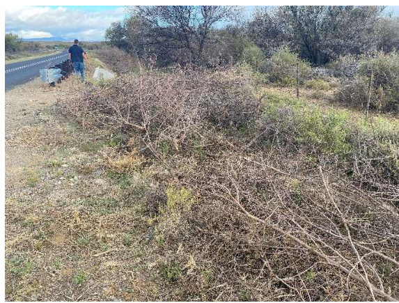
Cleared vegetation debris to be removed at upgraded culvert at Km38 on TR 16/9.
