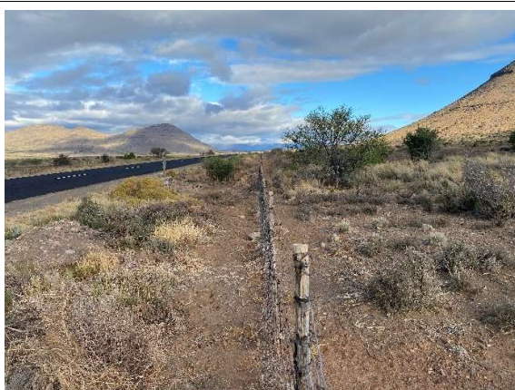
Cleared vegetation along the road reserve fence as firebreak condition along the route.
