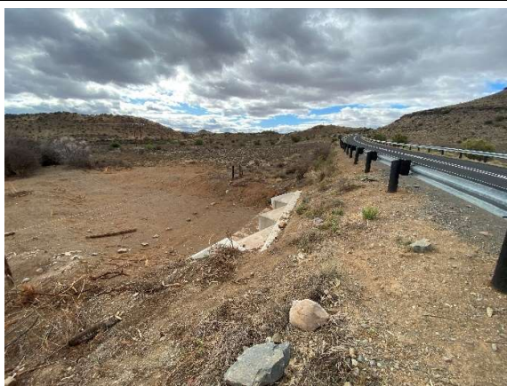
Downstream of box culvert with new concrete structures, erosion control, daylighting and clearing of vegetation.
