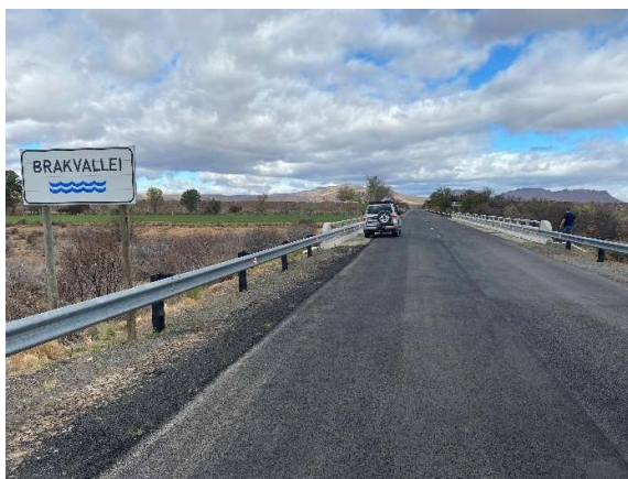
Condition of the new road surface and newly installed guardrails at Brakvallei River Bridge at Km 17.45.
