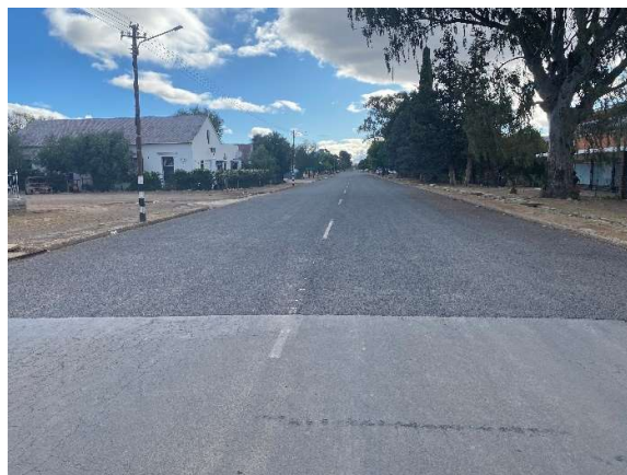
Contract end at Km 42 within the town of Murraysburg. Road surface redone, and surface work is now complete.
