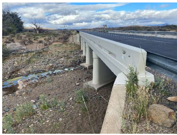
Ultkyk River bridge 4615: bridge deck resealed, joints and handrails installed, concrete repairs completed.
