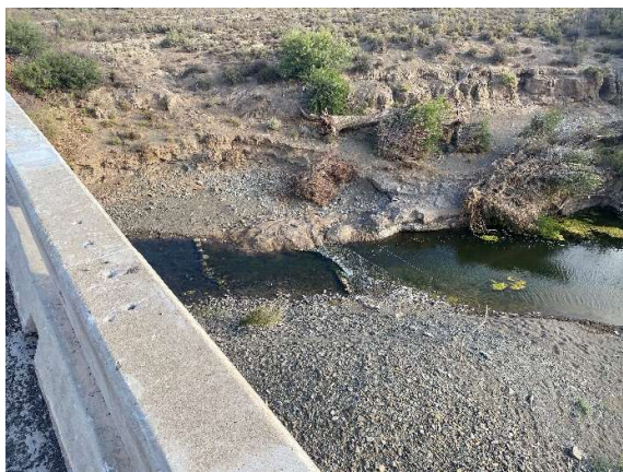
Downstream of the Buffalo River bridge as seen from the deck of the bridge.
