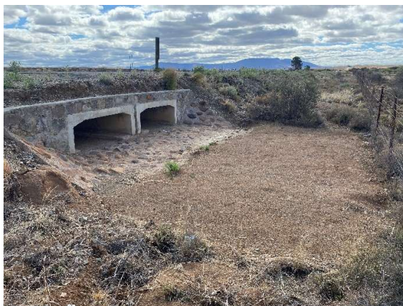
Km 46.75 on TR 16/8 with repaired concrete and stone-pitching, daylighting and vegetation clearance.
