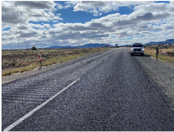
From approximately Km 0.25 on TR 16/9 showing the new road surface towards the northwest.
