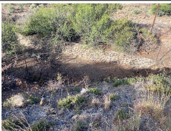
A stone-pitched side drains channel leading to a farm capturing the water from the road reserve.
