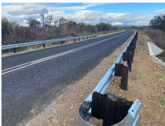
Newly installed guardrails at upgraded culvert at Km38 on TR 16/9.
