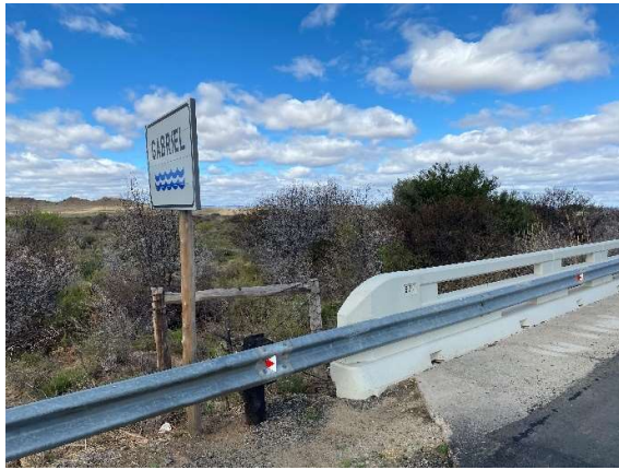
Condition of Gabriel River with newly installed guardrailings.
