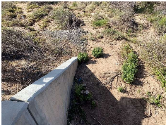
Concrete repairs at piers and wingwalls at the Gabriel River bridge.
