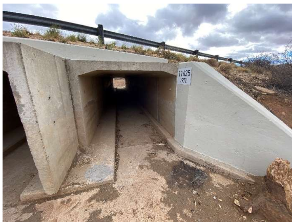
Culvert upgraded with concrete repairs apron slabs and cut off walls at culverts on inlet and crack repairs.
