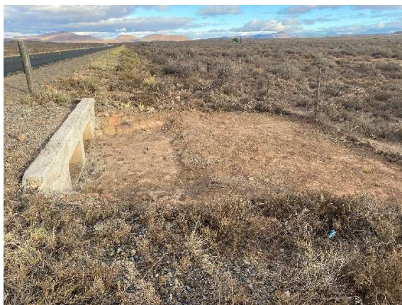
Culverts upgraded with new concrete structures, daylighting, and clearing of vegetation.
