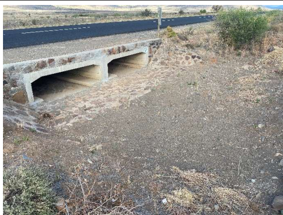
Culvert upgraded along the TR16/9 with repaired concrete and stone-pitching maintained.
