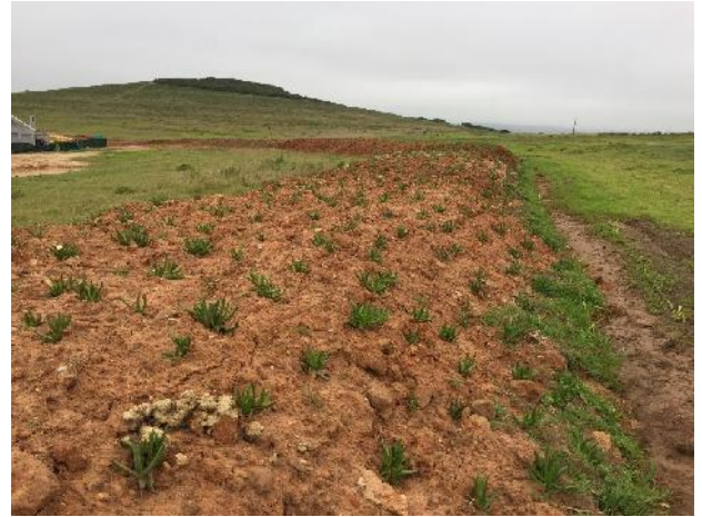
Rescued plants are planted on the stormwater deflection berm.
