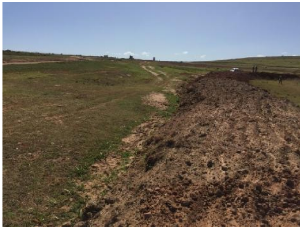
Stormwater deflection berm north of phase 2.
