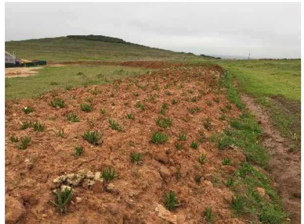
Stormwater deflection berm north of phase 2 - Vegetated.
