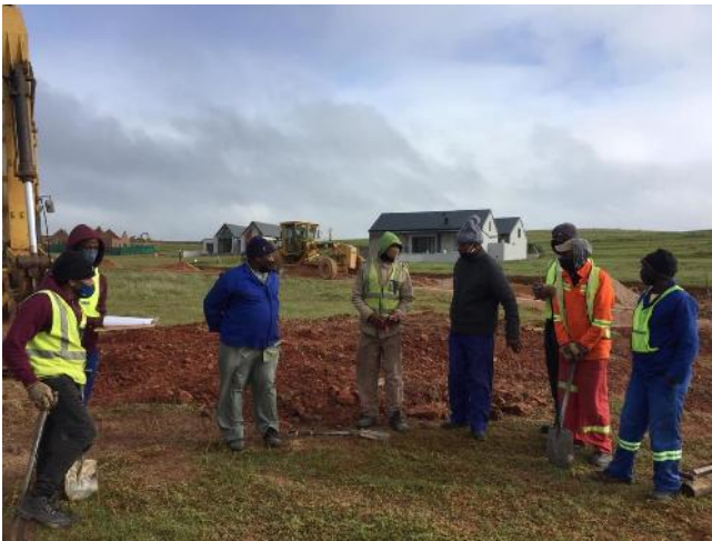
26 October 2020 – induction was given to construction staff members of the main access road contractor.
