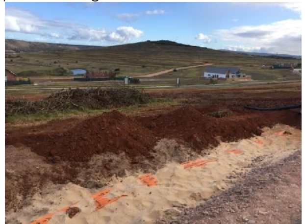
Topsoil is being replaced as top layer.
