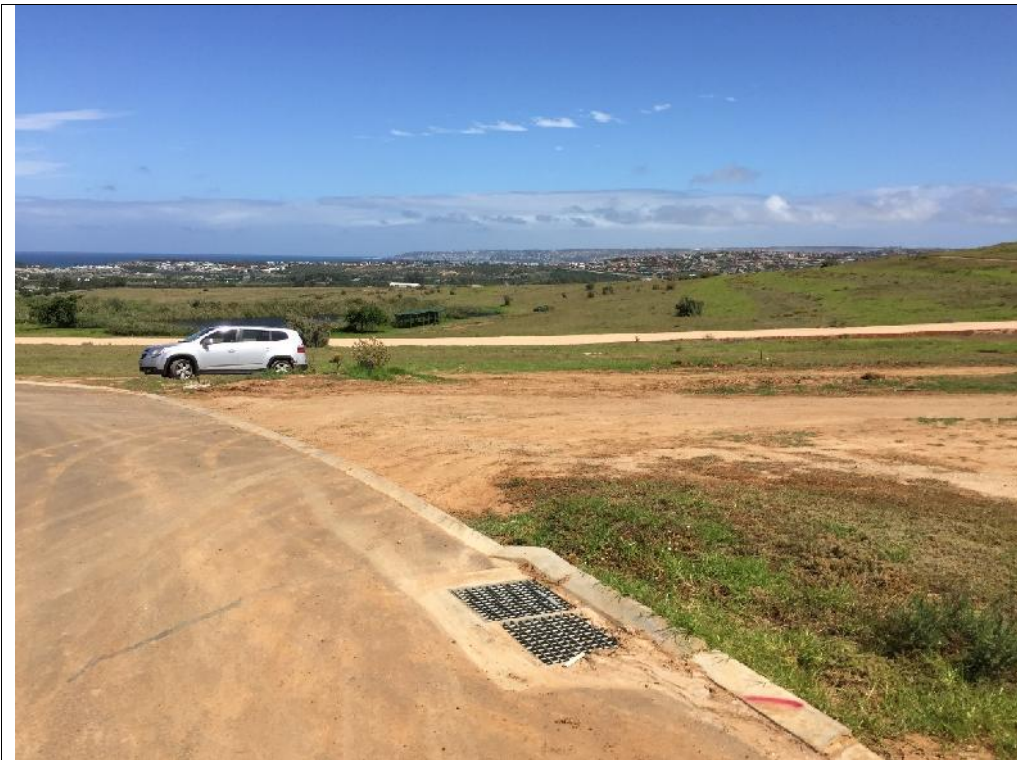
Temporary access road during the surfacing of the main access road.
