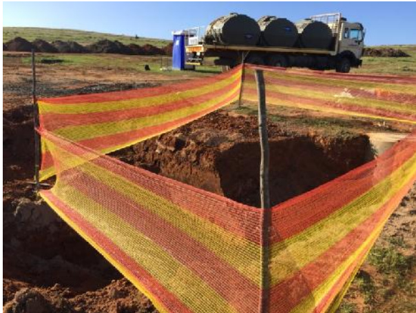
Open trenches were demarcated appropriately.
