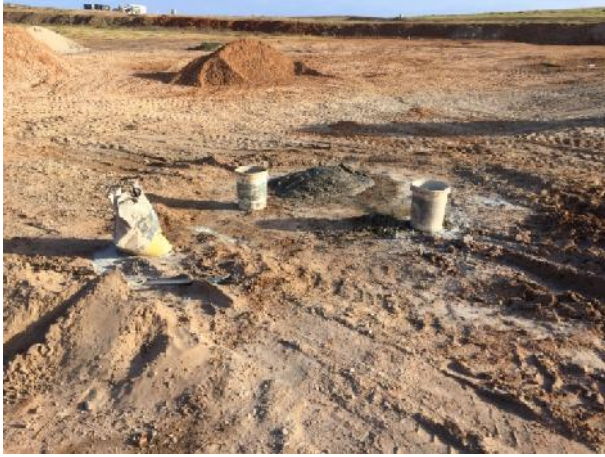
Civil contractor – limited cement mixing was necessary and was done in a central location. The area was rehabilitated.
