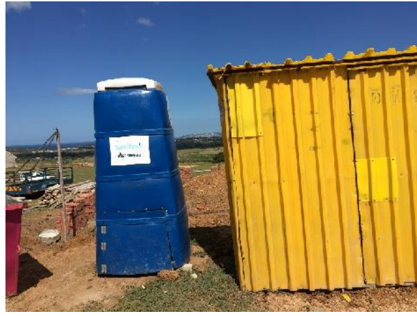
Individual home builder provide portable chemical toilets for staff during construction phase
