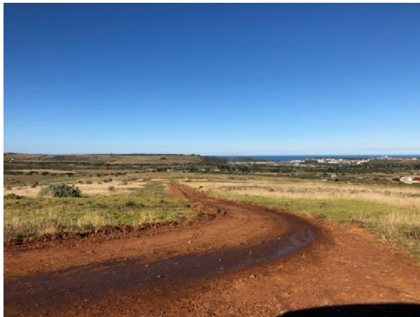
Water truck spraying water on haul roads.
