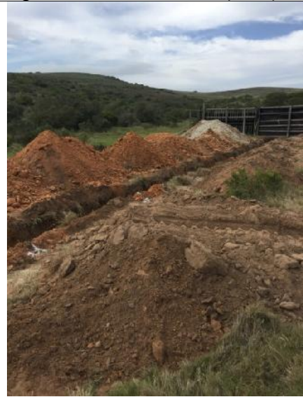
2021.03.24 – The construction of civis at phase 10 is ongoing and remains within the dedicated work zone.
