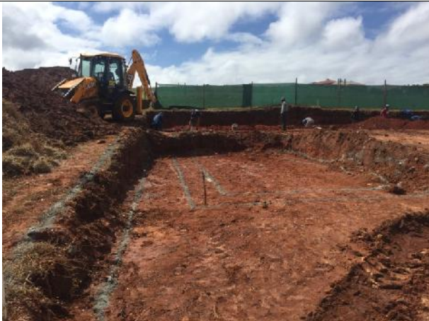
2021.03.17 - Individual house construction started on Erf 6635
