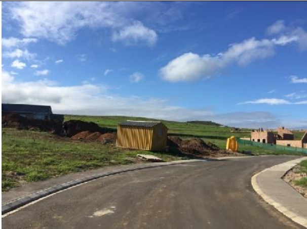
2021.04.28 – House construction started on Erf 6563. Environmental induction must be done as soon as possible.
