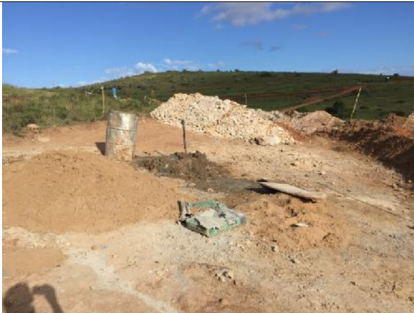
2021.04.28 – Phase 10 cement mixing area is within the proposed tar road section.
