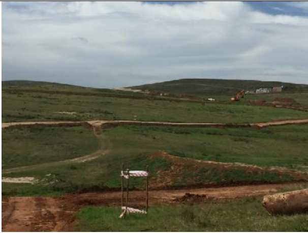
2021.03.24 – Construction of the road in Phase 10 have commenced
