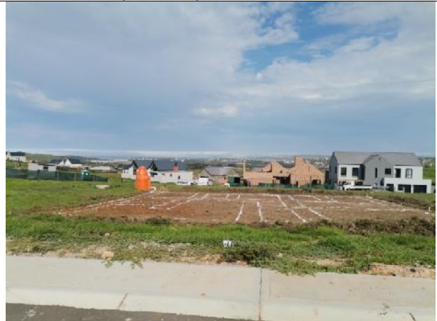
2021.04.21 – House construction started on Erf 6592. Environmental induction must be done as soon as possible.
