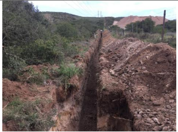
2021.03.24 – Trenches are to be demarcated according to Health and Safety requirements.
