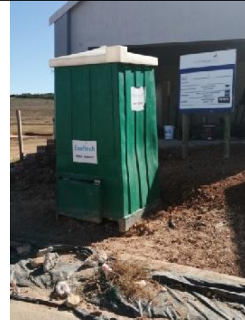
2021.02.17 - Individual home builder provide portable chemical toilets for staff during construction phase (Erf 6557)
