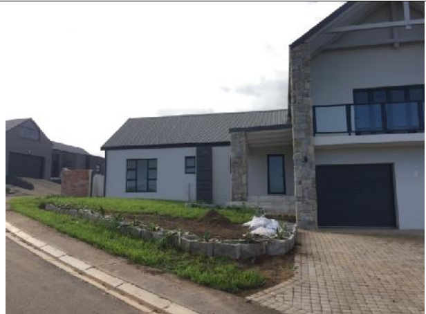
2021.04.28 - Individual house construction nearly done (Erf 6644)
