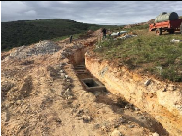
2021.04.28 – The construction of civis at phase 10 is ongoing and remains within the dedicated work zone.
