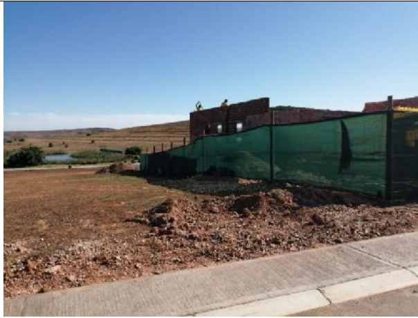
2021.02.17 - Erf 6549 - No-Go demarcation indicating the work zone.
