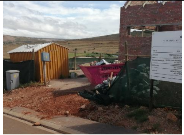
2021.03.10 - Individual home builders provide a suitable skip or bins on site (Erf 6631).
