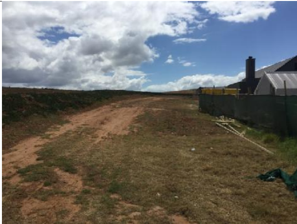
2021.02.24 - Temporary access road behind Erf 6558 must be demarcated and rehabilitated.
