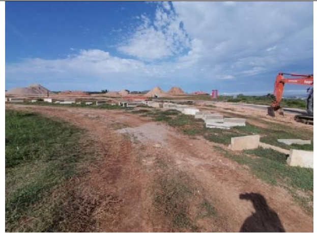
2021.04.21 – The phase 3 contractor removed the Port Jackson ( Acacia saligna ) when they started with the road maintenance.
