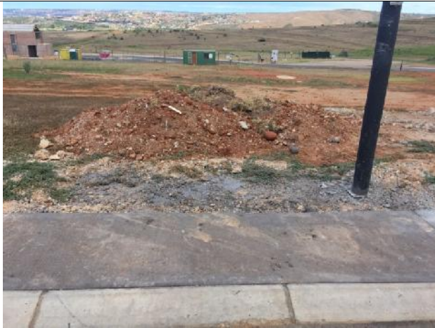
2021.02.24 - Sidewalk construction area must be cleared and rehabilitated.
