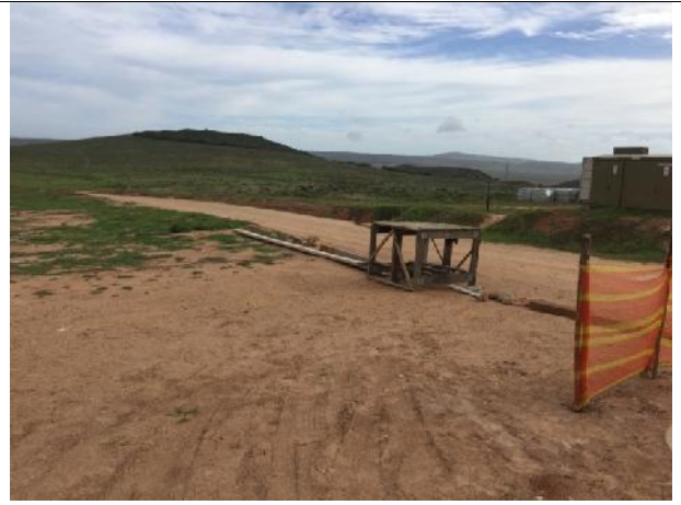
2021.03.24 – The 'temporary access road' located through the open space and Erf 6545 has been closed off. The compacted area must be ripped and rehabilitated with indigenous grass seed mixture sown over a lightly raked area (and watered).
