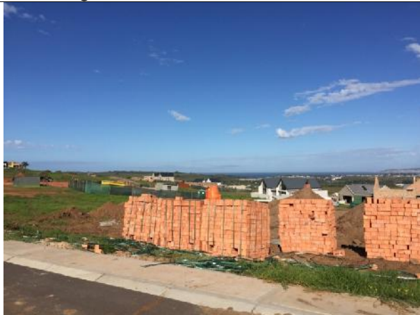
2021.04.28 - Erf 6593 - No-Go demarcation must still be installed.
