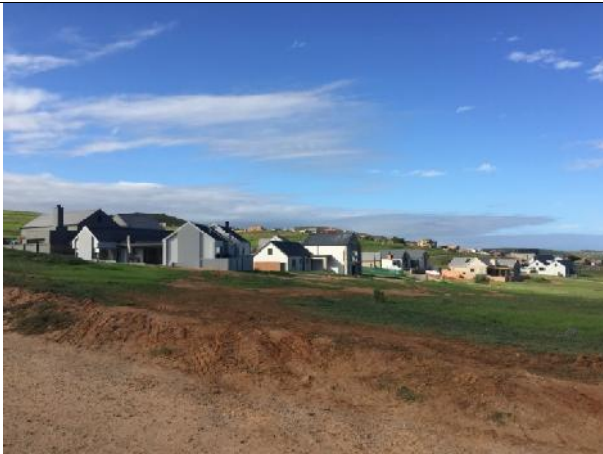
2021.04.28 - The temporary access road across the open space behind Erf 6557 MUST be closed off and rehabilitated.
