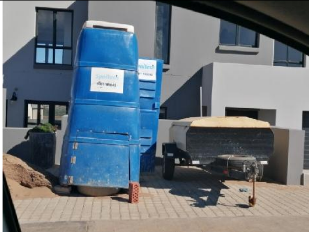
2021.02.17 - Individual home builder provide portable chemical toilets for staff during construction phase (Erf 6619)
