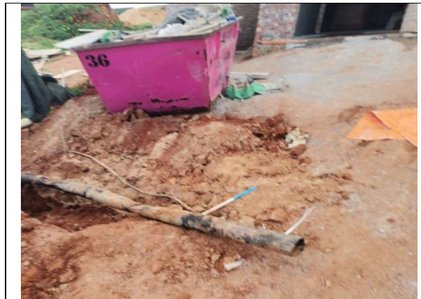
2021.06.23 - Individual home builders provide a suitable skip or bins on site (Erf 6631) – skips/bins must be covered to prevent the windblown litter from blowing away in the wind.
