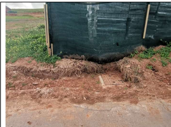
2021.06.23 – Erf 6637 - No-Go demarcation indicating the work zone – civil contractor was busy with remedial repairs to water pipelines.
