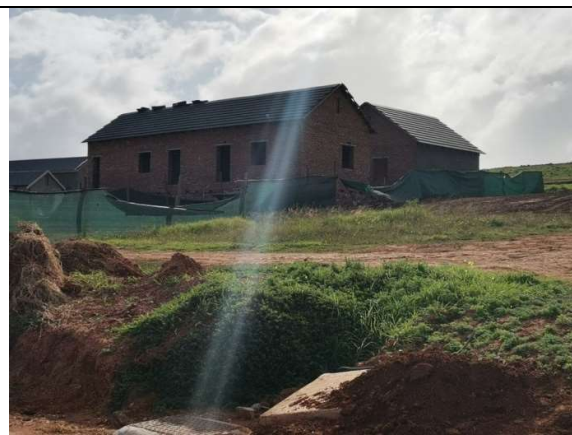
2021.06.23 – Erf 6566 – Contractors need to maintain the No-Go demarcation, especially during inactive periods (weekends & outside working hours).
