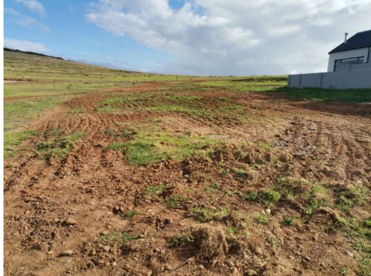
2021.06.23 – Temporary access roads across Erf 6556 have been closed off and the area was rehabilitated.
