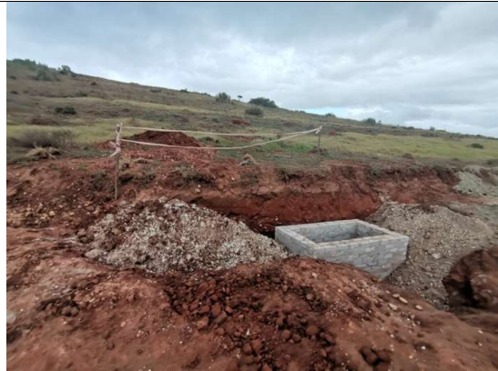
2021.06.23 – Trenches are to be demarcated according to Health and Safety requirements.
