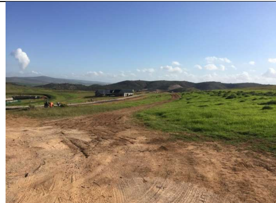
2021.06.09 – All temporary access roads MUST be closed off and rehabilitated.
