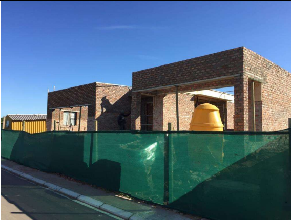
2021.06.04 – Unit construction sites with portable chemical toilets for staff.
