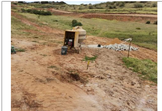
2021.07.28 – Stand mixers are used - a non-permeable layer must be used underneath the concrete mixer, or suitable settling ponds and trapping mechanisms to be implemented – all disturbed areas must be rehabilitated.
