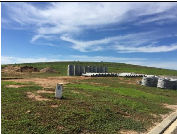
2021.04.07 – The construction material storage area was located in a future development zone
