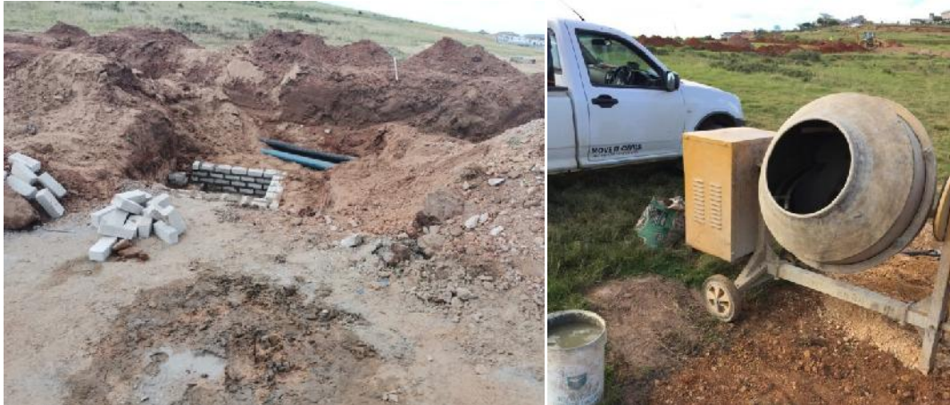
2021.06.23 – The cement mixing area was within the proposed surfaced road section and no contaminated soil was noticed (photo taken June 2021).
