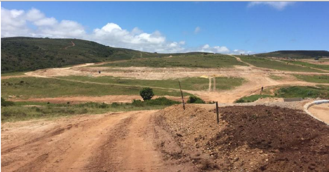
2021.12.09 – Temporary haul route during the construction of the main access road to Phase 10 (photo taken in December 2021)
