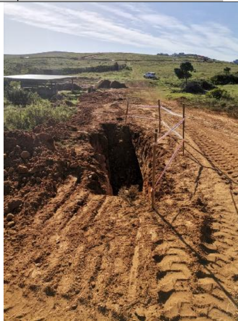
2021.03.31 – No-Go demarcation for deep excavations
