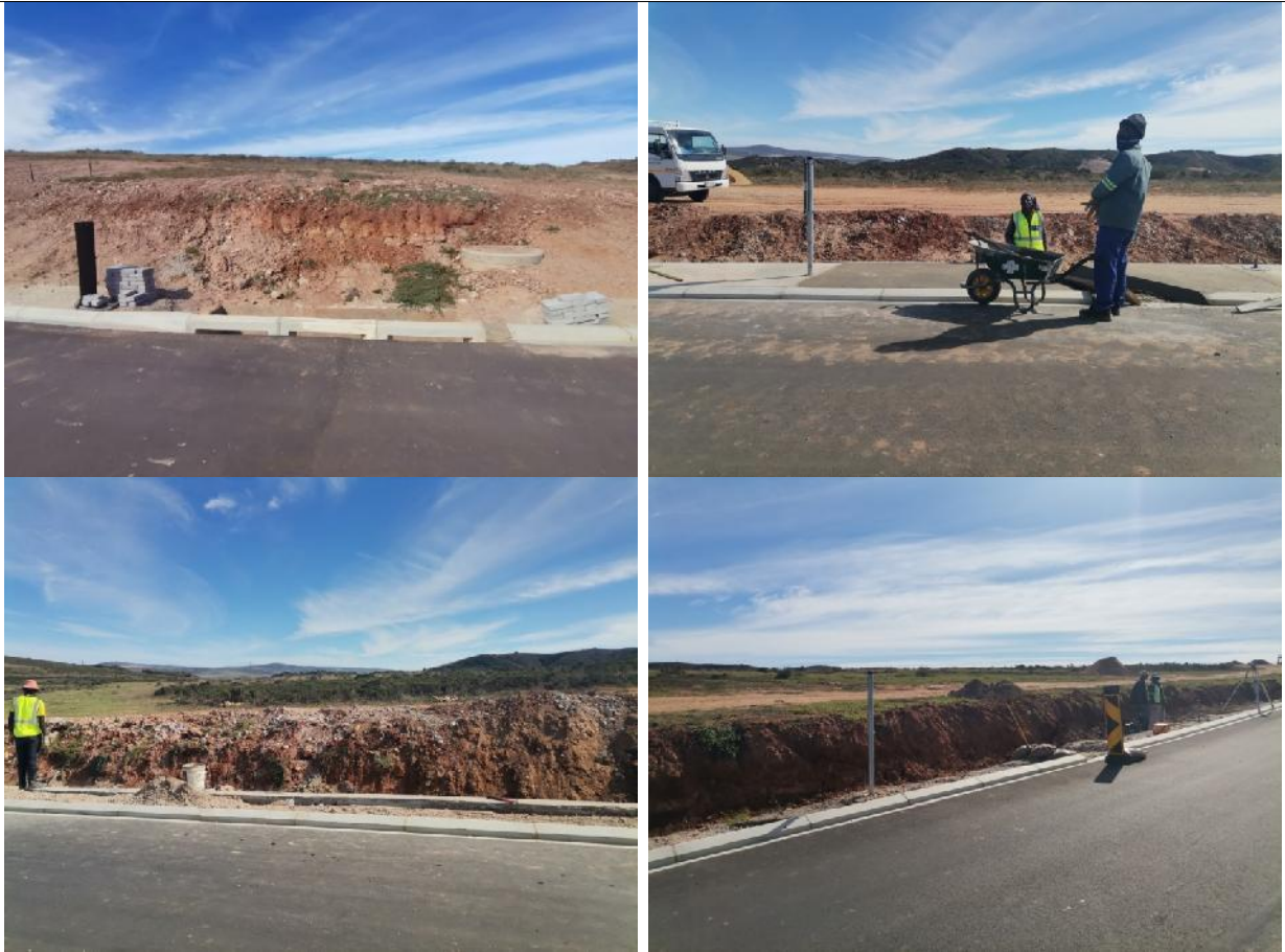
2022.04.20 – Progress with the construction of the stormwater channel of Mafunyane Street (photo taken April 2022)
