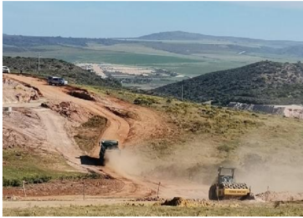
2021.09.08 – Water was sprayed on the roads to minimize the dust (photo taken September 2021).
