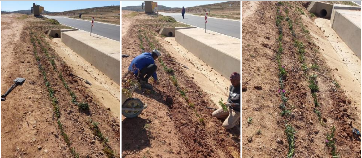
2022.09.08 - The rescued plants being planted on the embankment next to the stormwater outlet.
