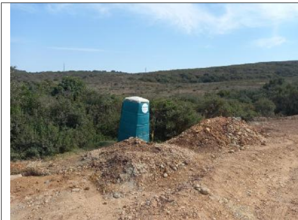
2022.09.15 – Ablution facilities are available to staff installing civil services.
