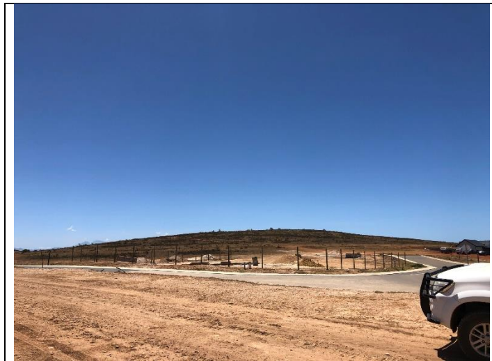
Main civil contractor – busy installing demarcation/fence around the cement mixing area.
