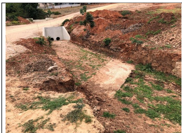
Silt fence will be installed as soon as the final shaping is done
