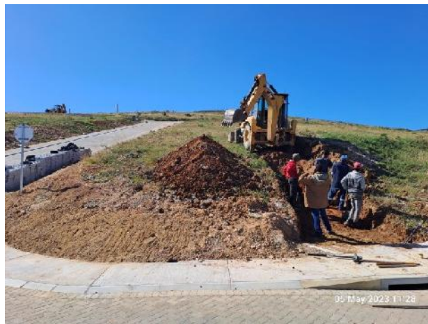
5 May 2023 – contractor busy installing grass blocks in the stormwater channel (phase 11).
