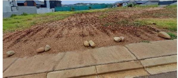
(2023.05.12) – Erven that were disturbed during house construction ( phase 2 ) have been rehabilitated.
