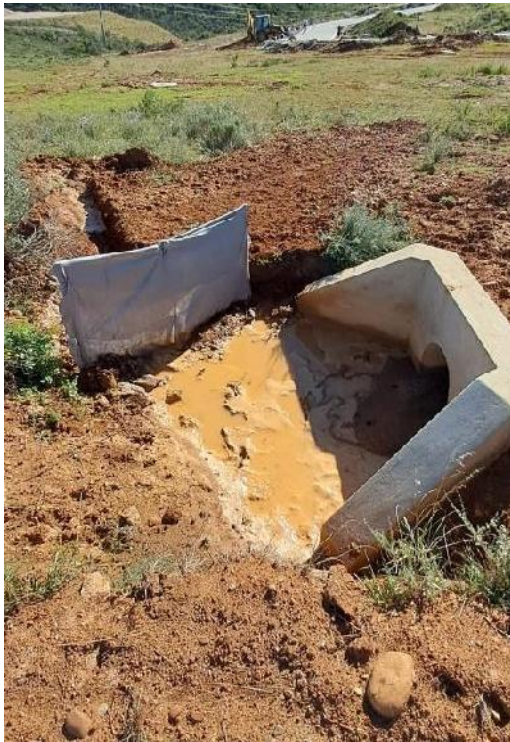
(2023.05.23) – Silt fences at stormwater outlets in phases 4, 12 and 14 proved to be effective (provided that they are cleaned after rain spell)
