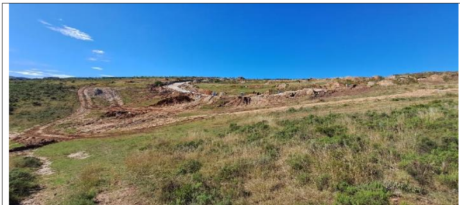
General view of the construction site – Phase 12
