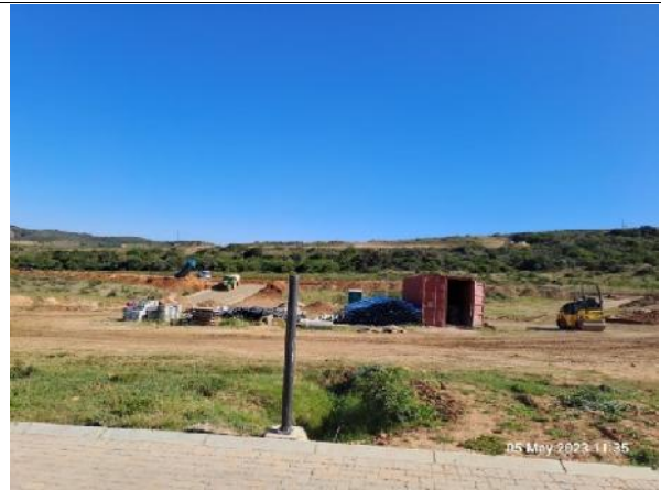
(2023.05.05) – General view of site camp at phase 12 with included ablution facility.
