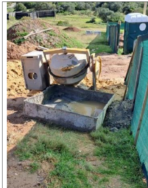
(2023.06.09) – Bunding for cement mixing in place (note that it is required that all construction activities be confined to the demarcated housing construction zone).
