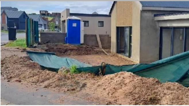
(2023.06.09) – Evidence of ablution facility at individual housing construction (note the green net was temporary removed to work on HOA infrastructure).
