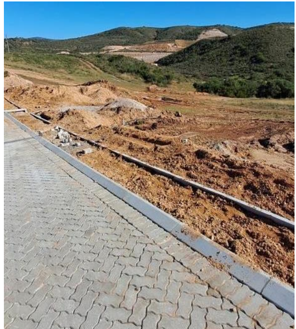
(2023.05.23) – Once the main road and sides/walkways are completed, then the road verges will be rehabilitated (phase 4) .
