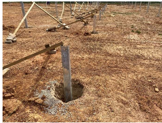
Footings in place awaiting concrete fillings.
