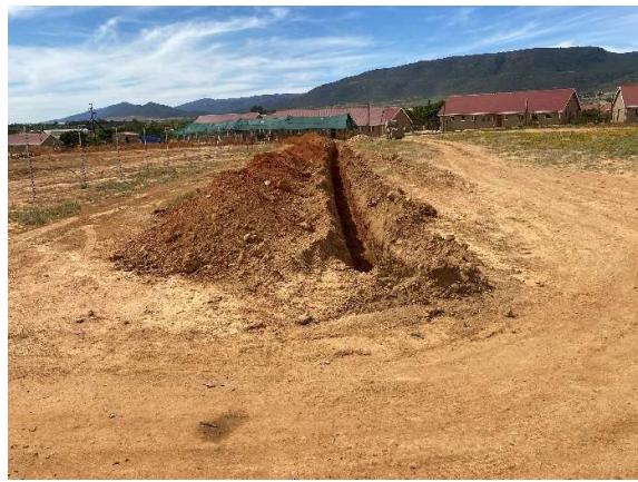
Excavated trenches for implementing groundwater control measures.
