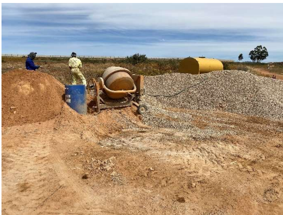
Cement batching active for the construction of the solar panel footings and control stations.
