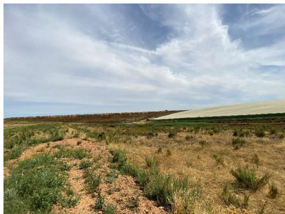
Towards the west of the development seen towards the south showing the condition of the no-go area.
