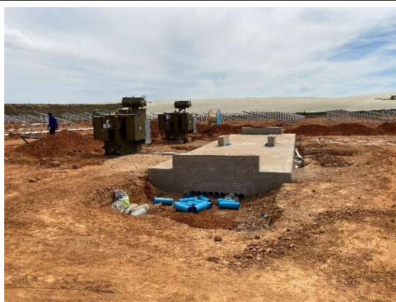
Control station substructure being constructed.
