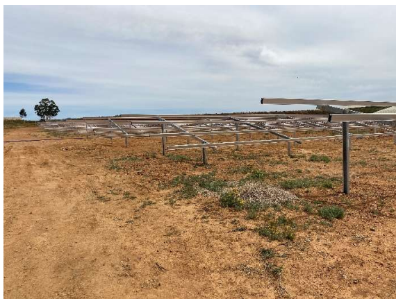
Condition of the newly installed solar panel footings and frame structures.
