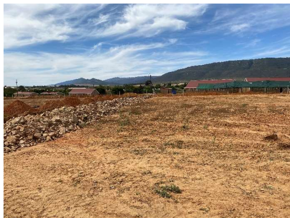
Condition of the site seen towards the north with a channel being lined with rocks for groundwater control.
