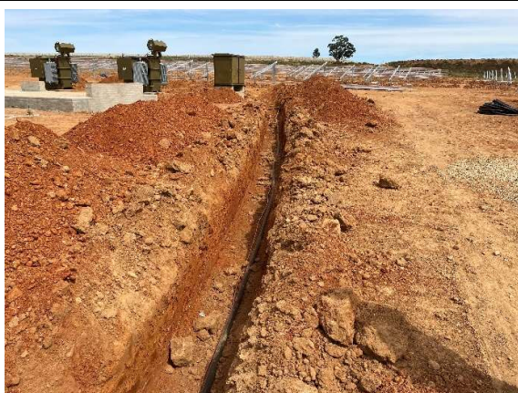
Excavated trench for the installation of electrical distribution cables.
