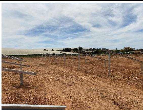
Condition of the newly installed solar panel footing and frame structures as seen towards the west.
