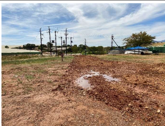
Completed and covered trenches of power cables leading towards the ring main unit and distribution network.
