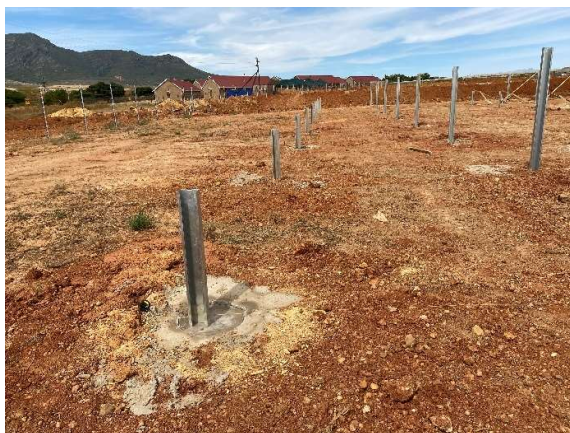
Concrete cast footings in place. Dry concrete remains are removed once concrete has set.
