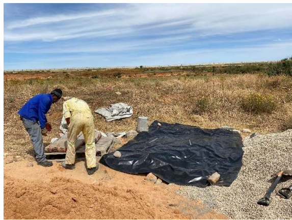
Impermeable builders plastic sheeting used during cement batching.
