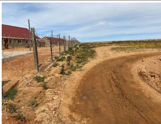
Watering of gravel access roads on site towards the northern boundary.
