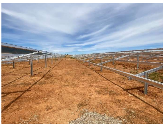
Completed panel footing and frame structures as seen towards the east.
