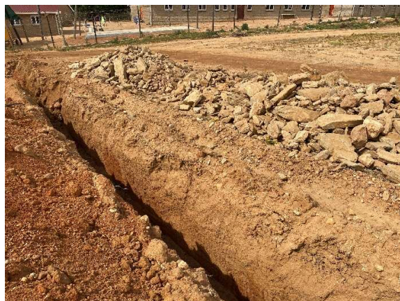
Excavated trenches towards the middle of the site where rocks and pipelines are installed for groundwater control.
