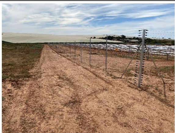
Along the southern boundary (outside) of the development footprint as seen towards the west.
