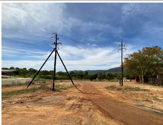
Watering of gravel access roads on site towards the northwestern corner.
