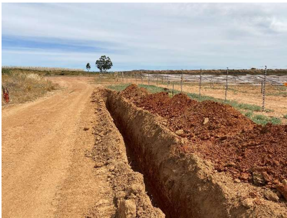
Excavated trenches for implementing groundwater control measures.
