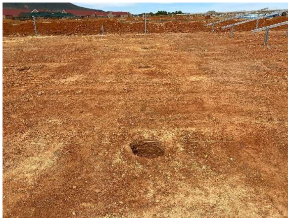
Excavated holes for the placement of the solar panel footing structures.
