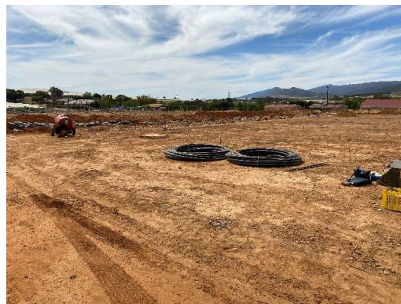
The condition of the site with water pipelines to be installed and utilized for washing of the panels.
