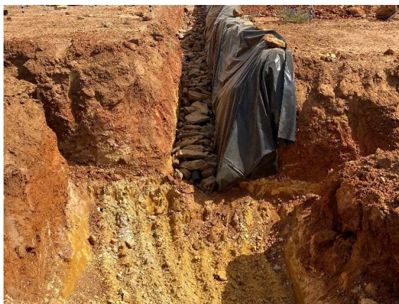
Excavated trenches towards the middle of the site where rocks and pipelines are installed for groundwater control.
