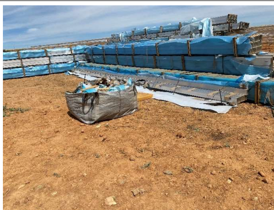
Structural material stored on-site with a bag for plastic storage.
