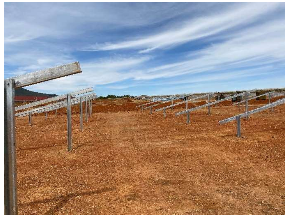
Condition of the newly installed solar panel footing and frame structures as seen towards the east.
