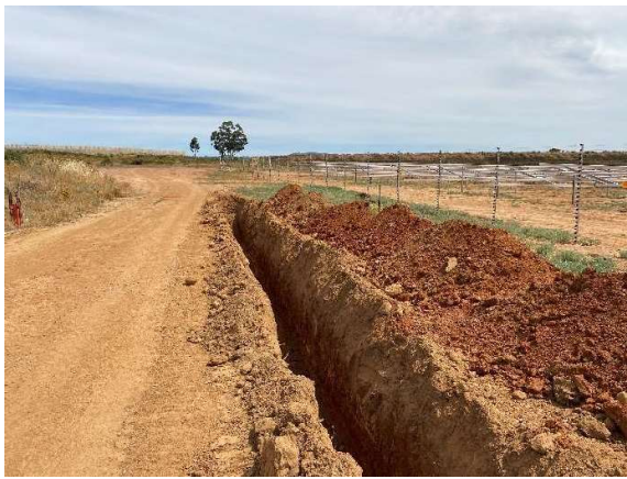
Excavated trenches for implimenting groundwater control measures.
