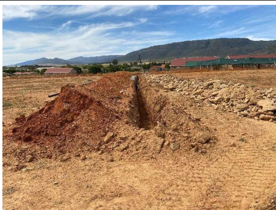
Excavated trenches towards the middle of the site where rocks are utilized for assisting with groundwater control.
