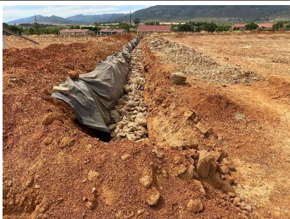
Excavated trenches towards the middle of the site where rocks are utilized for assisting with groundwater control.
