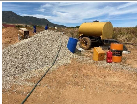
Water truck available for dust suppression.
