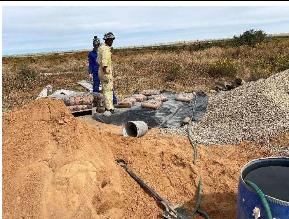
Impermeable builders plastic sheeting used during cement batching.
