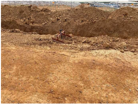
A rotating sprayer on site for dust suppression.
