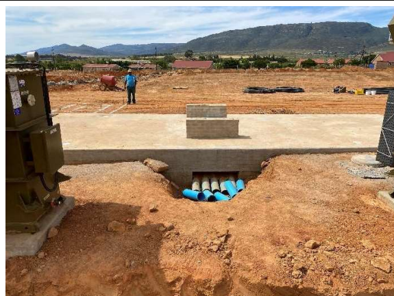
Electrical control station substructure.
