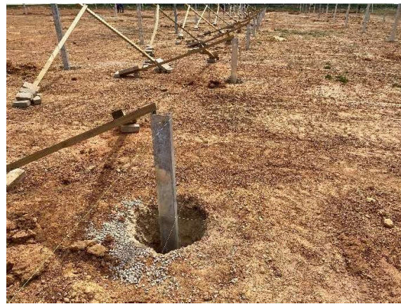
Footings in place awaiting concrete fillings.
