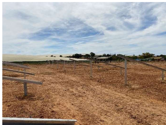
Condition of the newly installed solar panel footing and frame structures as seen towards the west.
