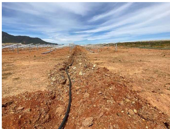
Excavated trenches where water pipelines have been installed for the washing of the panels.
