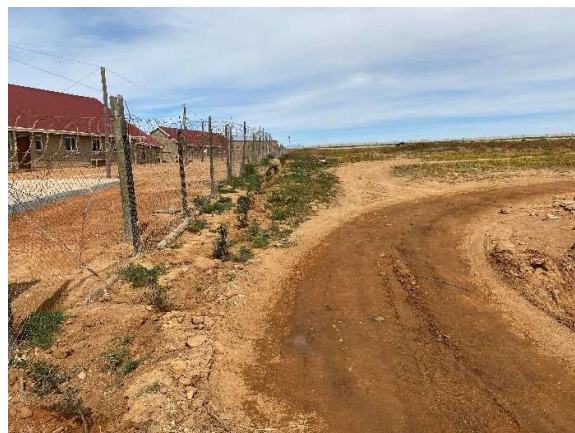
Watering of gravel access roads on site towards the northern boundary.
