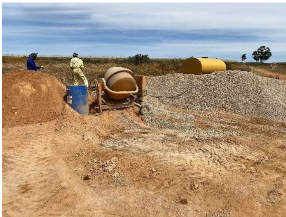
Cement batching active for the construction of the solar panel footings and control stations.
