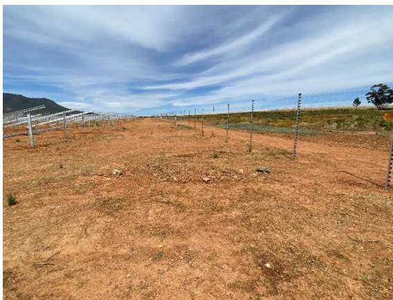
Along the southern boundary (within) of the development footprint as seen towards the east.
