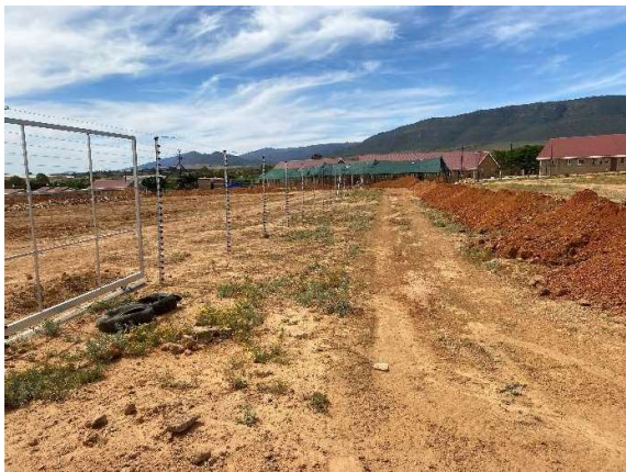
Eastern boundary of the development footprint with security fencing installed seen towards the north.
