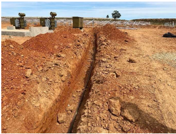
Excavated trench for the installation of electrical distribution cables.
