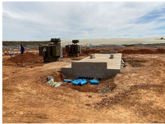
Control station substructure being constructed.
