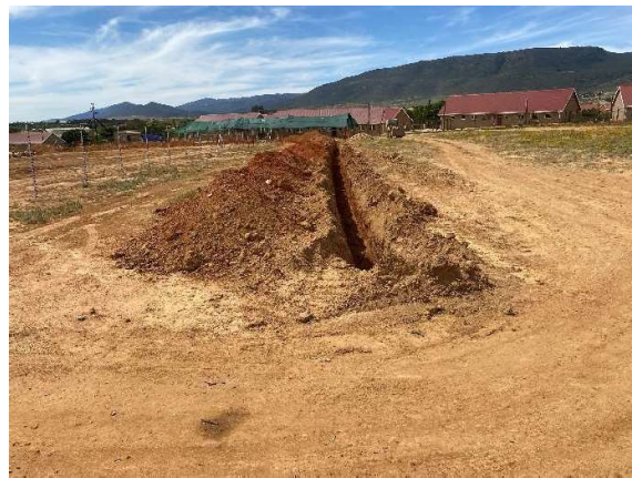
Excavated trenches for implimenting groundwater control measures.
