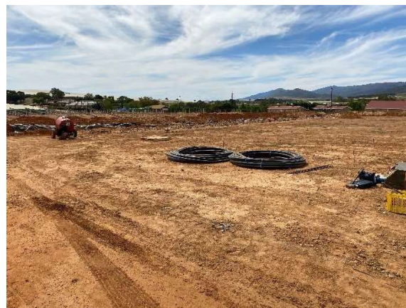
The condition of the site with water pipelines to be installed and utilized for washing of the panels.
