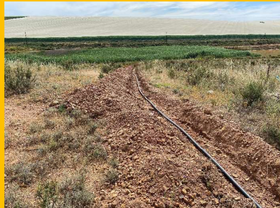
A water pipeline connecting to an existing pipeline within the no-go area, although outside the wetland boundary.
