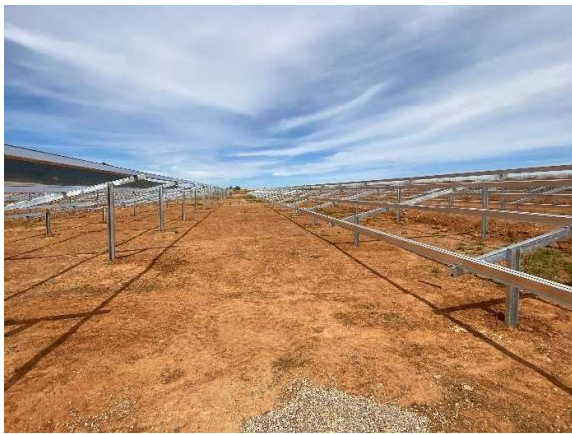
Completed panel footing and frame structures as seen towards the east.
