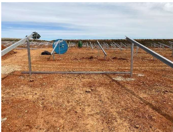
Condition of the newly installed solar panel footing and frame structures as seen towards the south.
