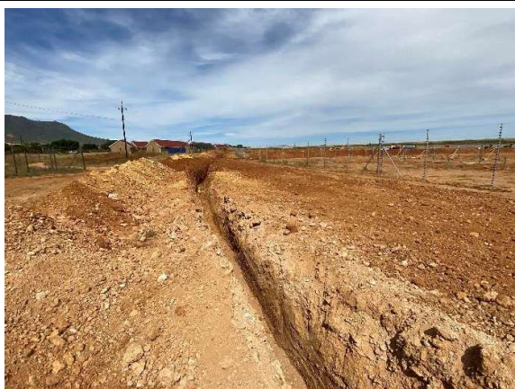
Groundwater cutt-off trenches along the northern boundary conveying groundwater towards the west.
