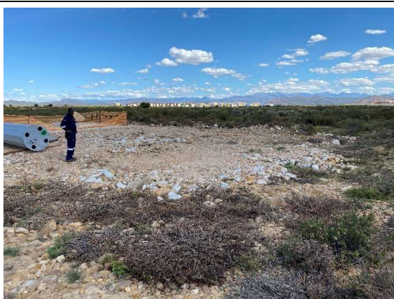
Completed footing and backfill at pylon location 17 as seen towards the southeast.
