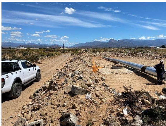
From pylon 8 as seen towards the south showing the derelict condition of this specific area.
