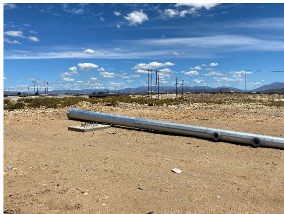
Pylon 9 on site adjacent to the footing as seen towards the south towards Raymond Pollet Drive.
