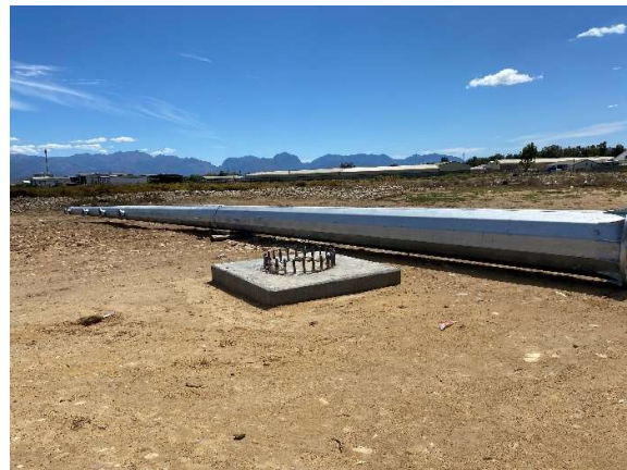
From pylon 10 footing as seen towards the west towards the Worcester industrial area off Maritz Street.
