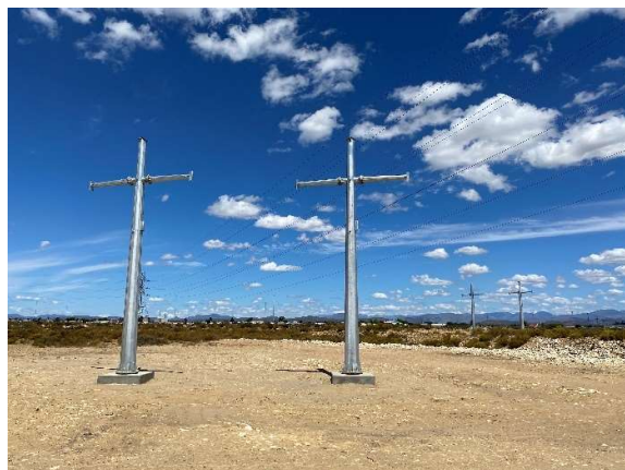
Two pylons erected at location 6, as seen southeast towards pylon location 7 in the back of picture.
