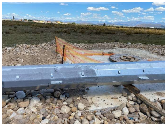
Completed footing and backfill at pylon location 13 as seen towards the southeast toward the Hex River.
