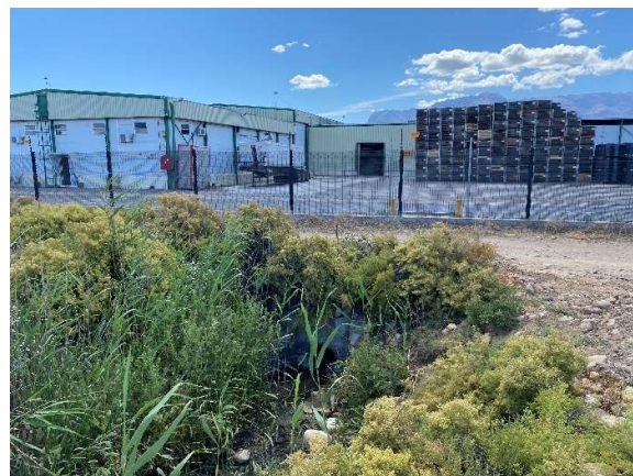
Stormwater outlets from the industrial area adjacent to Ceres near pylon 11.
