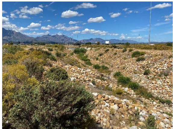
Existing stormwater drainage channel immediately north of Robertson Road (R60).
