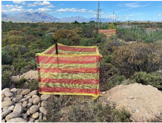
Test hole excavations along the route between pylons 18 and 21 sufficiently demarcated and limited.
