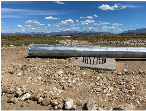
Completed footing and backfill at pylon location 14 as seen towards the southeast toward the Hex River.
