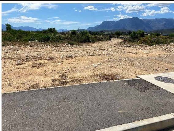
Short service access road created to pylon 16 from the Transhex main (tar) access road.
