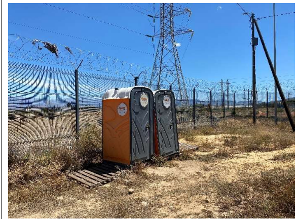
Chemical toilets in places within the Worcester Industrial substation.
