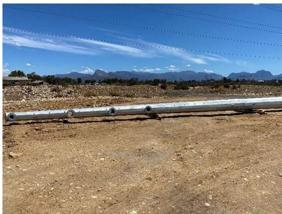
Pylon 5 per Figure 3 which has been placed on site at its completed footing.
