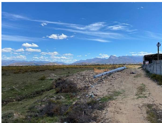
Completed footing and backfill at pylon location 13 immediately southeast of Carr Street.
