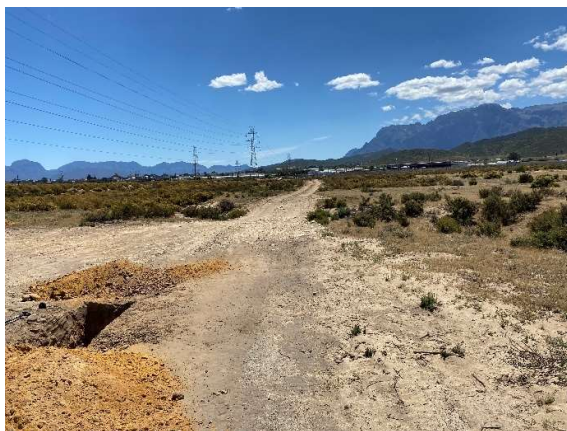
Test hole near pylon 6 as seen towards the west along the existing Eskom service road.
