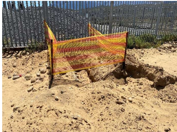
Excavations for future lines, appropriately demarcated.
