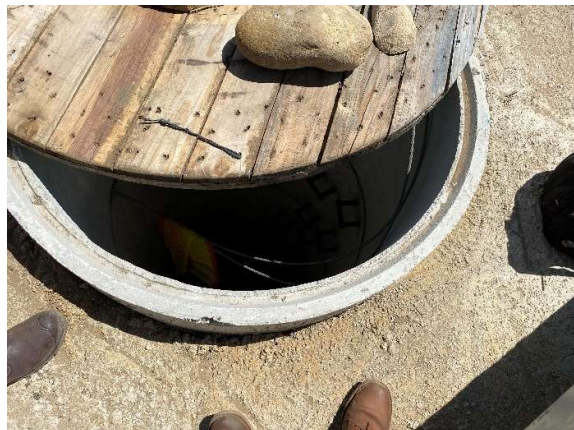
Manhole at pylon 5.
