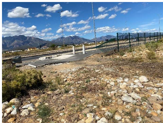
Temporary access from south of Robertson Road (R60).
