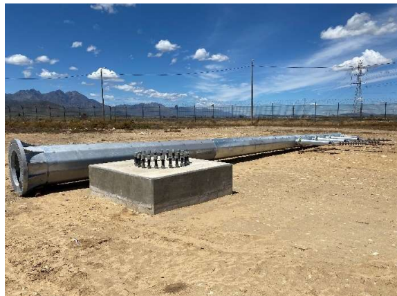
Constructed pylon footing and pylon 1 next to it within the Worcester Industrial Substation.
