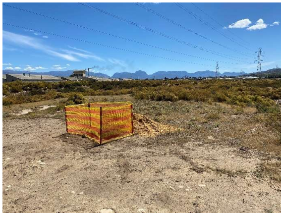
Test holes along the route near pylon 5, sufficiently demarcated.
