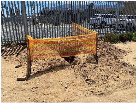
Excavations for future lines, appropriately demarcated.
