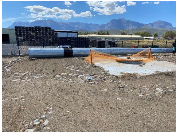
Completed casting and backfill of the pylon at location 12 along the industrial boundary (immediately east).
