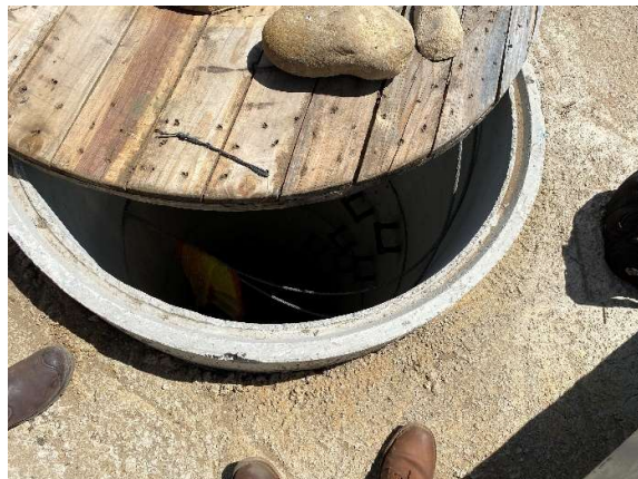
Manhole at pylon 5.
