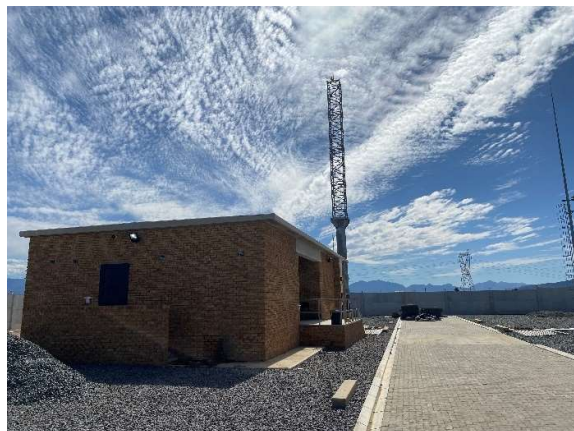
Within Transhex substation.
