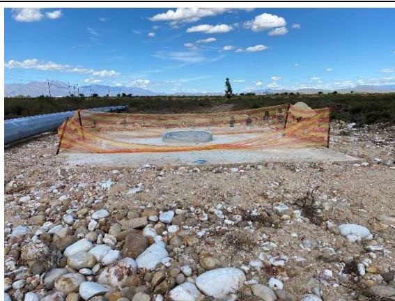
Completed footing and backfill at pylon location 17 as seen towards the east.
