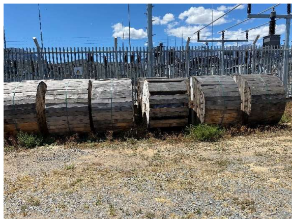
Electrical cable drums within the contractors camp at the Worcester Industrial Substation.
