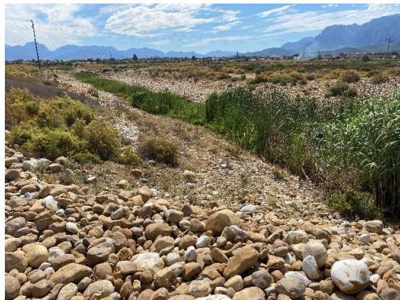
Existing excavated stormwater drainage channel from the Transhex development seen towards the southwest.
