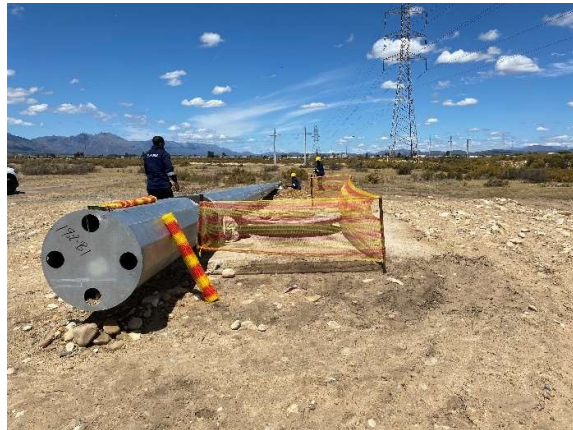
Pylon 5 per Figure 3 which has been placed on site at its completed footing.
