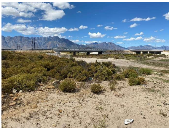
East of pylon 10 seen towards the north towards Raymond Pollet Drive bridge showing the Hex River.
