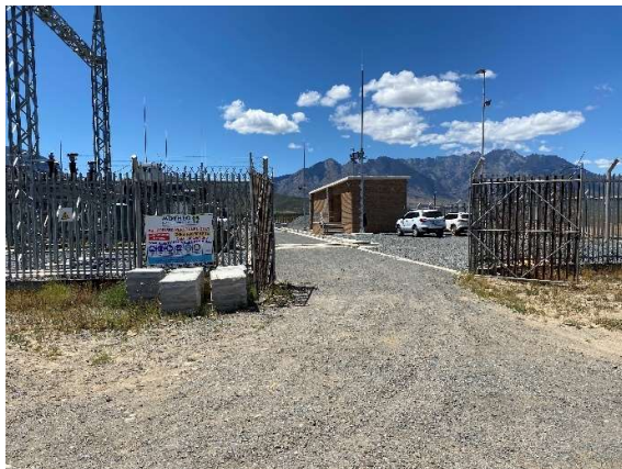
Worcester Industrial Substation internal gate.
