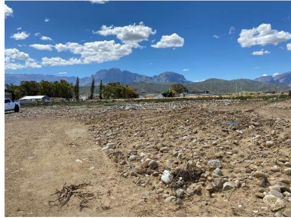
From pylon 10 footing seen towards the north towards Raymond Pollet Drive.
