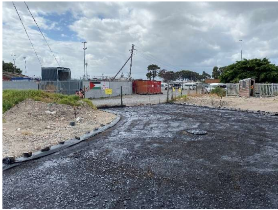
The newly surfaced road at the southeastern corner of the site connecting to Ngqwangi Drive.
