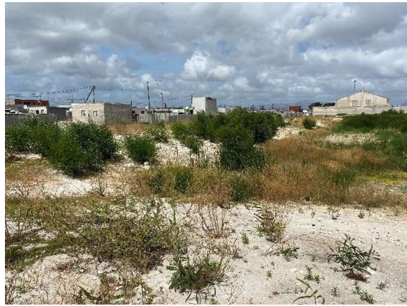
Current condition of the stormwater detention pond with some bullrush and acacia shrubs.
