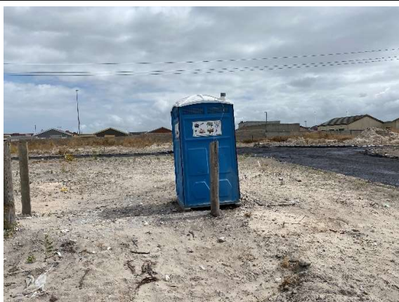
Chemical toilet in place adjacent the current works and secured to the ground.
