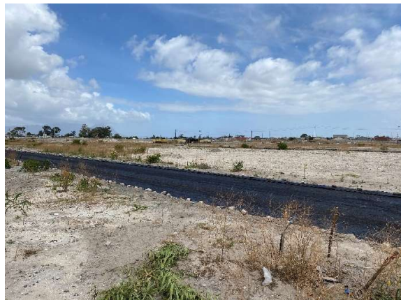
Along the south boundary of the site, as seen across the site towards the northwestern corner of the site.
