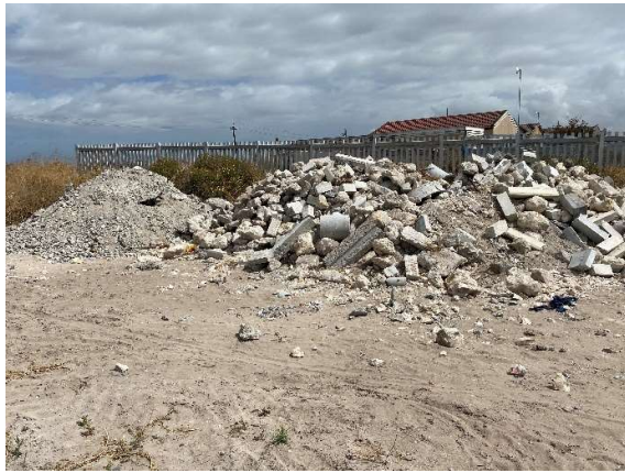
Building rubble temporarily stockpiled near the construction entrance.
