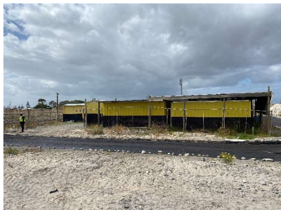
View of the contractors site offices and storage containers areas within the future public space area.
