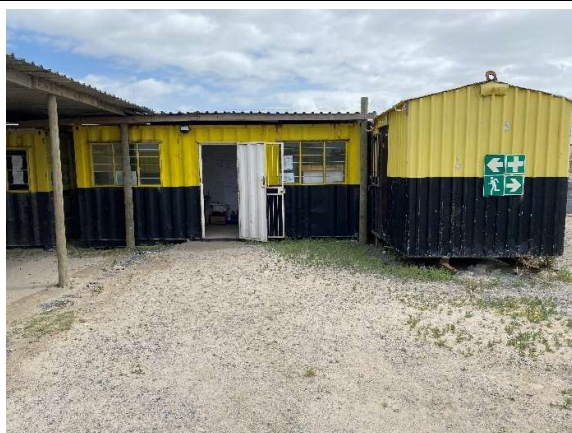
The contractors site offices located in the centre of the development footprint at the future public open space.
