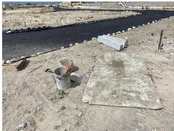
Kerbs being installed within the development footprint. A mixing board in place for the kerb mix.
