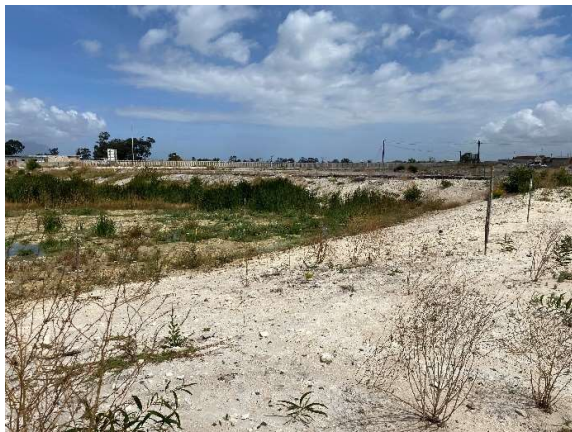
Current condition of the stormwater detention pond with demarcation stakes in place along the eastern bank.
