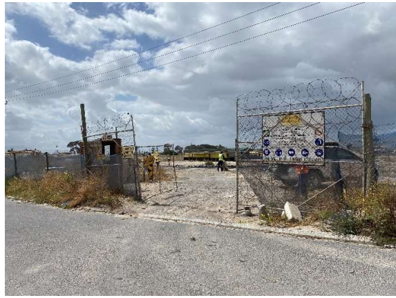
Existing construction access off Gcubane Road with the required safety and construction signage on the gates.
