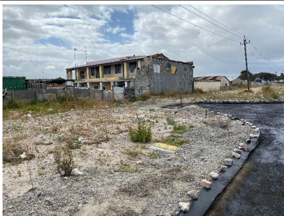
Condition of the site along the eastern boundary of the site as seen towards the south.
