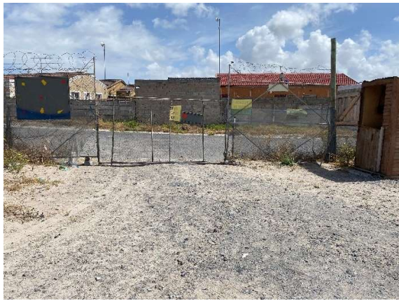
Entrance to the site securely closed off to the public during construction.
