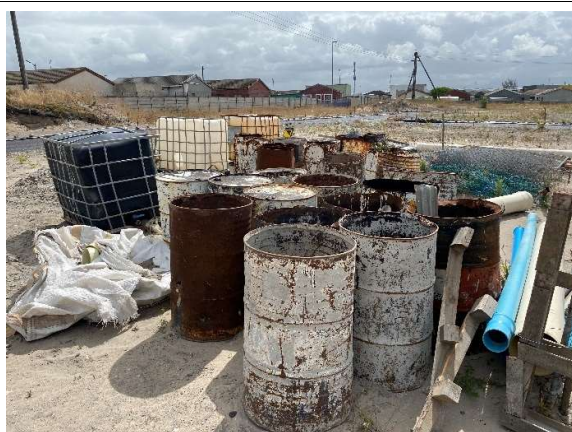
Empty bitumen drums and flowbins for water storage in place at the material laydown area.
