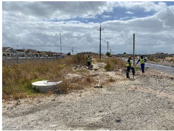
Stormwater manholes installed towards the northern boundary of the site.
