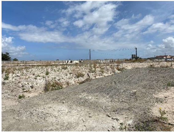
The condition of the northwestern section of the site, as seen towards the northwestern corner.
