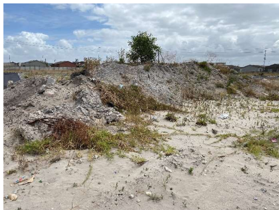
Excavated soils and builders rubble stockpiles behind the material laydown area.
