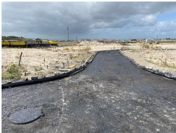
Newly surfaced internal road within the development where a service manhole can also be seen.
