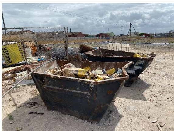
Waste skips in place at the laydown area. Proof of disposal slips are available in the environmental file.
