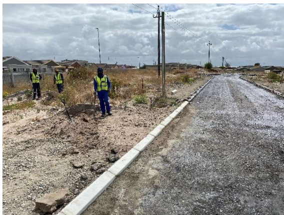
Kerbs being installed near the northern boundary and the temporary construction access.
