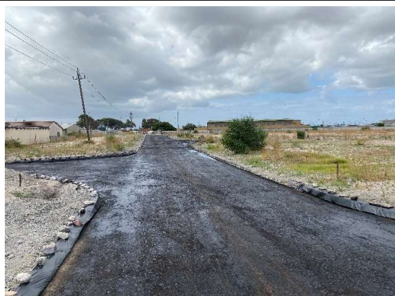
Condition of the newly surfaced road along the eastern boundary seen towards the south.
