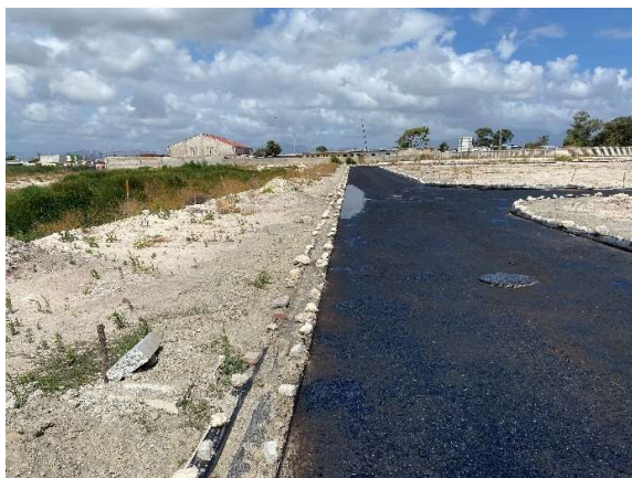
The stormwater detention pond along the internal road leading immediately north as seen towards the west.
