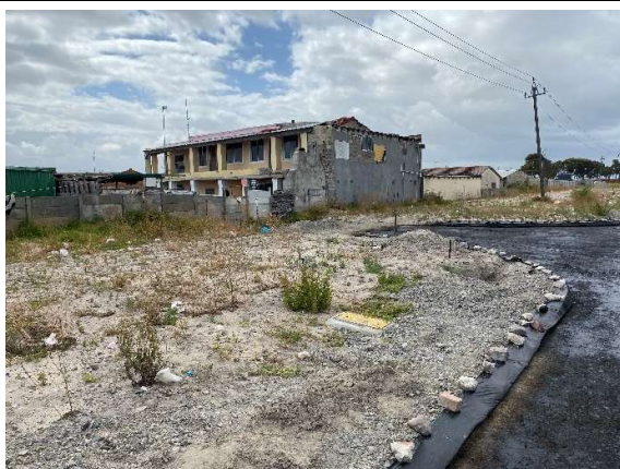
Condition of the site along the eastern boundary of the site as seen towards the south.
