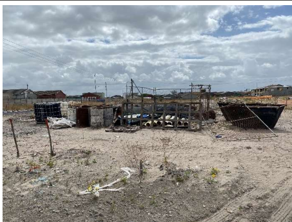
Temporary laydown area immediately east of the contractors camp with temporary fencing.
