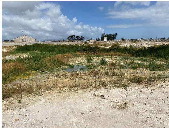
Current condition of the stormwater detention pond with stakes in place.
