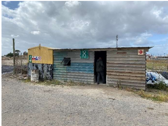
Contractors camp and eating area also serving as the emergency assembly point.
