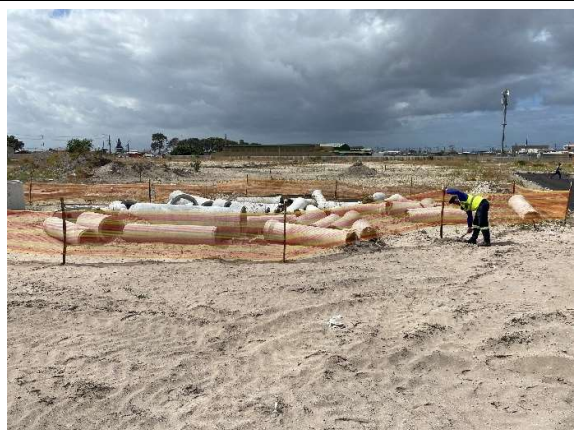
Material laydown area sufficiently demarcated with orange netting in place.
