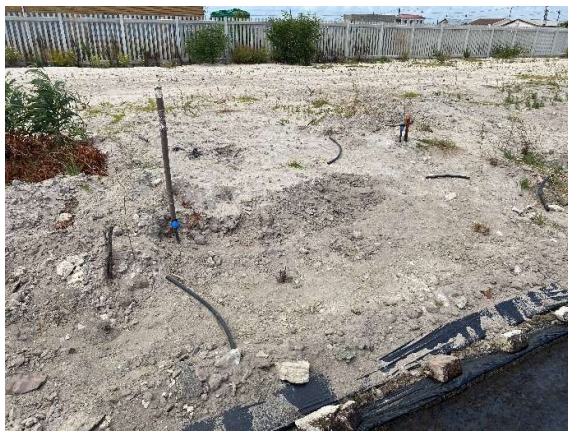
Condition of the civil services connection points completed along the internal roads.
