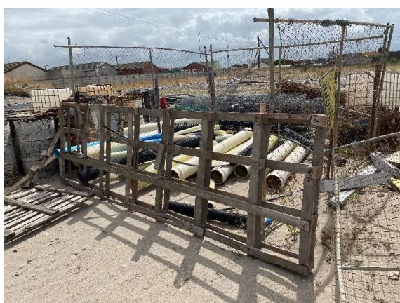
Temporary material laydown area, with material fenced in.
