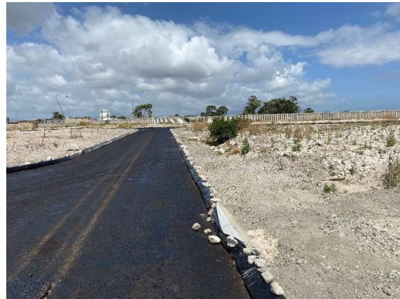
Condition of the completed internal road and kerbs as seen towards Sheffield Road in back of picture.
