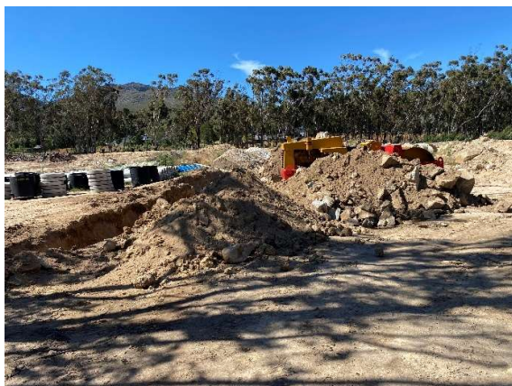
Excavated material and rubble stockpiles near the entrance to the site to be removed.
