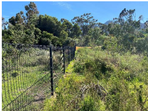
Condition of the northern boundary of the site with the fence line in place seen towards the east.
