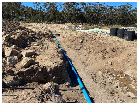
Installation of potable water pipelines along the centre-eastern section of the site.
