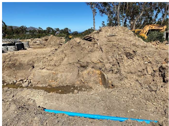
Installation of potable water pipelines along the centre-eastern section of the site. Also note the broken rock.
