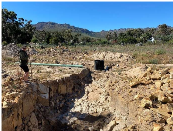
The installation of sewer and stormwater services along the western end of the development footprint.
