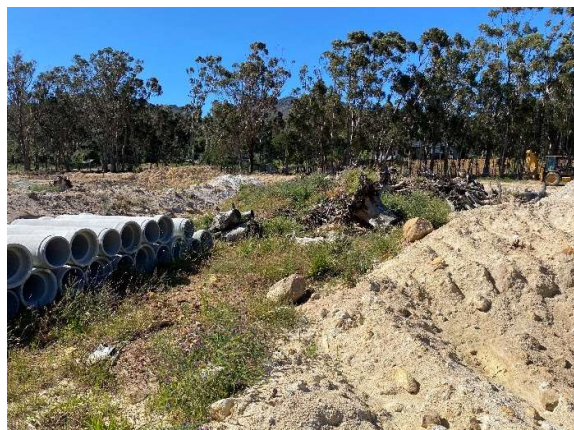
Temporarily stockpiled stormwater pipelines near the eastern centre of the site seen towards the southeast.
