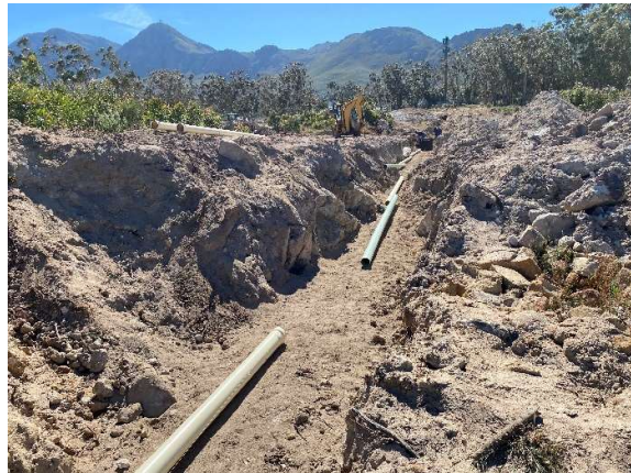
Sewer pipes being installed along the southern portion of the site as seen towards the east.
