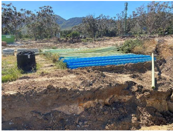
Sewer and water pipes at the current material laydown area along the eastern portion of the site.
