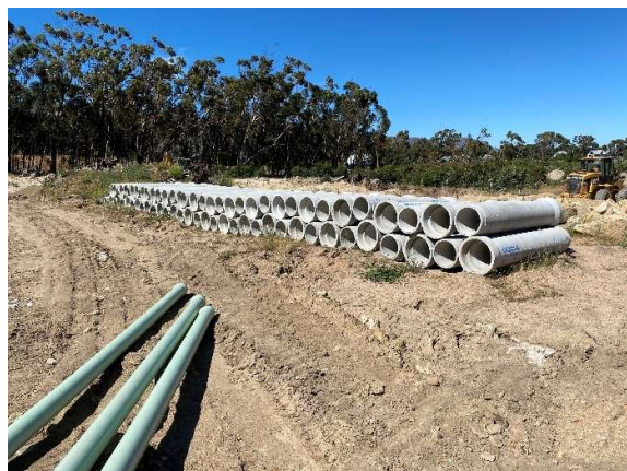
Temporarily stockpiled stormwater pipelines near the eastern centre of the site seen towards the south.
