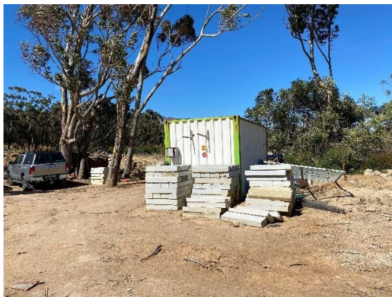
Contractors site office container.
