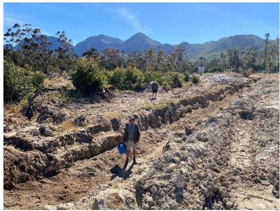
Installed sections of sewer pipelines along the southeastern section of the site.
