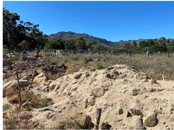
Installation of bulk services underway just towards the west of the conservation area.
