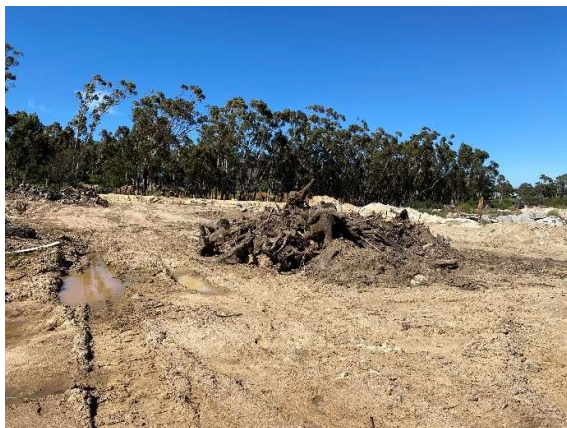
Felled Blue Gum trees (cleared vegetation) temporarily stockpiled on site.
