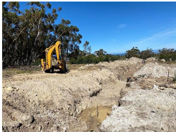
Installation of sewer pipes along the centre of the site as seen towards the west.
