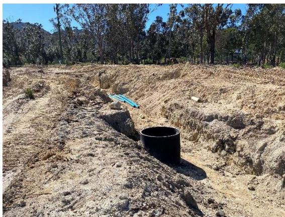
Installation of sewer, and potable water services as seen towards the east.
