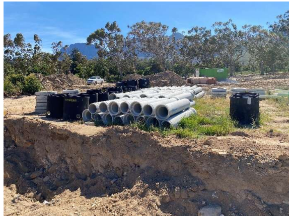
Stormwater pipes at the current material laydown area along the eastern portion of the site.
