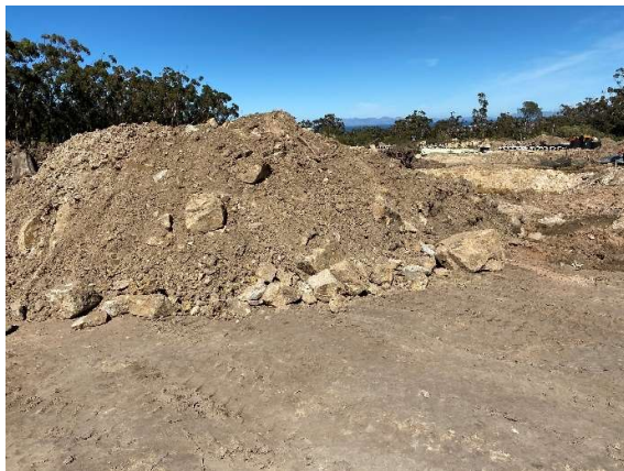
Excavated soil stockpiles on-site containing some broken rocks.
