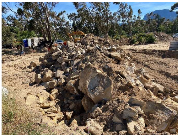
Soil and rock stockpiles present along the laydown area near the eastern centre of the site seen.
