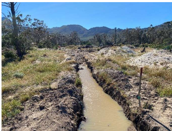
Installation of bulk services along the northwestern corner of the development footprint seen to the east.
