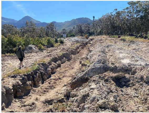
Trench excavations along the southern portion of the site where bulk services are being installed.
