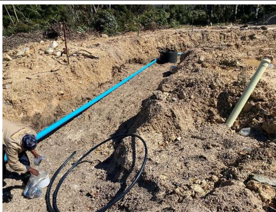
Installation of potable water pipelines near the contractors camp.
