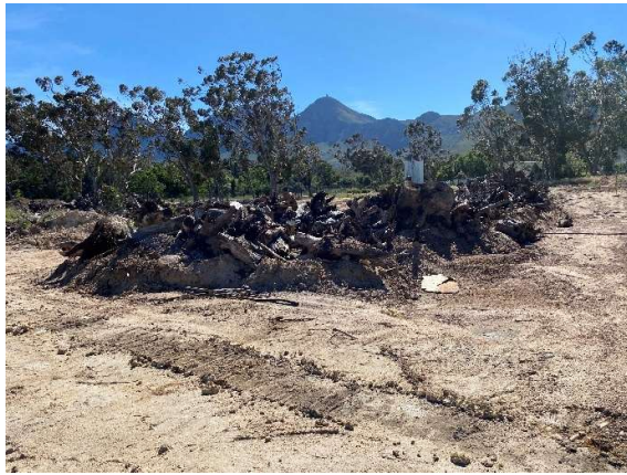
Cleared Blue Gum trees and roots, temporarily stockpiled along with topsoil towards the east of the site.
