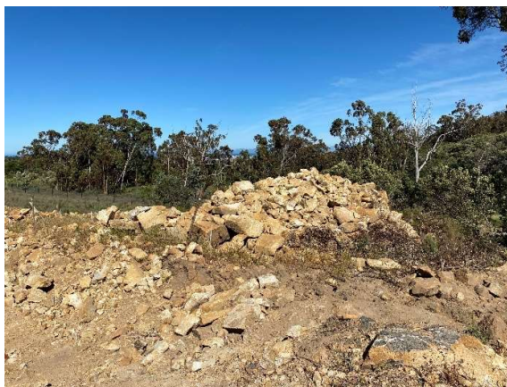
Rocky outcrop area with additional excavated rocks stockpiled just northeast of the attenuation area.
