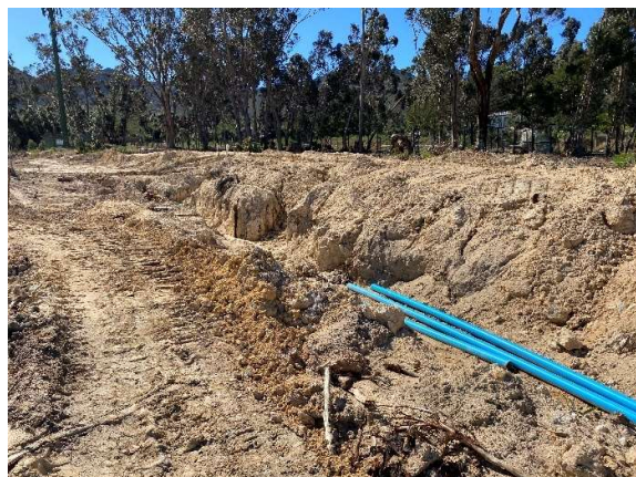
Installation of sewer, and potable water services as seen towards the east.
