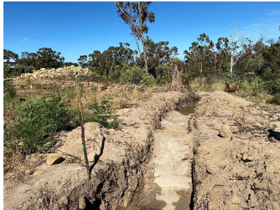
Installation of bulk services along the northwestern corner of the development footprint seen to the west.
