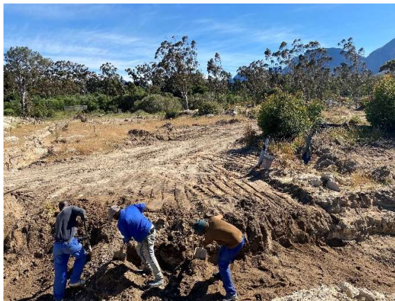
Installation of sewer pipelines along the southern portion of the site.
