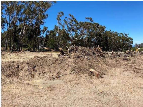
Cleared vegetation and stockpiled topsoil towards the east of the site.
