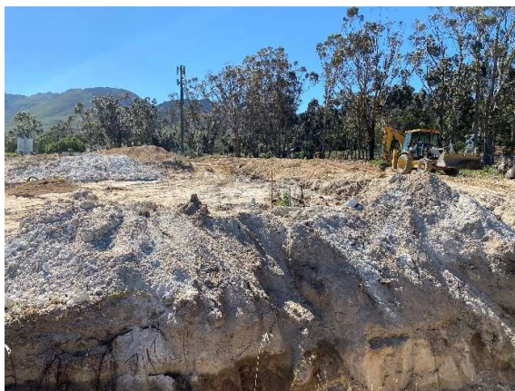
Excavations along the southeastern portion of the site showing the subsoil layers.
