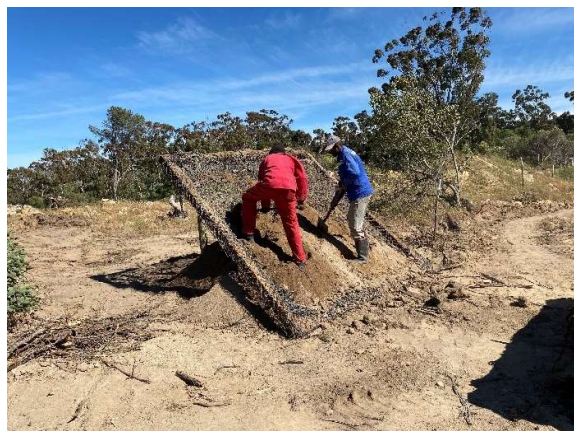
Contractors sieving excavated soil materials by size using a sieve.
