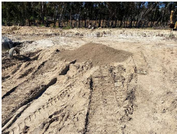
Sand and sieving area towards the centre of the site near the stockpile area.
