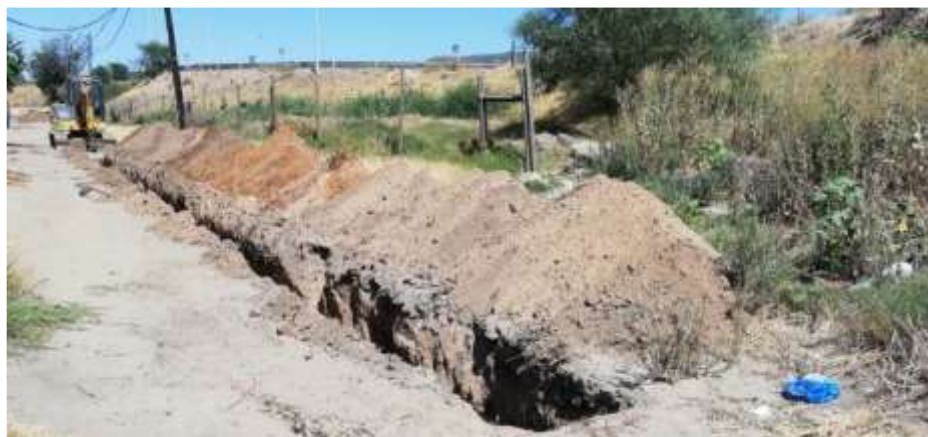
Figure F: Excavation for pipe trenching with stockpiles alongside.
