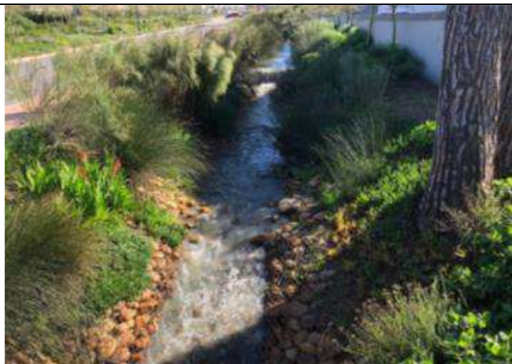
Figure B: Examples of open swales, considered to be SuDs utilised as part of residential developments for conveyance of stormwater
