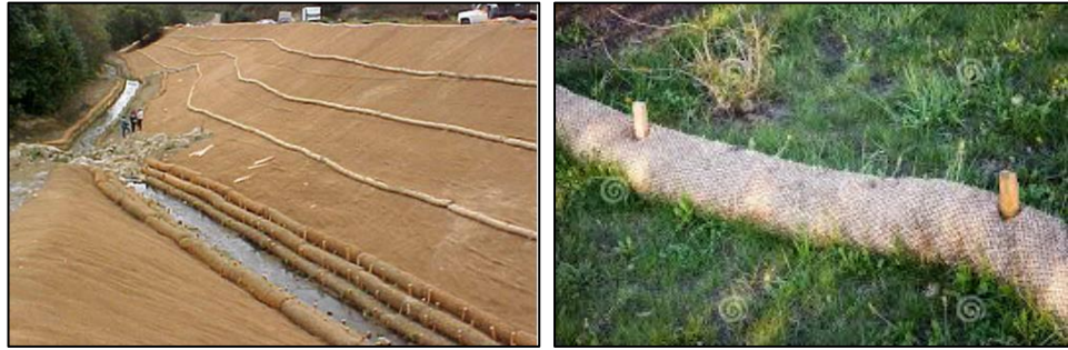
Figure 32: Examples of Coir logs for hydroseeding along embankments.
