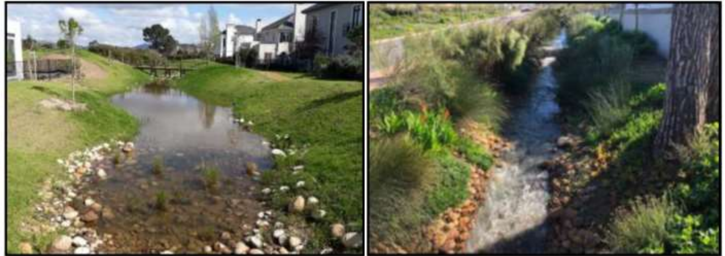
Figure B: Examples of open swales, considered to be SuDs utilised as part of residential developments for conveyance of stormwater
