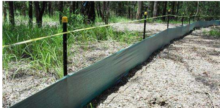
Figure A: (Left) example of temporary safety fencing used to demarcate a watercourse
