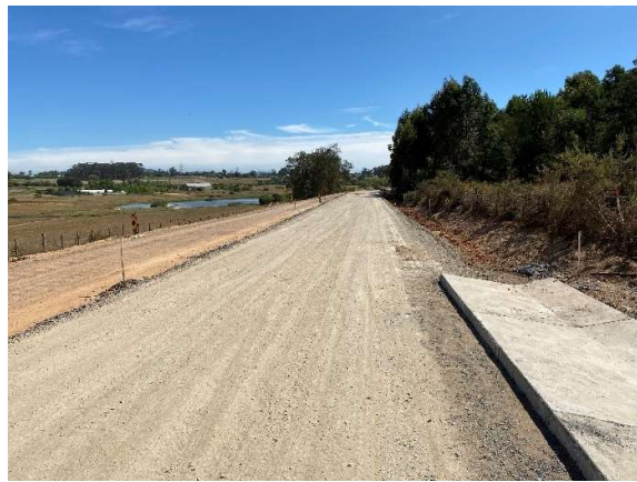
Stormwater side drains being installed.
