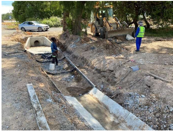
Stormwater side drains being installed.
