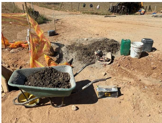
Cement mixing and handling adjacent the stormwater culvert.
