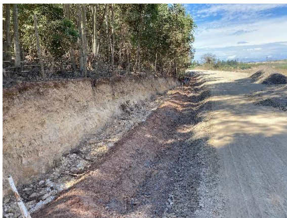
Completed cuttings along the Protea Road as seen towards the east.
