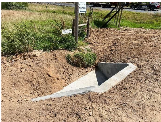
Newly upgraded stormwater culvert.
