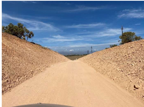
The cutting and shaping of Protea Road towards the east of the contract as seen towards the east.
