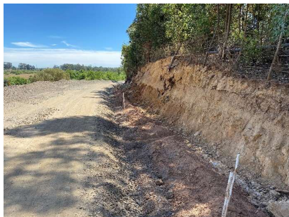
Completed cuttings along the Protea Road as seen towards the east.
