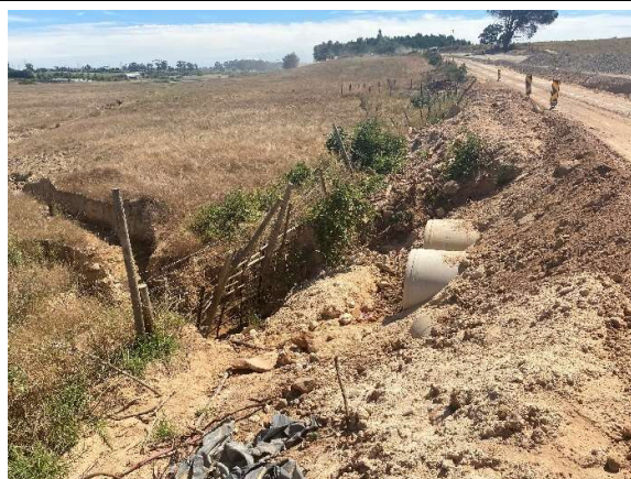
Upgraded stormwater pipelines outlet.
