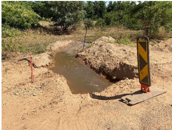
Newly installed stormwater pipeline outlet.
