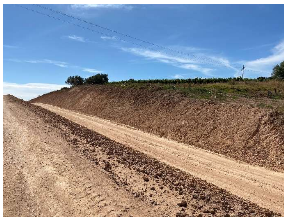
The cutting of Protea Road as seen towards the west.
