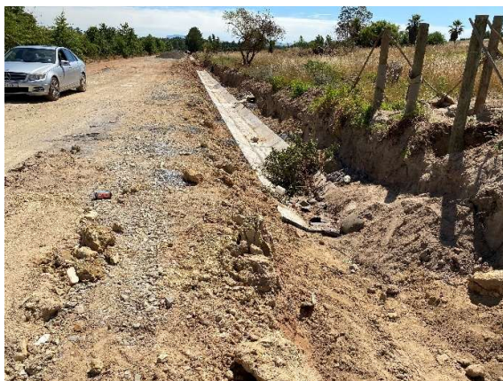
Stormwater side drains being installed.
