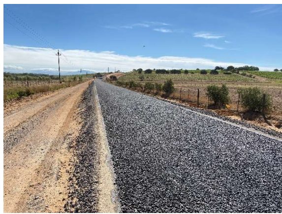
One lane traffic currently open along the completed road surface.
