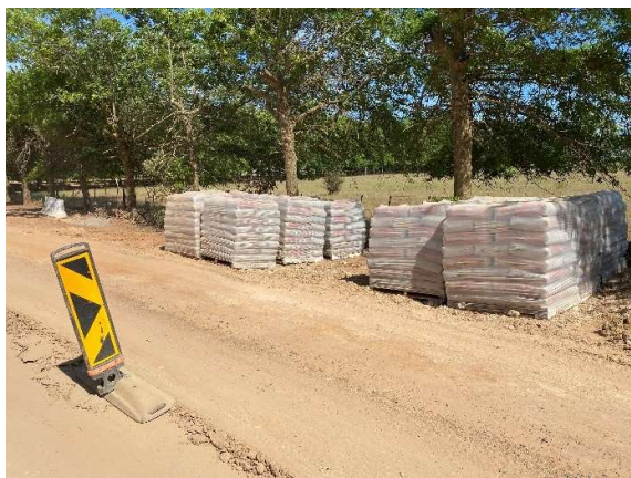
Curbmix cement pallets offloaded near the the Joostenberg Primary School.
