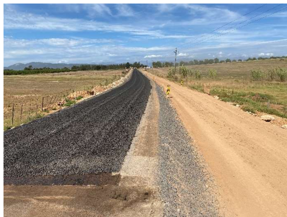
Partially completed road surface along the eastern end at the start of the contract.
