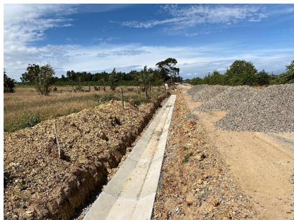
Stormwater side drains being installed.
