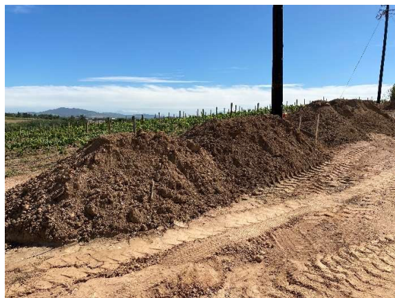
Windrowed topsoil adjacent the newly cleared section of Protea Road.
