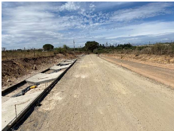
Stormwater side drains being installed.
