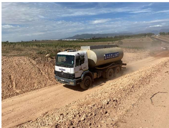
Water tanker for dust suppression along the route.
