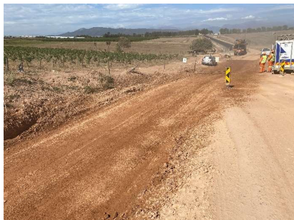
Road treated with water for dust suppression.
