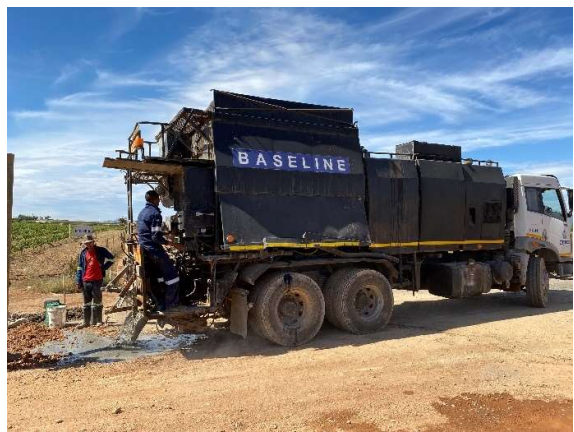
Premix cement adjacent the stormwater culvert.
