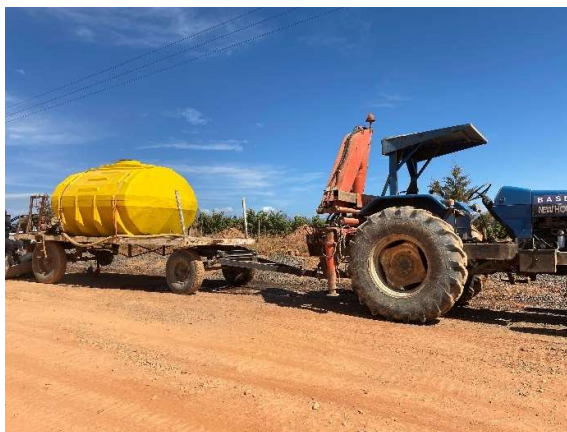
A tractor and water cart along the route for dust mitigation.
