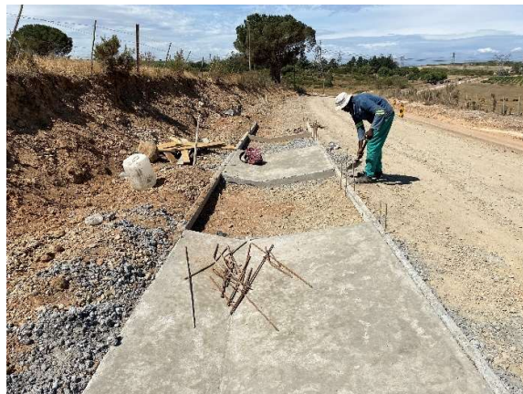
Stormwater side drains being installed.
