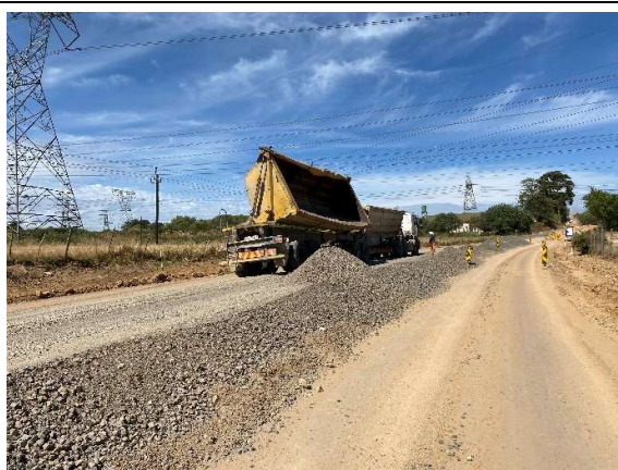
Material for road preparation being offloaded.
