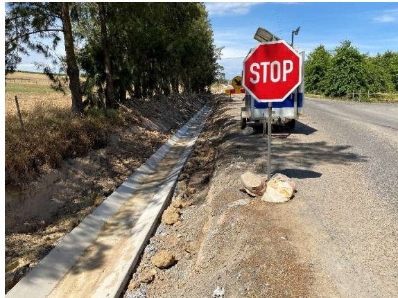
Stormwater side drains being installed.
