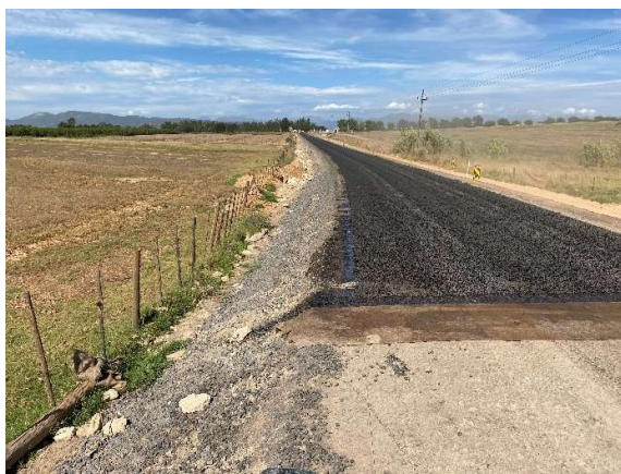
Partially completed road surface along the eastern end at the start of the contract.
