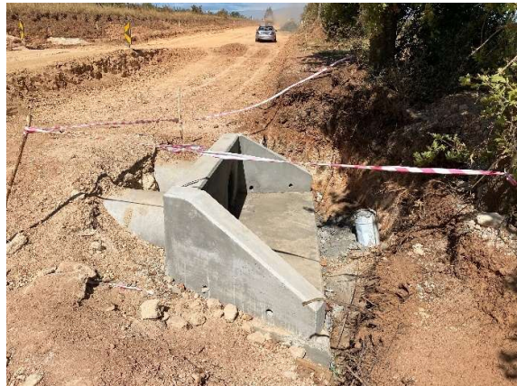
Upgraded stormwater pipeline outlets with new wingwalks at the outlet.
