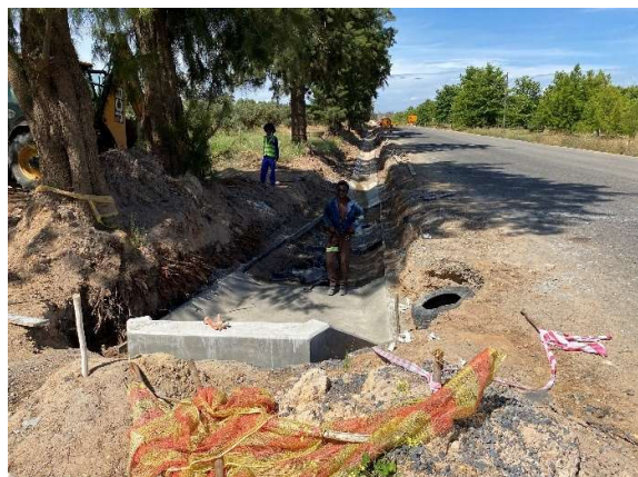
Stormwater side drains being installed.
