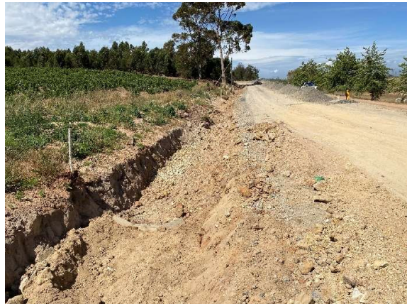
Excavations underway for the installation of side drains.
