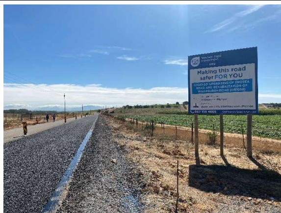
Notice board at the intersection of Hercules Pilaar Road and Protea Road at the start of the contract.
