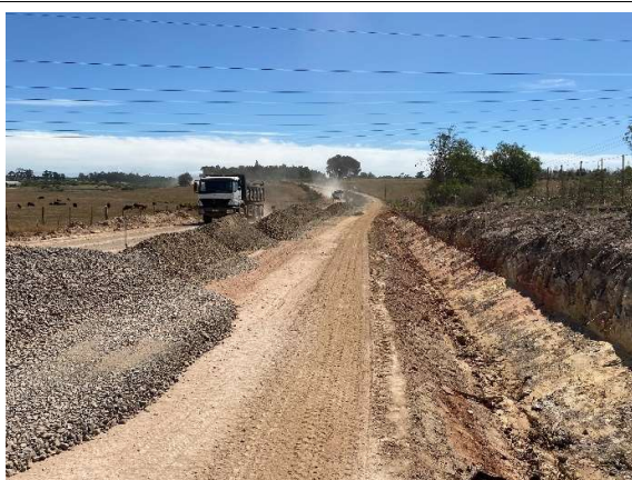
Excavated side drain channels and trucks delivering aggregate as seen towards the west.
