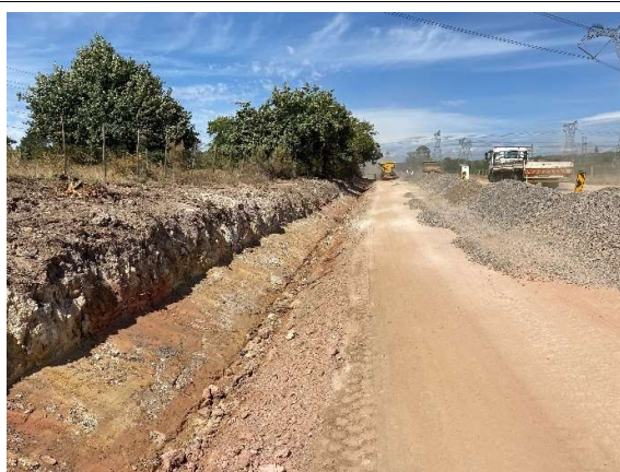
Excavated side drain channels and trucks delivering aggregate as seen towards the east.
