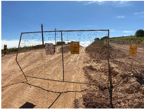
Notice of excavations and construction in progress.
