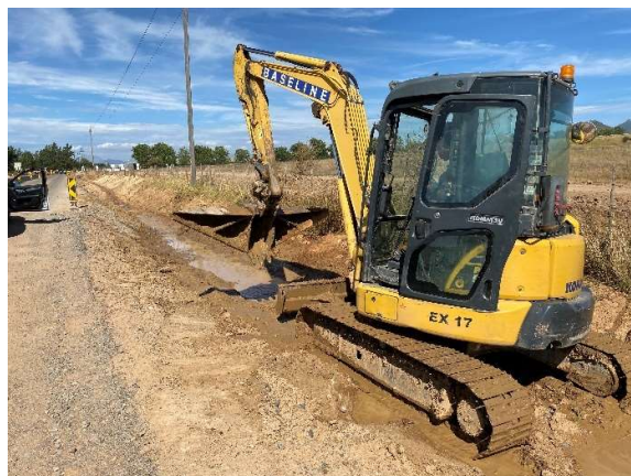
Excavating side drain channels.
