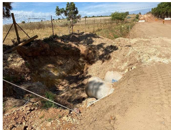
Upgraded stormwater pipeline inlets near the the Joostenberg Primary School.
