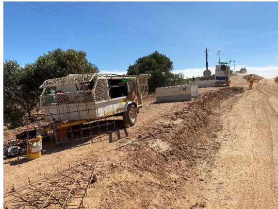
Traffic control station along the construction route.
