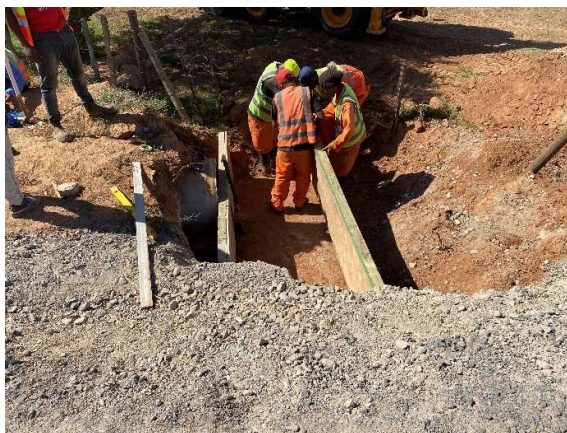
Stormwater pipeline being reconstructed.
