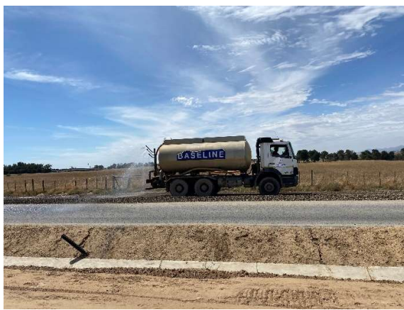
Water tanker for dust suppression along the route.
