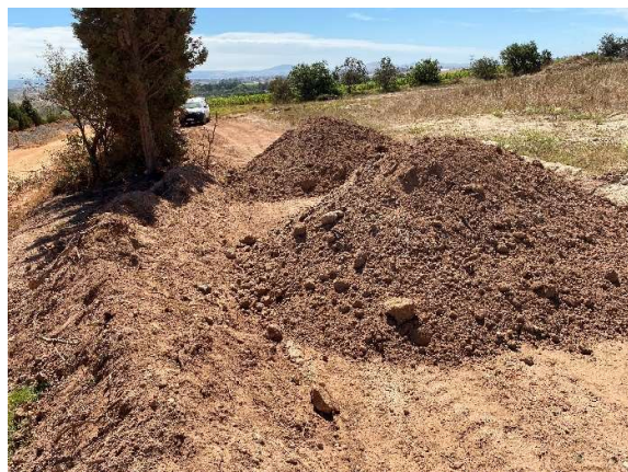
Windrowed topsoil on top of the road shoulder.
