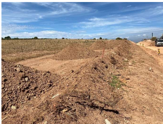
Windrowed topsoil on top of the road shoulder.
