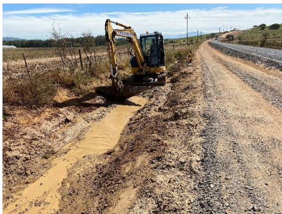
Excavating side drain channels.
