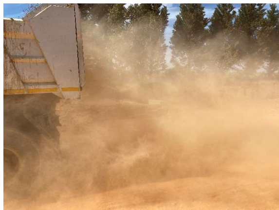
Dust generation from the truck movement.
