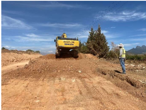
Shaping of the road and embankments underway.
