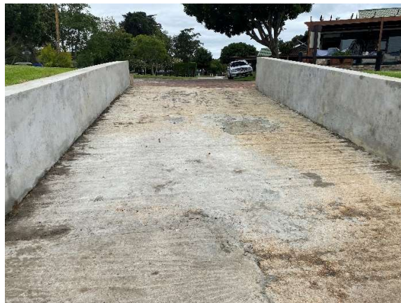
Condition of the slipway.
