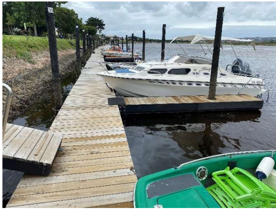
Completed jetty showing the gang-plank, jetty and fingers as seen towards the south.
