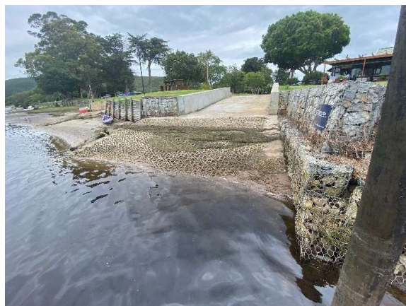
Condition of the slipway.
