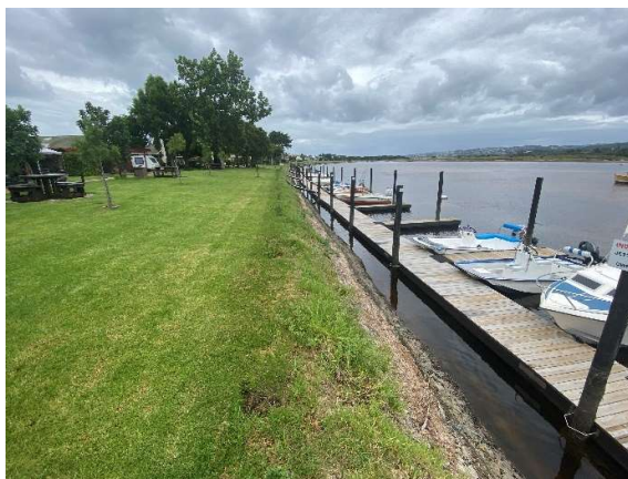
Rehabilitation of the riverbank.
