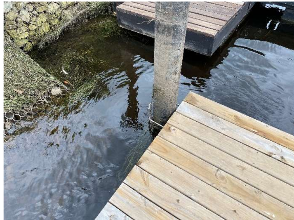
The southern end of the San Marino jetty and the northern end of the Blue Waters River Estate jetty.
