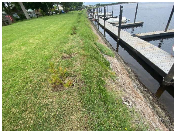
Rehabilitation of the riverbank.
