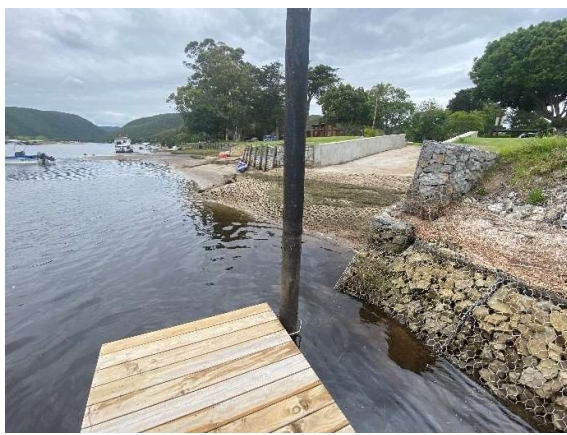
The northern end of the jetty showing the completed layers of the .
