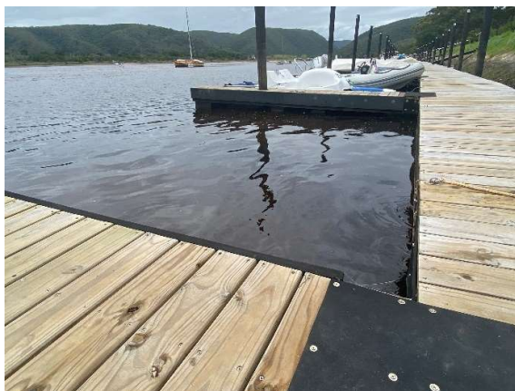
Attached floating jetty and mooring fingers with the 5m gap as seen towards the north.
