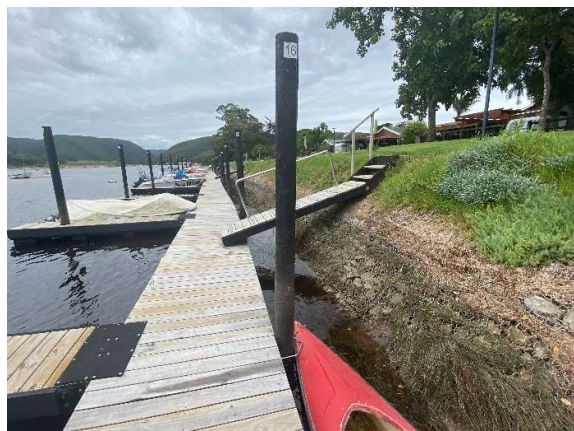
Condition of the jetty showing the gang-planks on low tide as seen towards the north.
