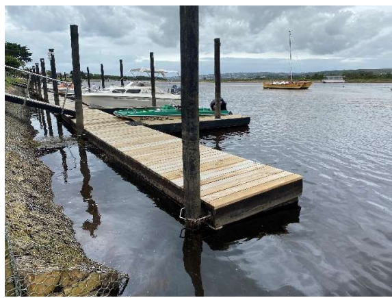
Weinstalled mooring poles.
