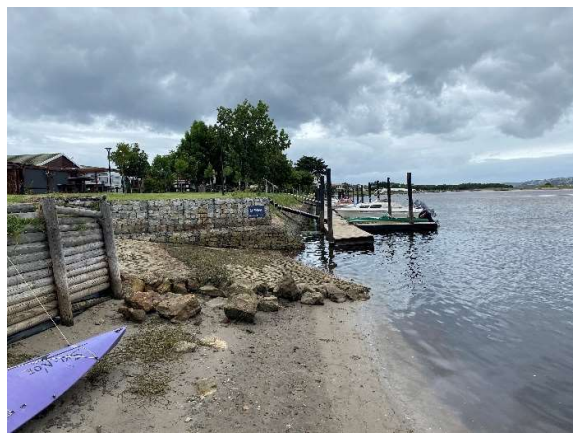
Bottom of the slipway during low tide as seen towards the south.
