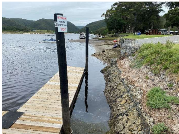
Successfully installed mooring poles.
