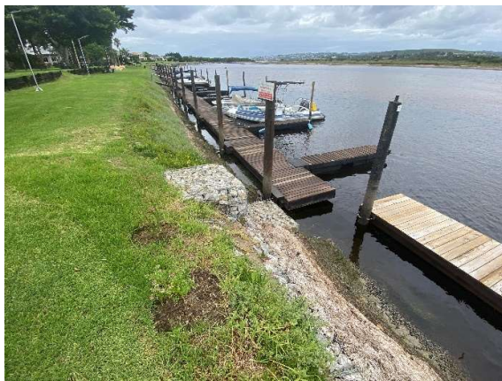
Tie-in point with Blue Waters.
