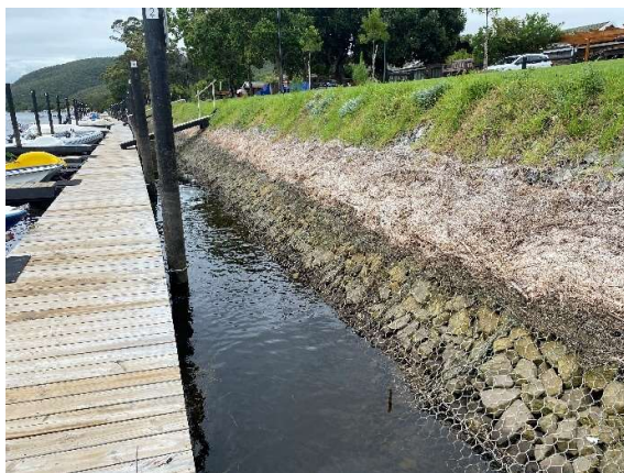
Condition of the jetty and the reno-matresses on low tide as seen towards the north.
