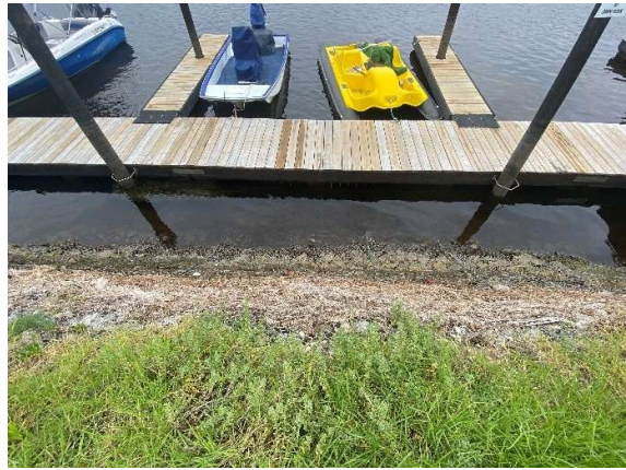
Rehabilitation of the riverbank.
