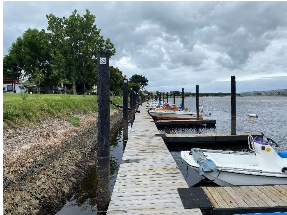
Successfully completed and operational jetty as seen towards the south.
