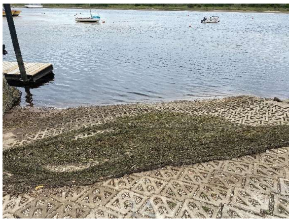
Vegetation debris at the bottom of the slipway.
