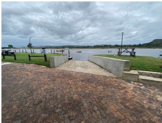
Condition of the slipway from the road-side.
