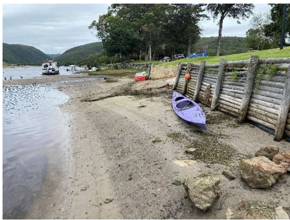
Bottom of the slipway during low tide as seen towards the north.
