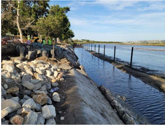
Geotextile over the sandbags followed by reno-mattress (17 July 2023)
