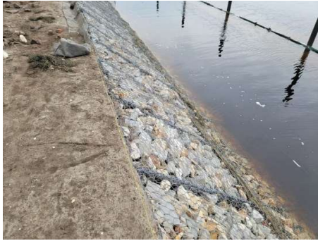
Completion of the installation of the reno-mattress layer (28 July 2023) – prior to adding the growing medium
