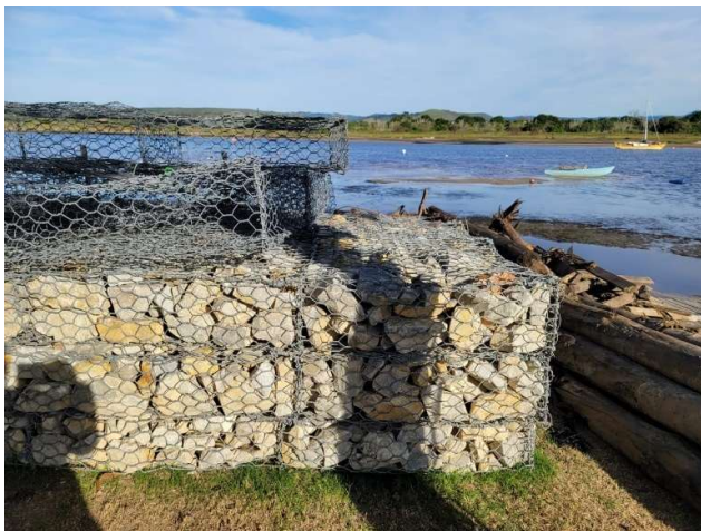
Preparation of the reno-mattress (14 July 2023)
