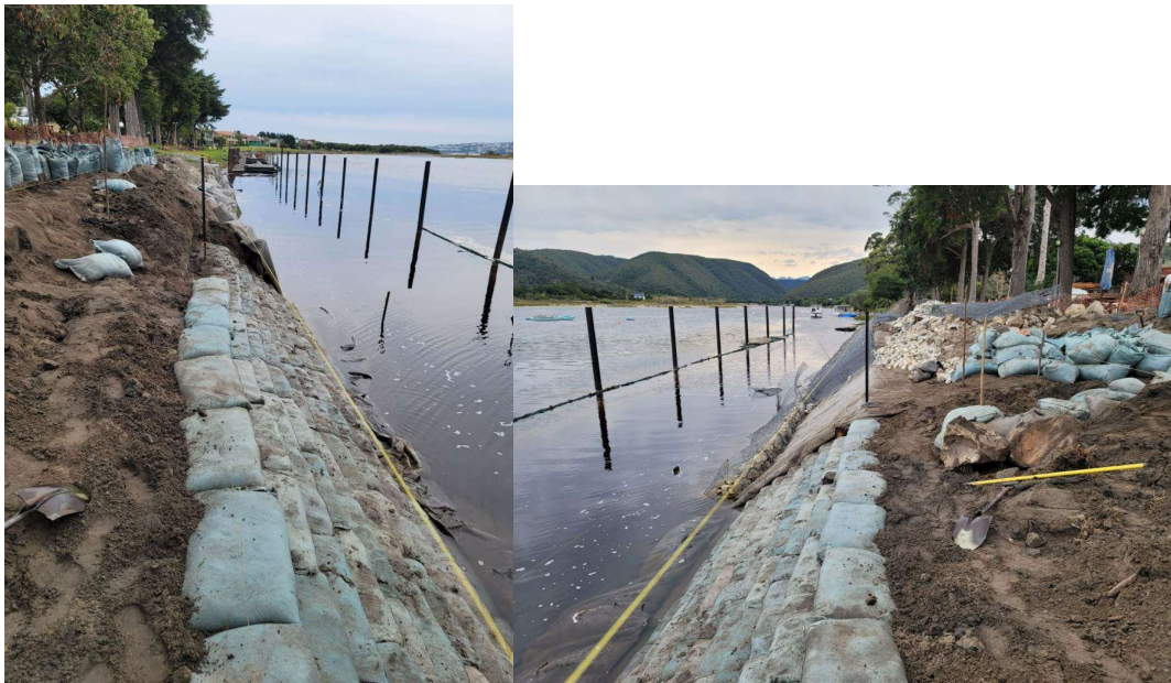
Photographs showing the distinctive layers and progression of shaping, placing sandbags, geotextile followed by the last layer of reno-mattress (28 July 2023)
