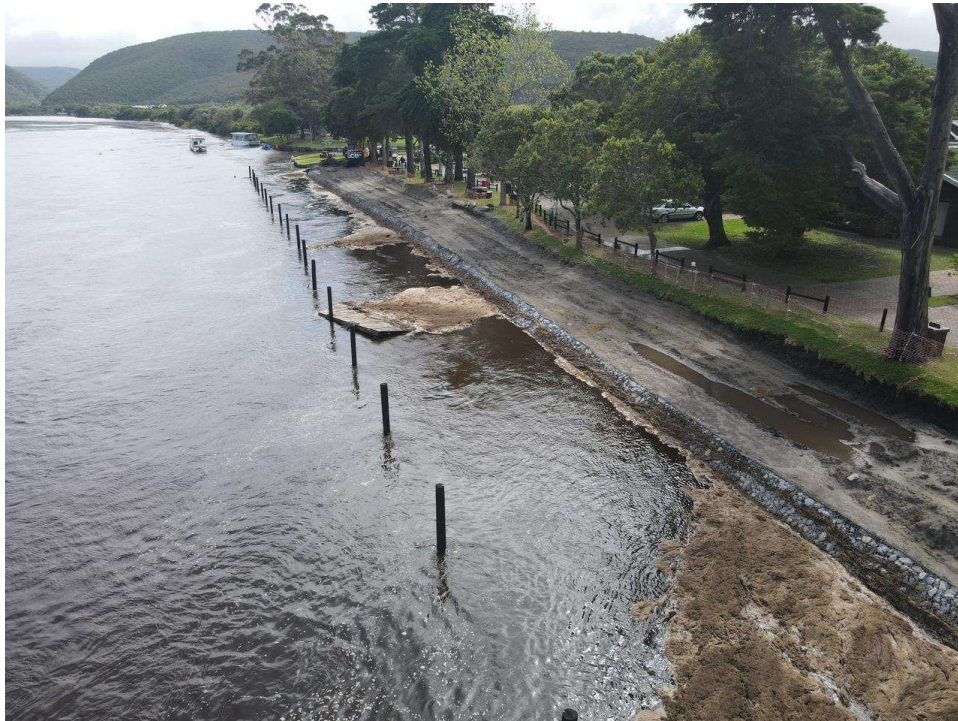
Drone footage following storm surge
