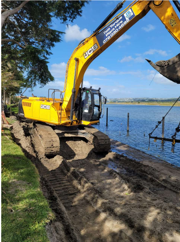
Tie-in with Blue Waters in progress - Photograph taken 20 September 2023
