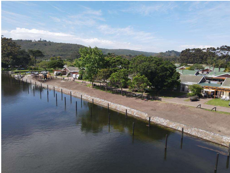
Drone footage following storm surge
