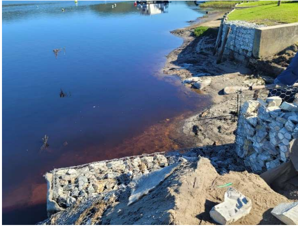
Termination in progress
