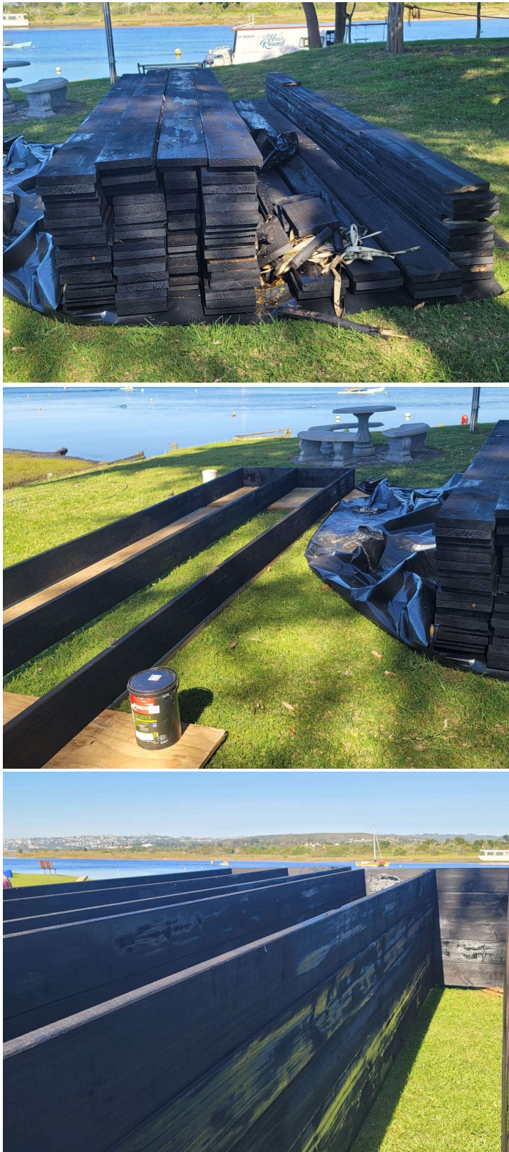
Jetties being assembled on the bank/lawn
