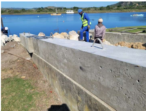
Repair of slipway in progress
