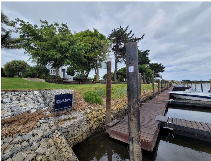
Tie-in with Blue Waters (Photograph taken 28 November 2023)
