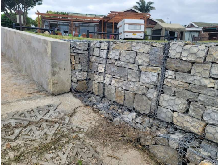
SANRAL spillway completed (photographs taken 28 November 2023)
