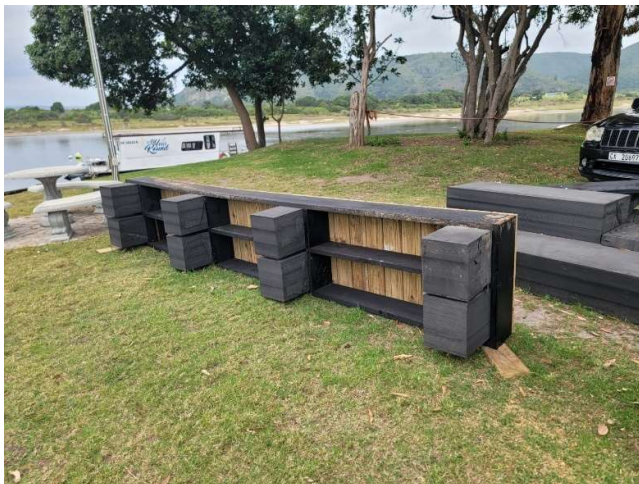
Installation of fingers in process
