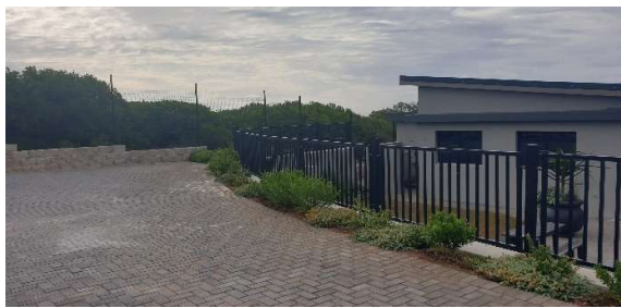
Condition of landscaping inside the premises.
