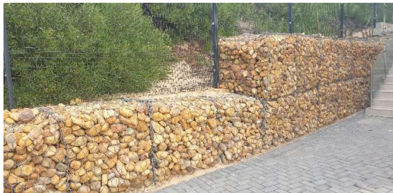
Gabion retention wall towards the south end of the property.
