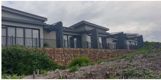
Condition of the single residence towards the north.
