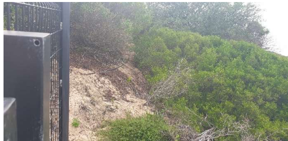
Stormwater outlet on the northern section of the property.
