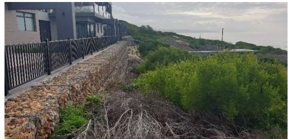
Condition of the gabion retention wall on the eastern boundary of the property.
