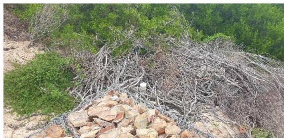
Stormwater installation towards the east of the site.
