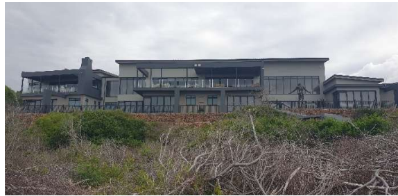
Condition of the single residence towards the west.
