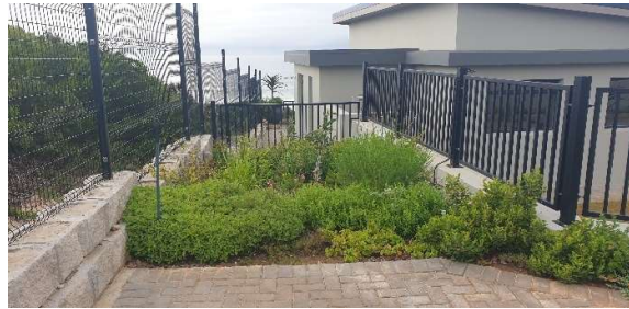
Condition of landscaping inside the premises.
