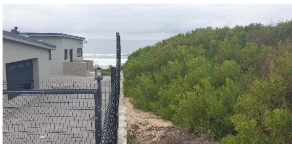
The southern boundary of the property, where one of the sewage conservancy tanks is located.
