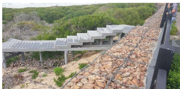
Broadwalk towards the south east.
