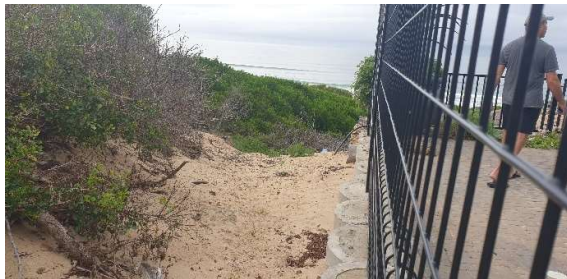
Condition of the natural vegetation corridor towards the north of the site where the stormwater outlet is located.
