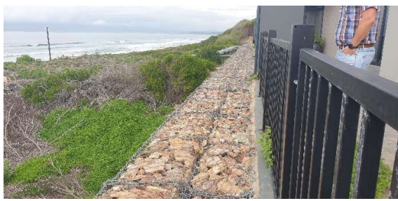
Gabion retention wall on the eastern property boundary.
