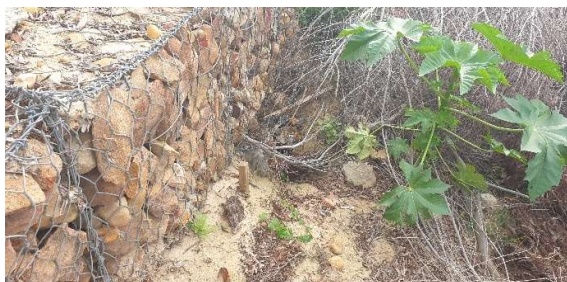
Surveyor peg still in place.
