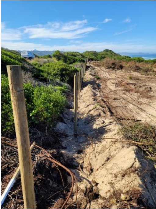
2023.05.10 – Demarcation of the disturbance footprint is clearly indicated, and no-go areas are visible.
