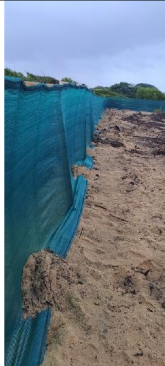
2023.05.12 – Shade netting doubles as a silt fence, ensuring that soil erosion is minimized.
