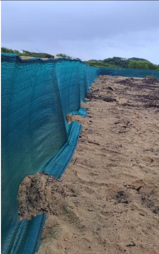
2023.05.12 – the bottom 200mm of the shade netting is buried to act as silt trap.
