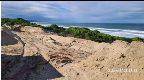
(2023.06.13) – Busy with bulk excavation and earthworks
