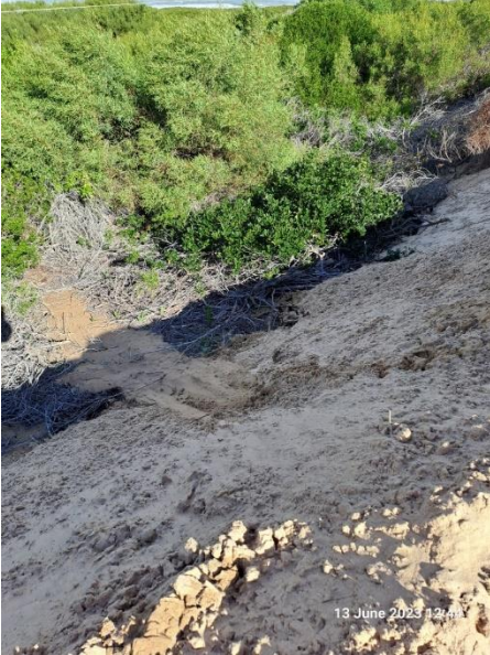
(2023.06.13) – Gabion retainer will be installed to further stop the sand movement
