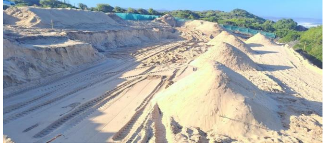
(2023.06.22) – busy with bulk excavation and earthworks.
