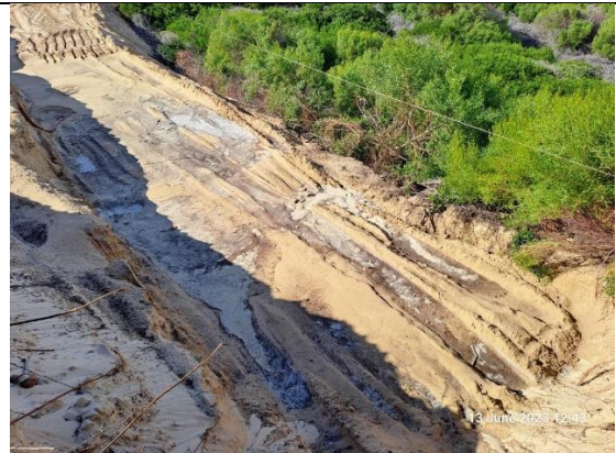
(2023.06.13) – Most southern edge of the property where most earthworks have been completed – gabion retainer will be installed along the southern boundary of the disturbance footprint.
