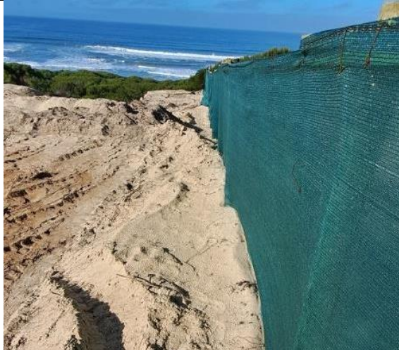
(2023.07.13) The contractor maintains the shade net demarcation.
