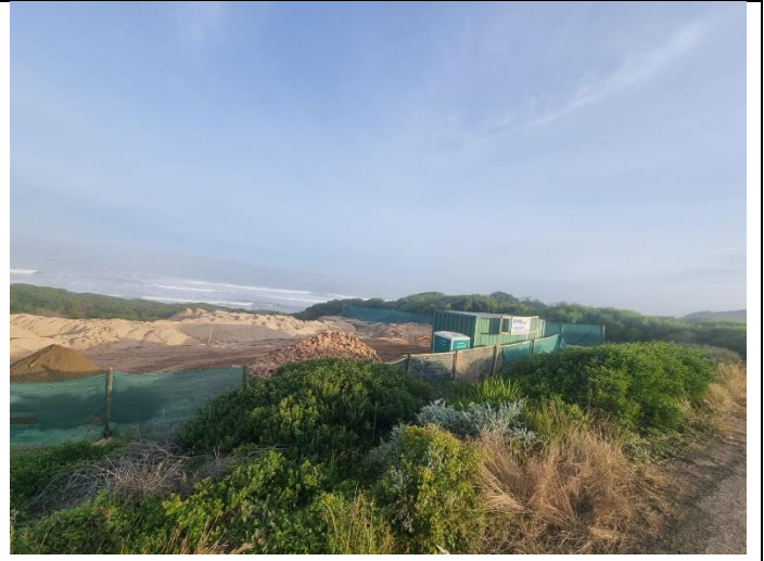
(2023.07.06) gabion stone is moved and stockpiled within the demarcated area.
