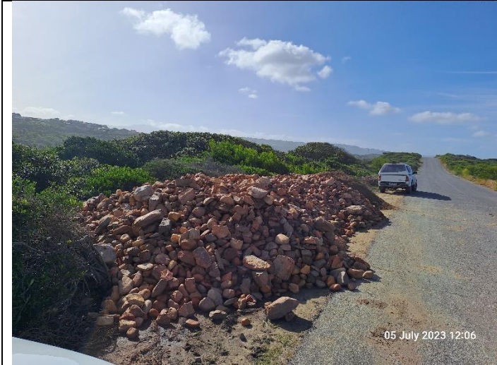
(2023.07.05) Gabion stone is delivered in the road reserve.
