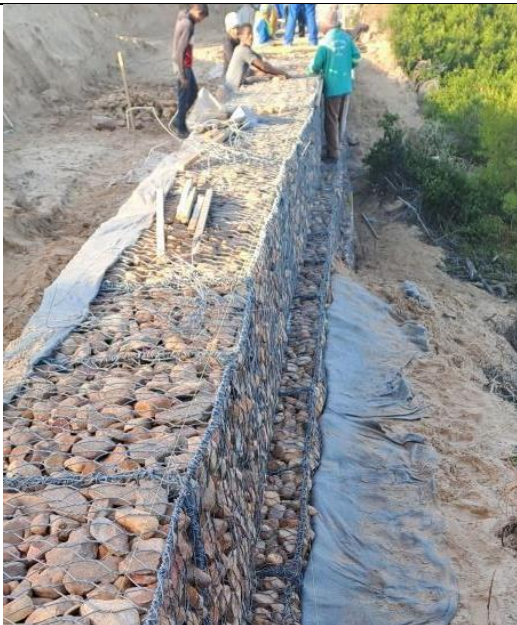
(2023.07.27) – gabion retainer installation progress.
