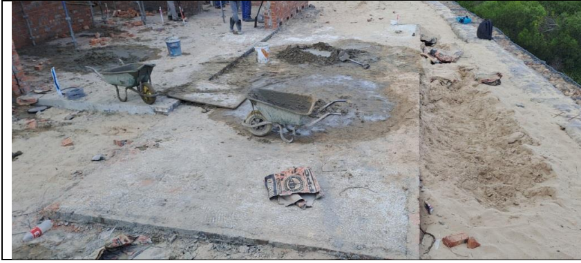
Concrete batching on top of building foundation.
